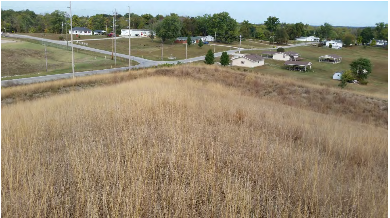
Photo 3: EV2 East Plant Area cover facing northwest
