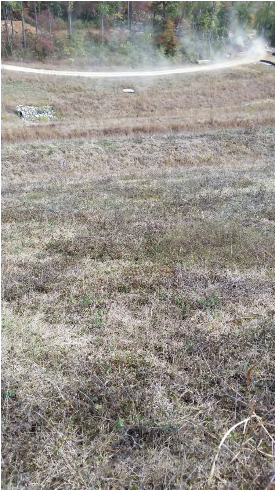
Photo 25: ES8 and ES10 facing north across detention basin 3
