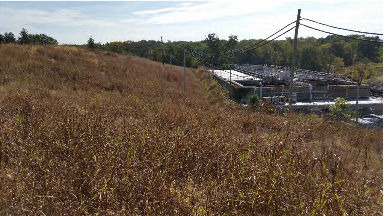
Photo 11: EV6 East Plant Area cover facing southwest
