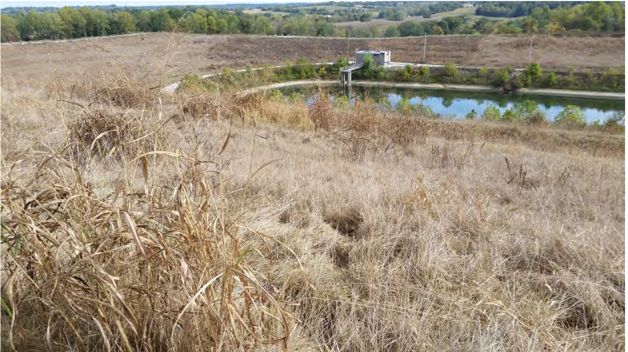
Photo 19: ES2 drainage swale facing north
