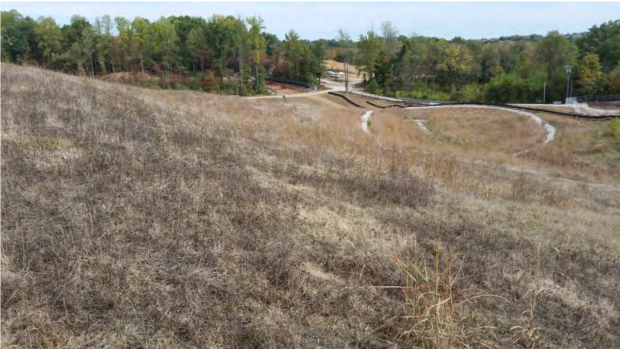
Photo 27: ES11 detention basin #5 facing north
