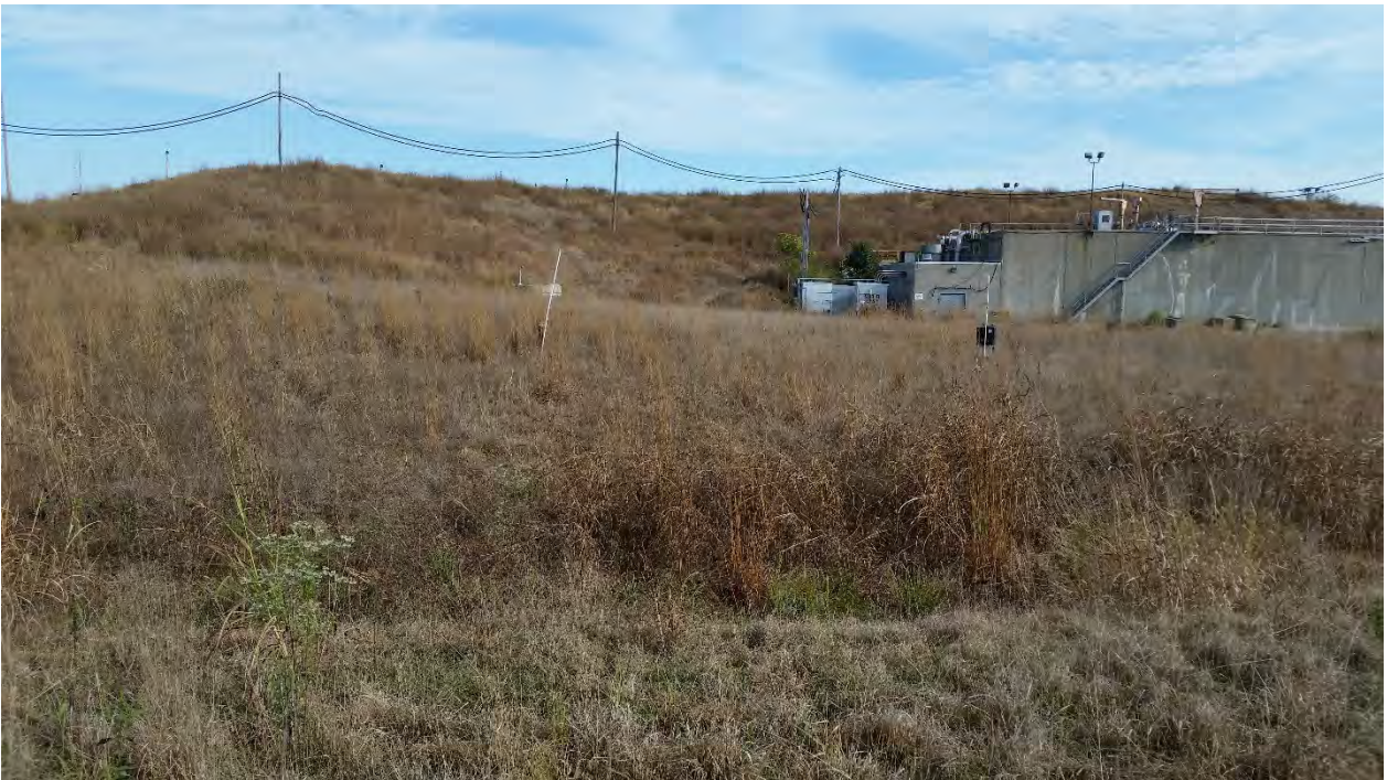
Photo 12: EV7 East Plant Area cover facing north
