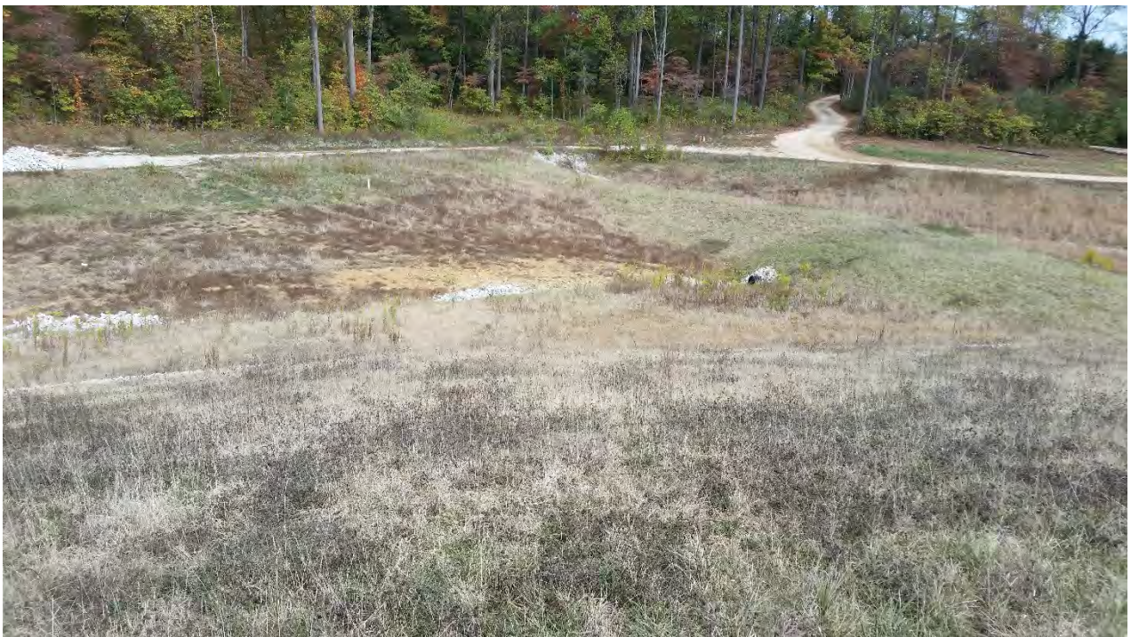
Photo 4: EV3 East Plant Area cover facing north
