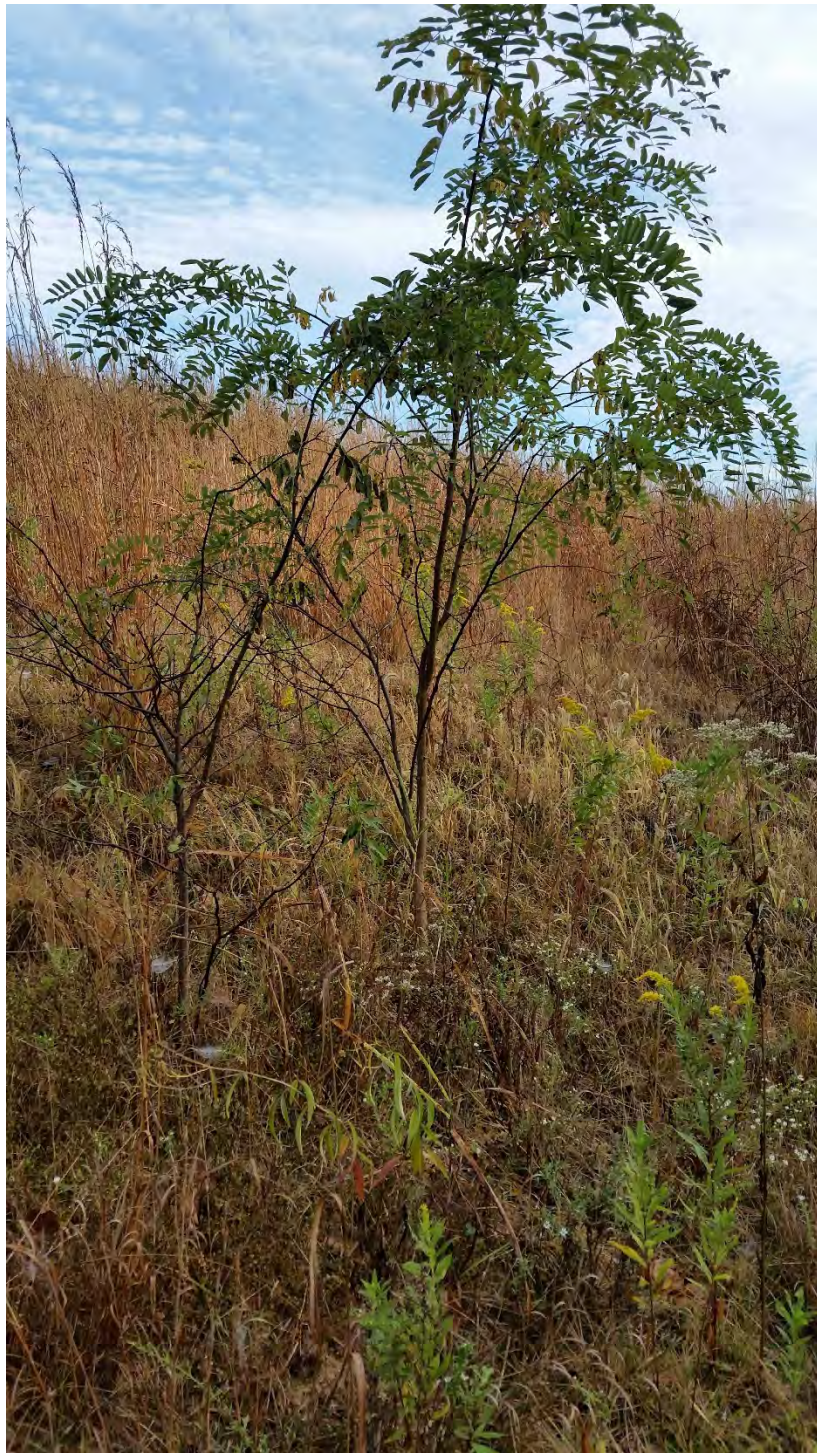
Photo 14: EV9 East Plant Area cover facing south (removed tree growth at time of inspection)
