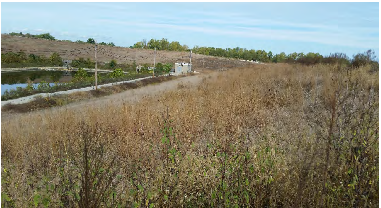
Photo 8: EV5 East Plant Area cover facing northwest
