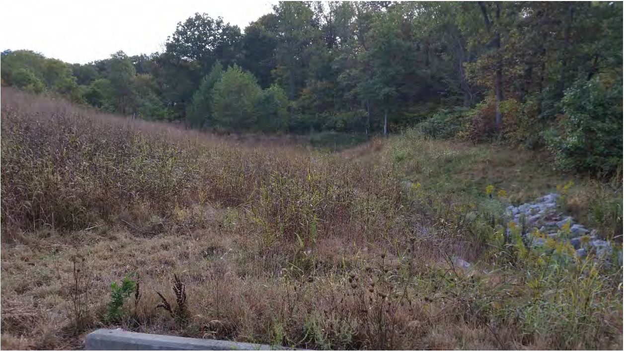
Photo 28: ES13 detention basin 6 facing east
