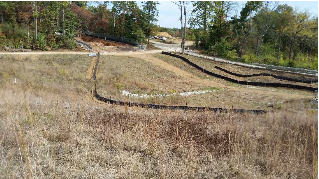
Photo 6: EV4 East Plant Area cover facing northeast across Pilot Trench alignment
