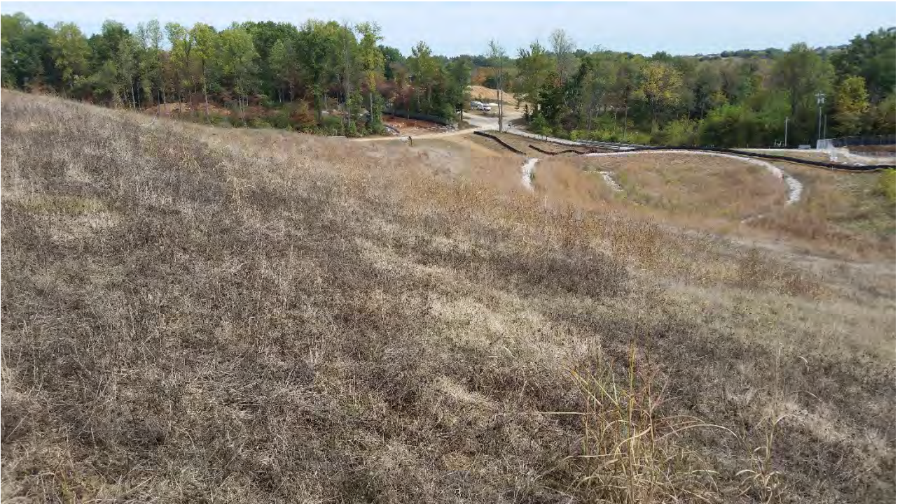
Photo 5: EV4 East Plant Area cover facing northeast
