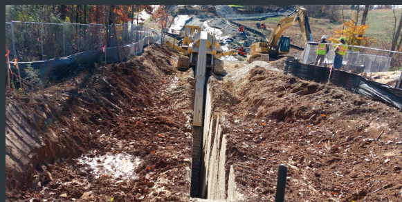
PILOT TRENCH CONSTRUCTION
