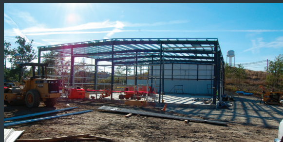
NEW GROUNDWATER TREATMENT PLANT
