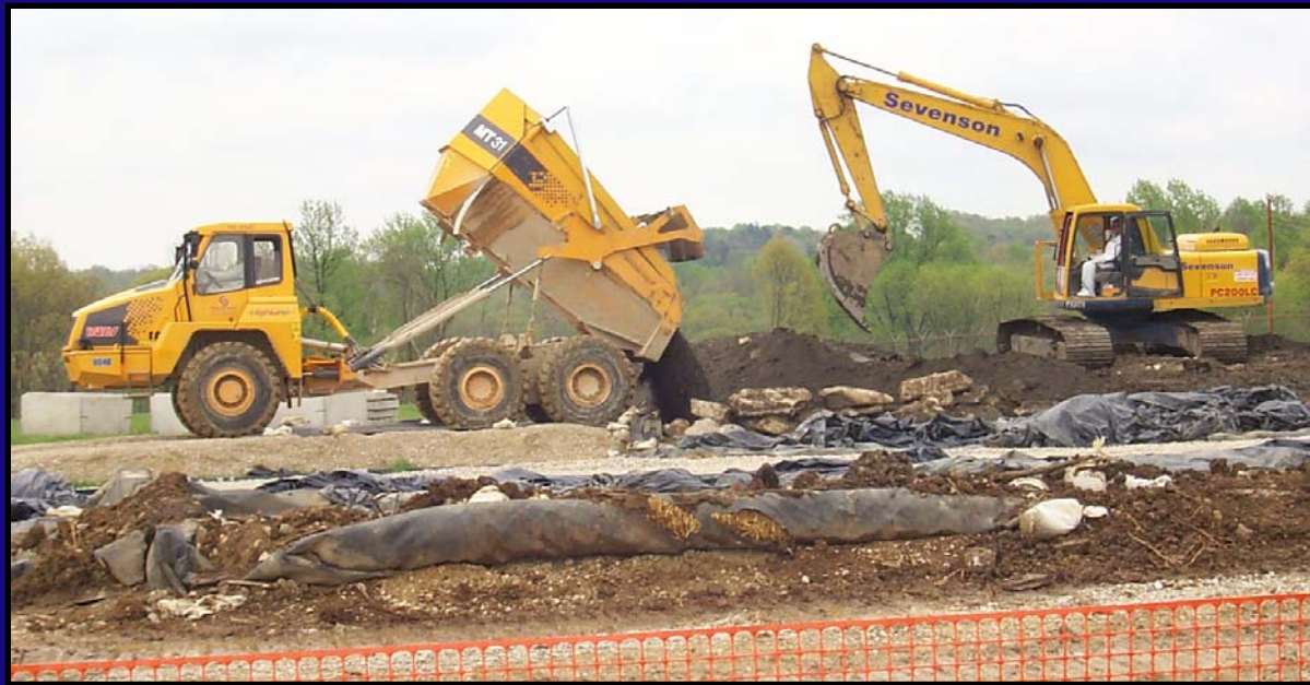
Stockpiling and covering
