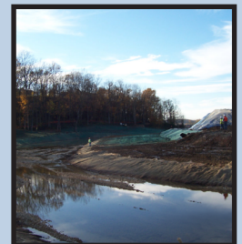
Hydroseeding Diversion Channel 2
