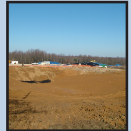
Clay Placement &amp; Compaction
