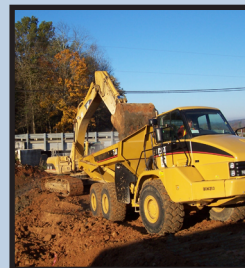
Diversion Channel 2 Bypass
