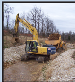
Backfill Placement In Creek Restoration
