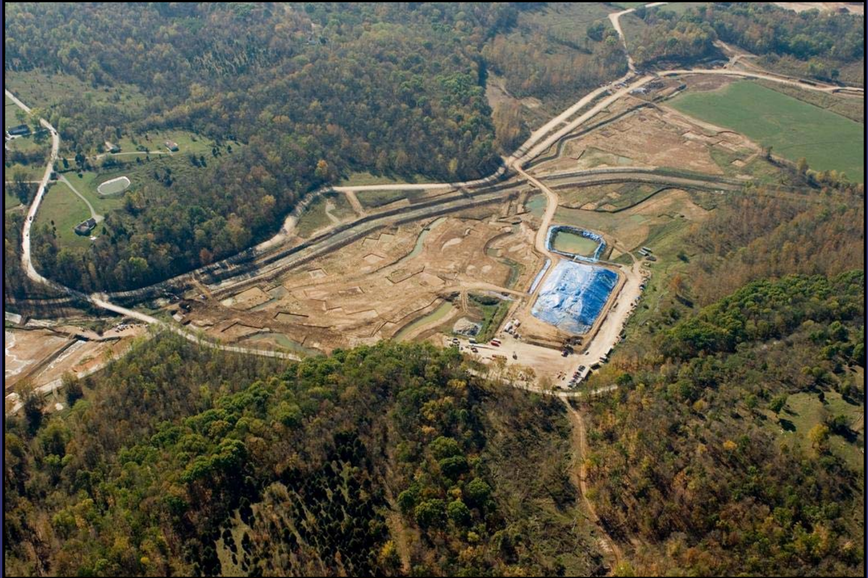
Excavation east of Peerless Road
