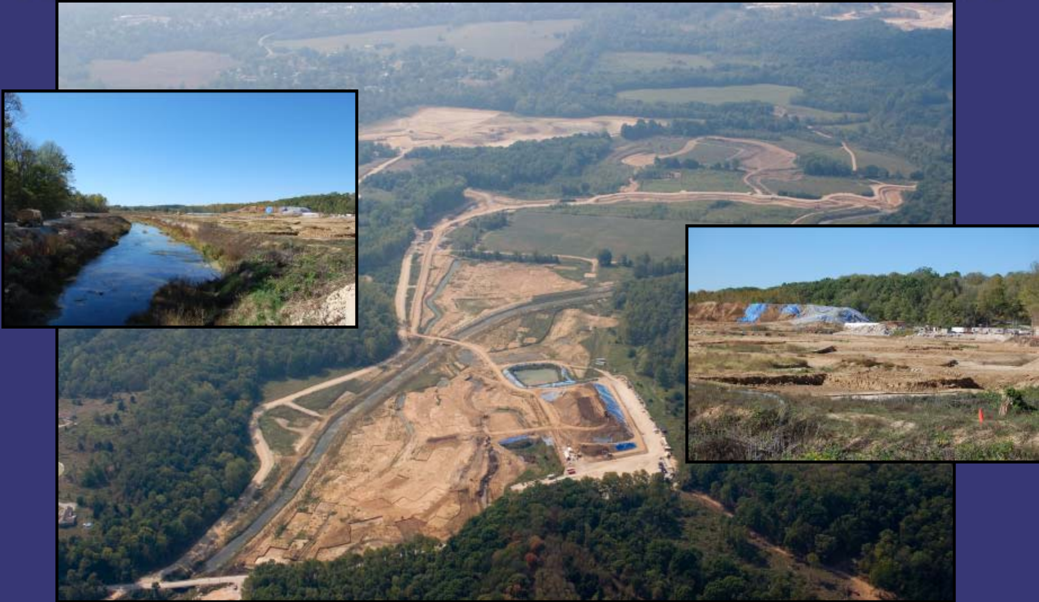
Excavation west of Peerless Road
