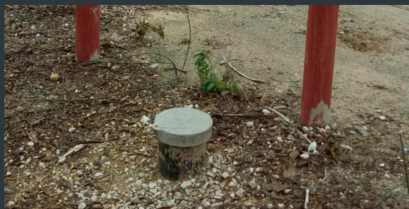
GROUNDWATER WELL INSTALLED
