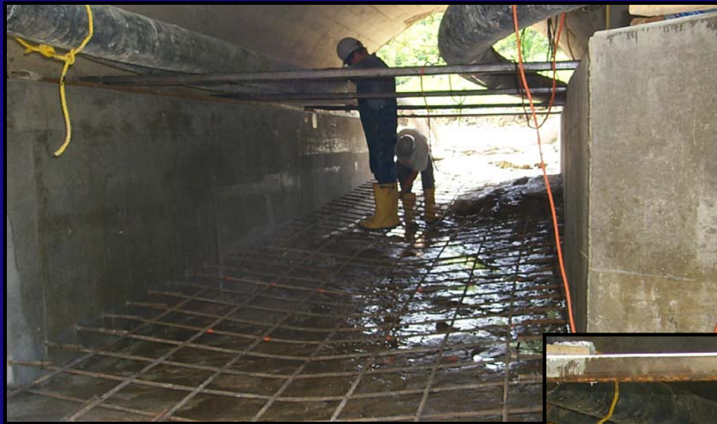
Restoration of culvert under Bailey Scales Road
