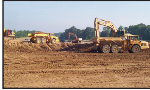
Excavation of Clean Soil at a Local Source
