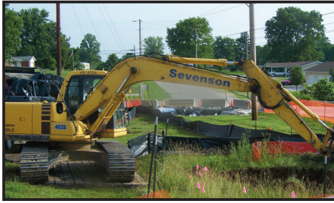
Sewer Abandonment at Breckenridge Rd. and GM Drive
