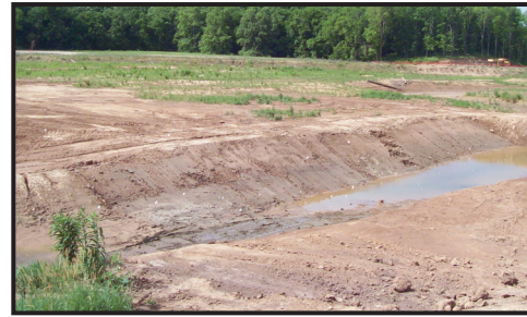
Creek Excavation Downstream of Peerless Rd.
