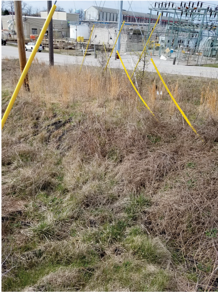
Photo 16: East Plant Area Cover System southeast of EV6.
