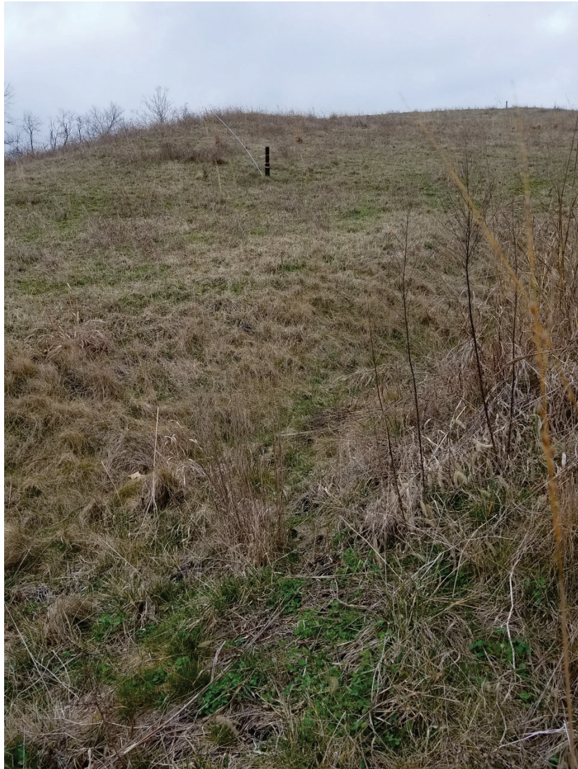
Photo 17: ES14 East Plant Area Cover facing south towards EV9.
