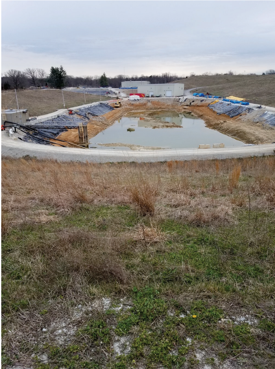
Photo 7: EV3 East Plant Area Cover facing south.
