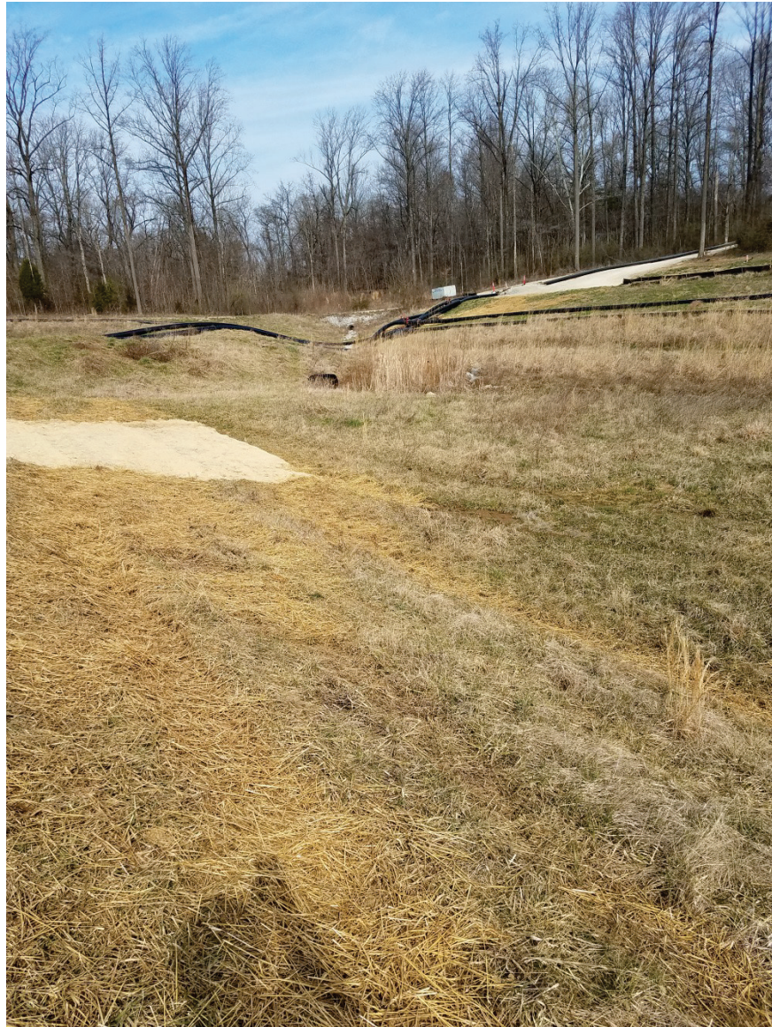
Photo 10: ES9 East Plant Cover System facing west through detention basins.
