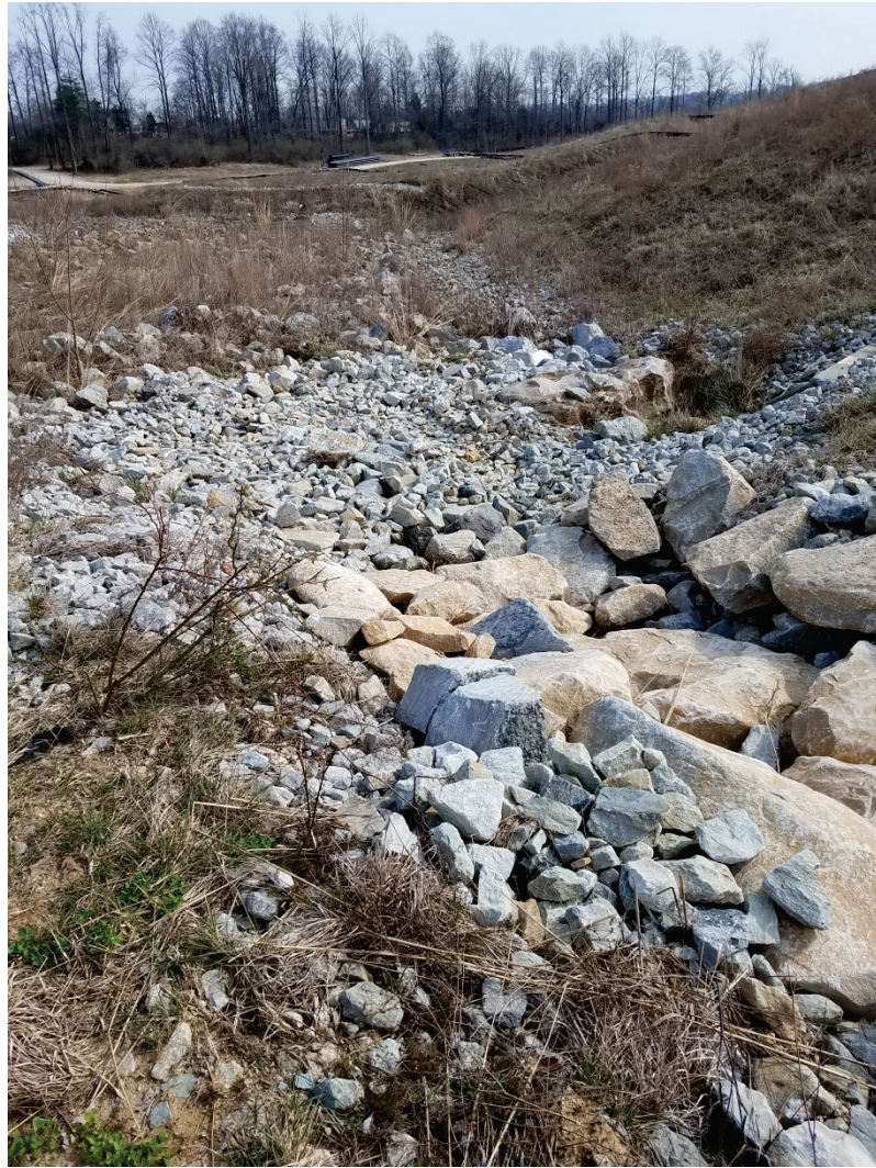
Photo 6: Drainage channel at ES6 East Plant Area Cover facing northeast.
