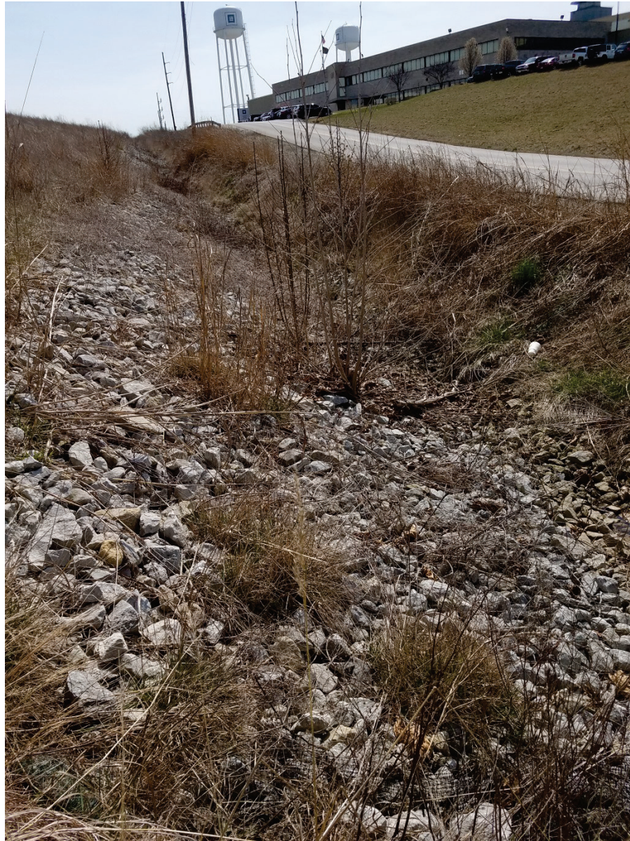
Photo 4: West of ES3 East Plant Area Cover, along GM Drive, facing south.
