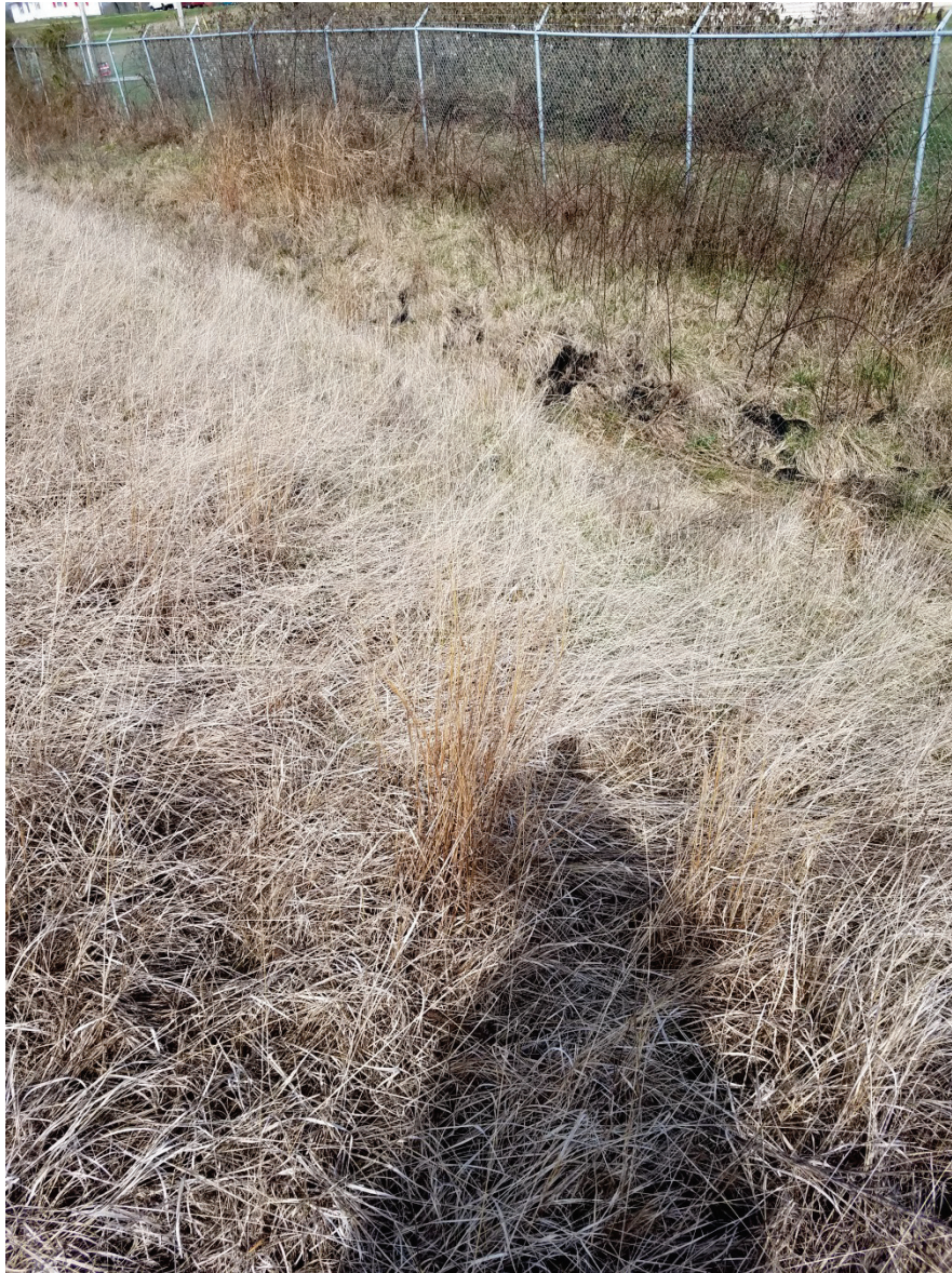
Photo 5: EV2 East Plant Area Cover facing northwest
