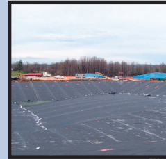
Completed Vault Liner
