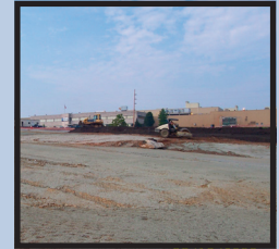
Vault Material Placement
