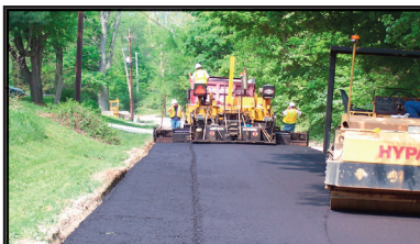
Paving Broomsage Road
