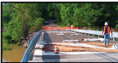
Peerless Road Bridge Construction
