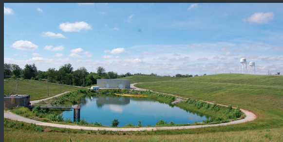
WATER TREATMENT PLANT AND THE STORM WATER POND
