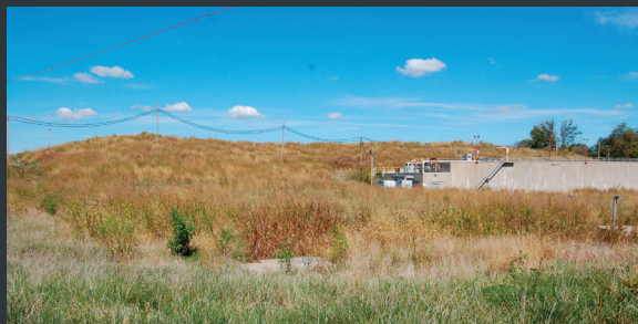
THE COVER SYSTEM FACING NORTH
