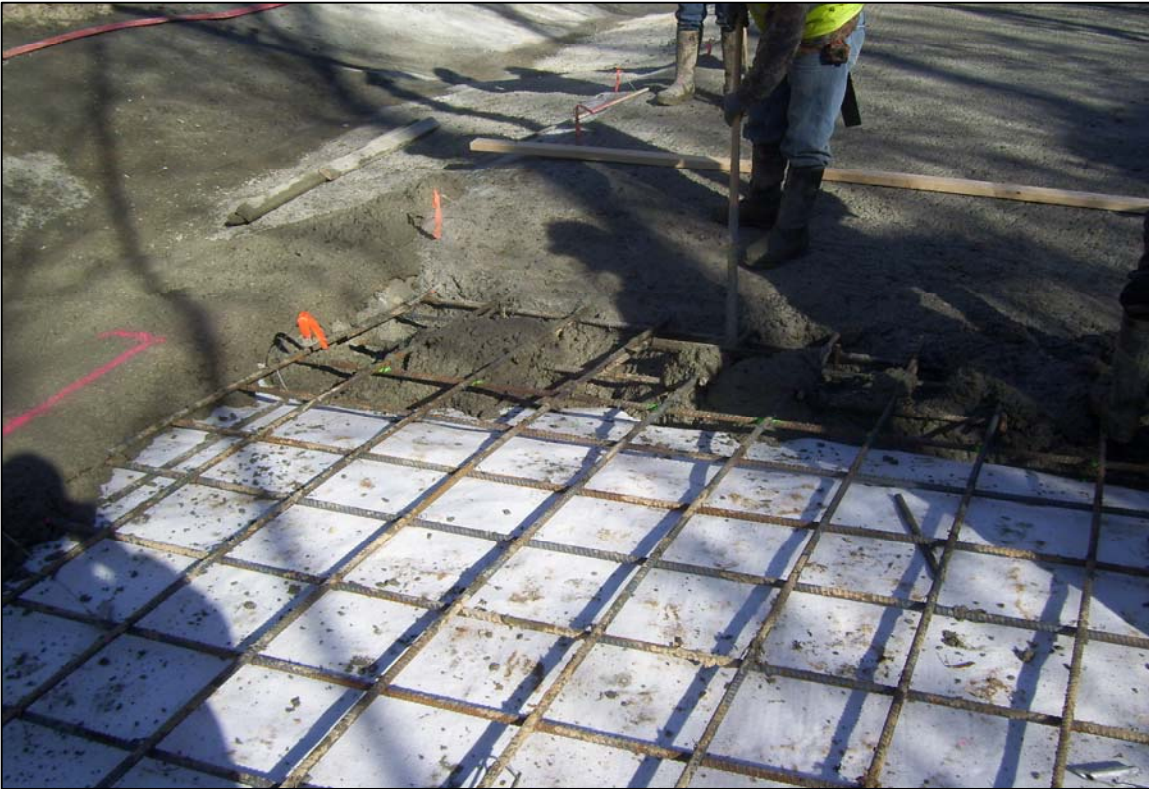
PHOTO No. 32: LAYING OF REBAR MATTING OVER GLC FEB. 2012
