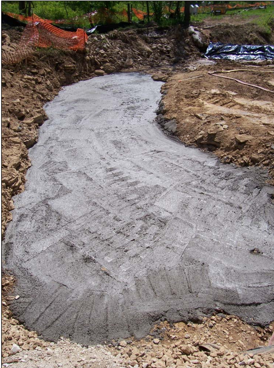
PHOTO No. 11: CONCRETE FILLED IN SWALLET 4. MAY. 2005
