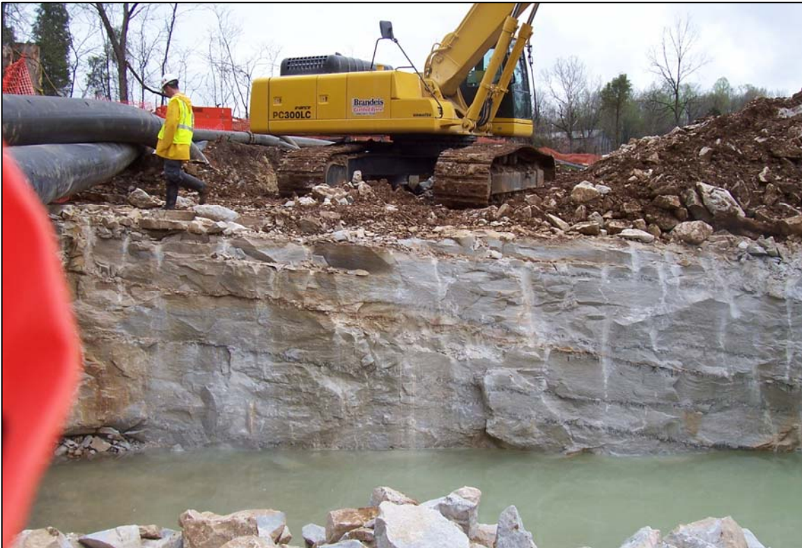
PHOTO No. 8: ROCK FACE OF EXCAVATION ALONG BROKEN OUT FRACTURE NEAR SWALLETS 1A AND 1B. APR. 2005
