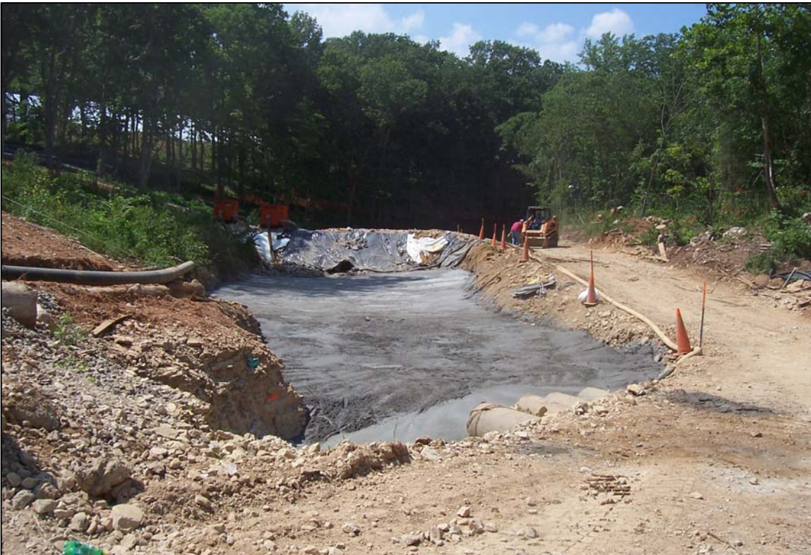
PHOTO No. 14: COMPLETED CONCRETE NEAR SWALLETS 2 AND 3. AUG. 2005
