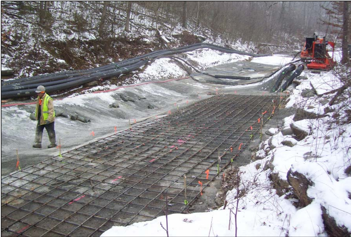
PHOTO No. 34: REBAR MATTING FOR CONCRETE ACCESS ROAD. FEB. 2012
