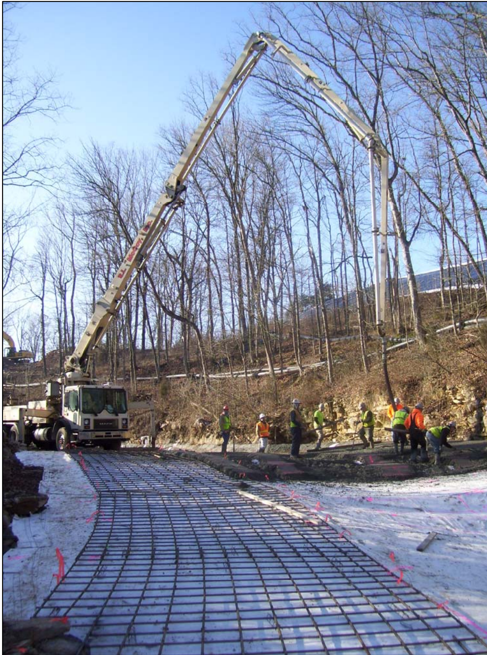
PHOTO No. 31: REBAR MATTING COVERING GLC LAYER FOR CONCRETE POUR FEB. 2012
