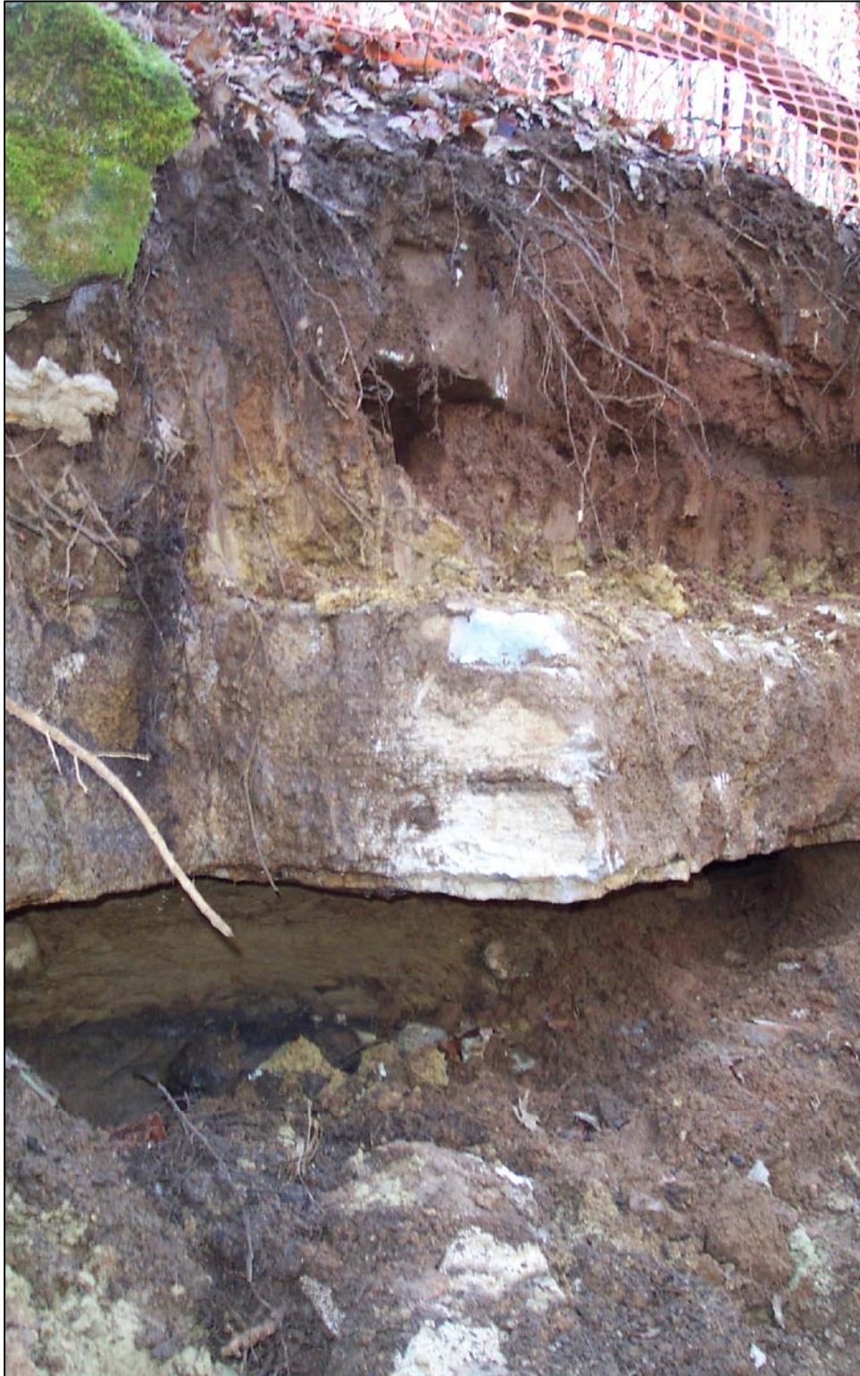
PHOTO No. 4: SPRING 018 EXPOSED, AFTER INITIAL REMOVAL ACTION EXCAVATION. NOV. 2004
