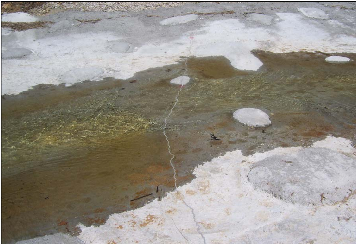
PHOTO No. 41: TYPICAL CRACK REPAIR USING QUIKRETE BRAND CRACK SEALANTS. APR. 2013
