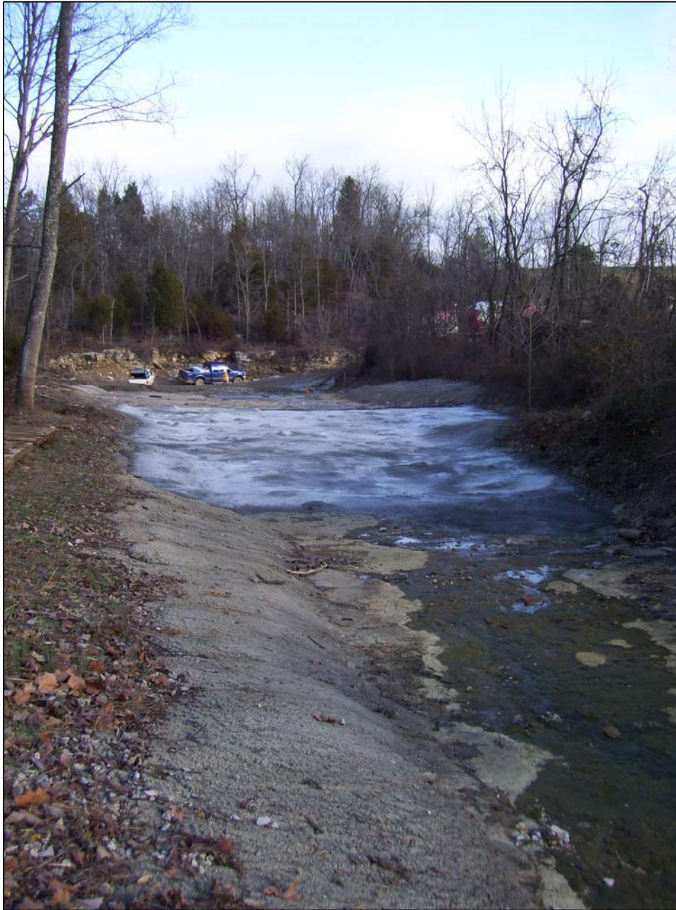
PHOTO No. 20: TRIBUTARY 3 CONCRETE SEALING WORK LOOKING DOWNSTREAM. DEC. 2012
