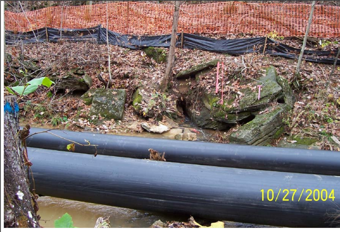
PHOTO No. 3: SPRING 018 PRE-EXCAVATION. OCT. 2004
