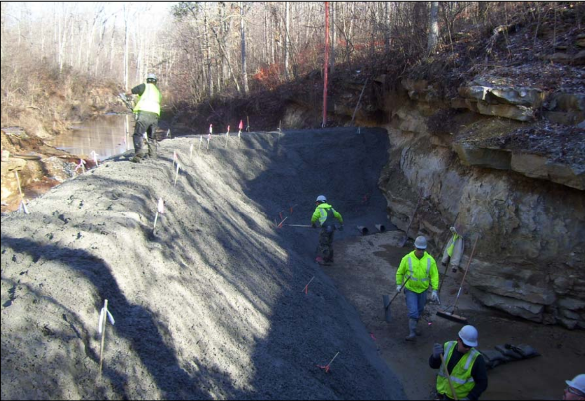
PHOTO No. 24: PLACING CONCRETE ON THE SPRING 018 CONTAINMENT BERM. DEC. 2012
