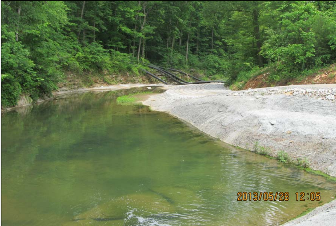
PHOTO No. 38: POND CONSTRUCTED WITHIN CREEK UPSTREAM OF SPRING 018. MAY 2013
