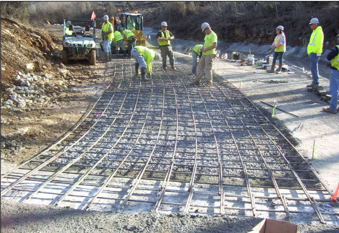
PHOTO No. 33: LAYING OF REBAR MATTING OVER GLC FEB. 2012
