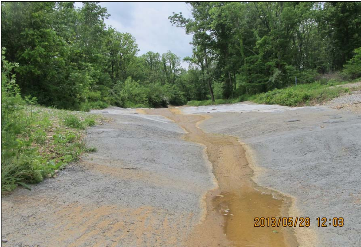
PHOTO No. 35: COMPLETED CONCRETE LOOKING UPSTREAM ALONG SEALED TRIBUTARY 3. MAY 2013
