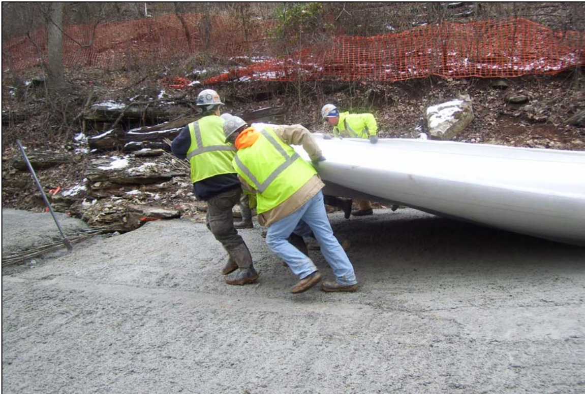
PHOTO No. 29: PLACING GEOSYNTHETIC CLAY LINER (GCL), FEB. 2012
