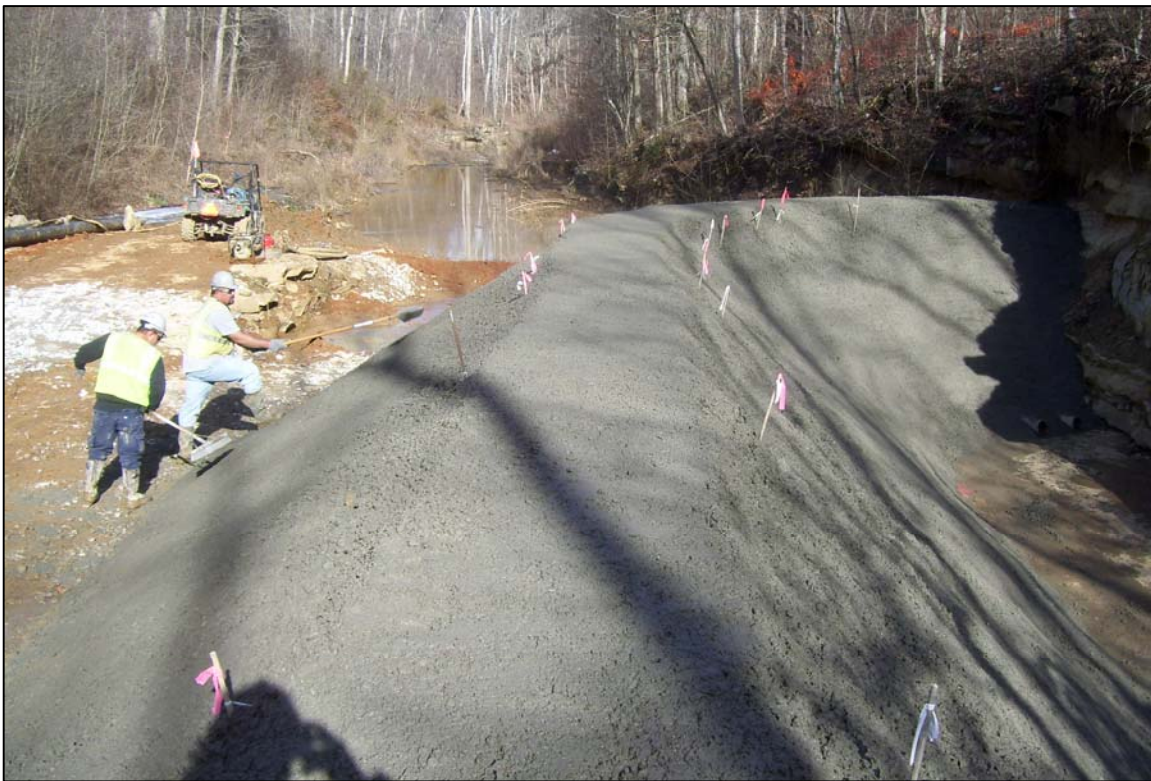
PHOTO No. 25: FINAL CONCRETE ON THE SPRING 018 CONTAINMENT BERM. DEC. 2012
