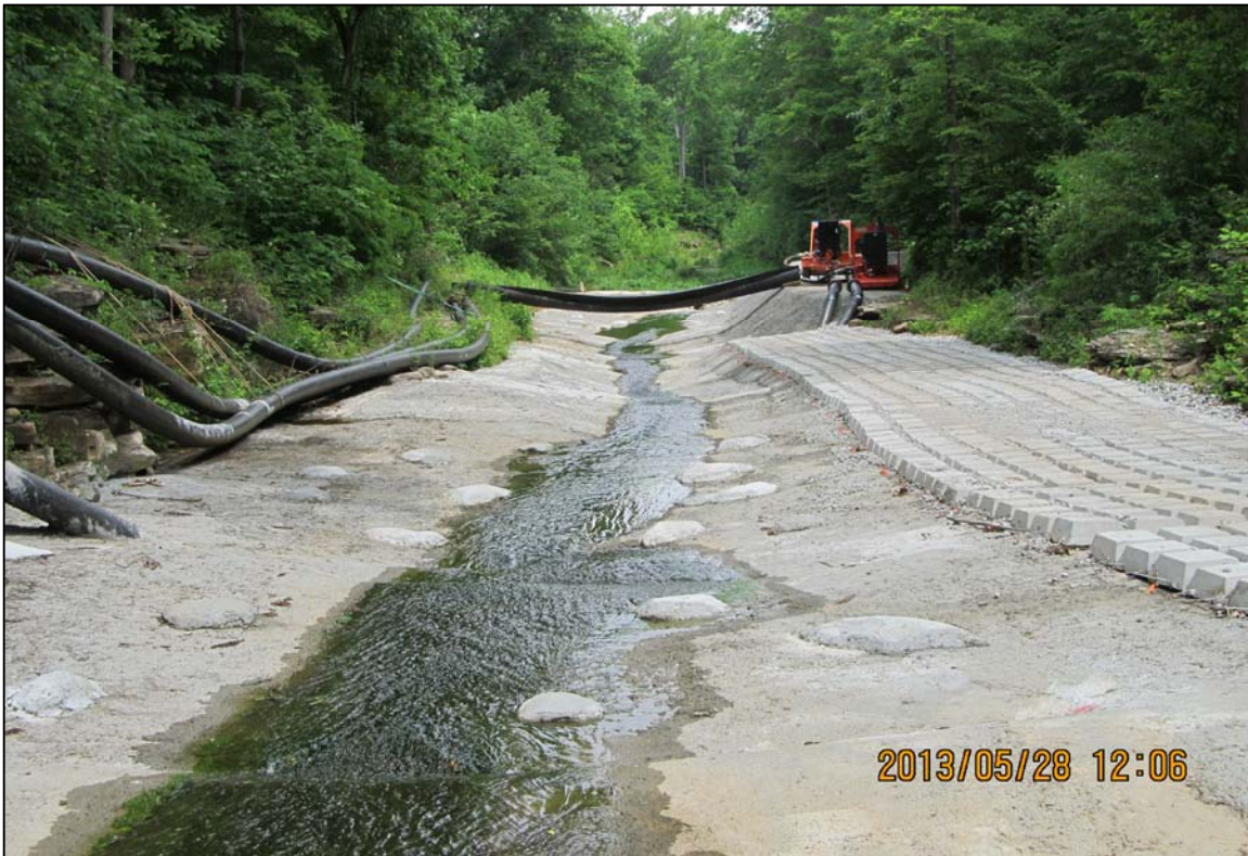
PHOTO No. 39: FACING DOWNSTREAM AT SPRING 018 CONTAINMENT BERM AND PUMPS. MAY 2013
