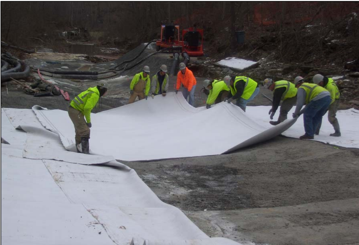
PHOTO No. 30: PLACING GEOSYNTHETIC CLAY LINER (GCL), FEB. 2012
