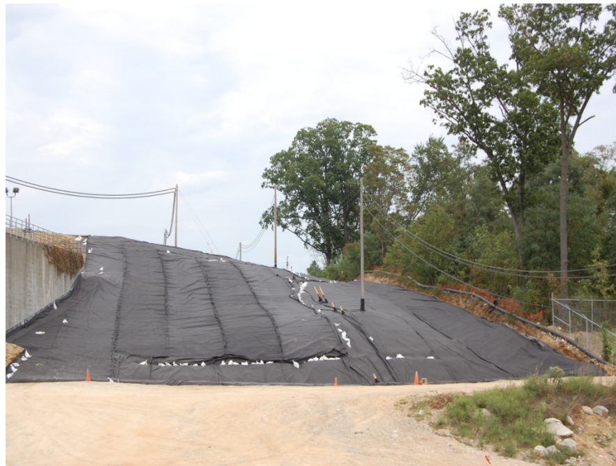
Photo No.34: AOI-11 - Drainage Geocomposite Material (Facing North). September 2010
