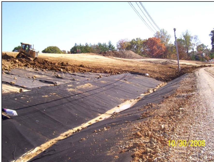
Photo No.46: East AOI-10 - Common fill placement (Facing Southeast). October 2008
