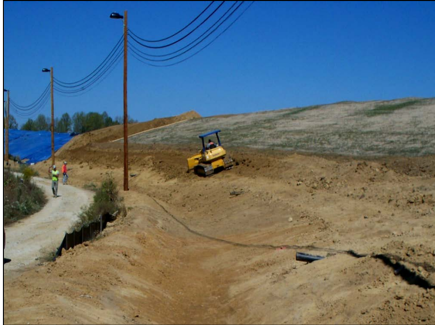
Photo No.53: East AOI-10 – Topsoil placement (Facing Northeast). October 2010
