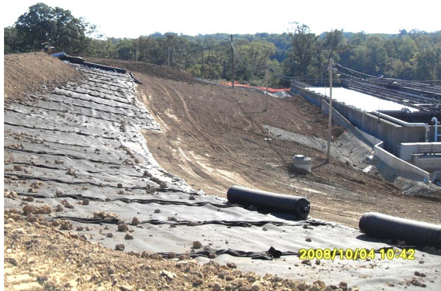
Photo No.33: AOI-11 - Drainage Geocomposite Material Installation (Facing East). October 2008
