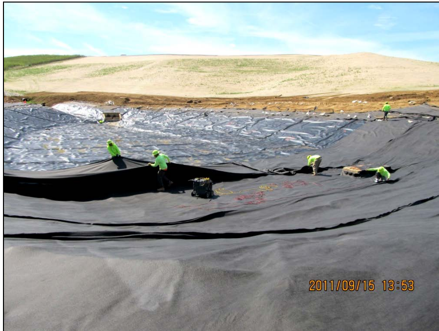
Photo No.40: Detention Basin 5 - Drainage geocomposite material installation (Facing West). September 2011
