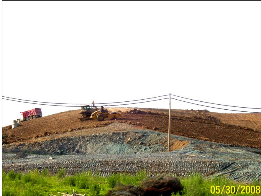
Photo No.11: AOI-6 – Clay Barrier Layer Placement (Facing North). May 2008
