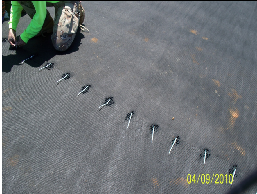
Photo No.31: Parcel 201 - Drainage geocomposite material installation (Facing Downwards). April 2010
