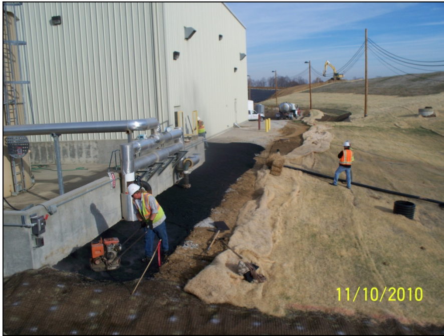
Photo No.81: AOI-5 - Asphalt Cover System (Facing North). November 2010
