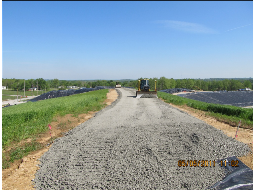
Photo No.77: AOI-5 - Access Road Construction (Facing North). May 2011
