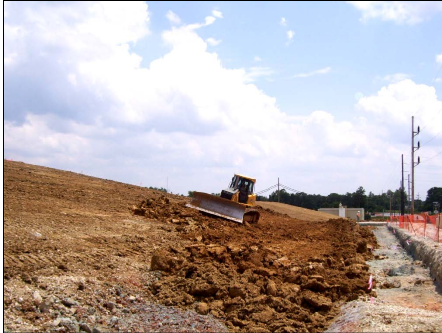
Photo No.17: AOI-5 - Clay Barrier Layer Placement (Facing South). July 2008
