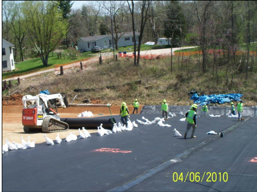
Photo No.21: Parcel 201 - LLDPE liner installation (Facing Southeast). April 2010
