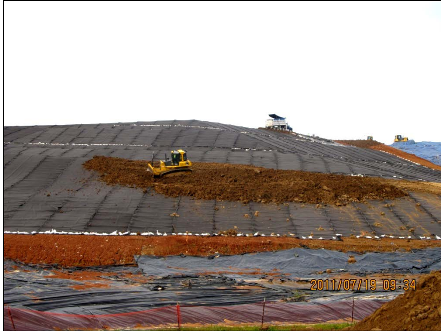
Photo No.47: AOI-4 - Common fill placement (Facing Southwest). July 2011
