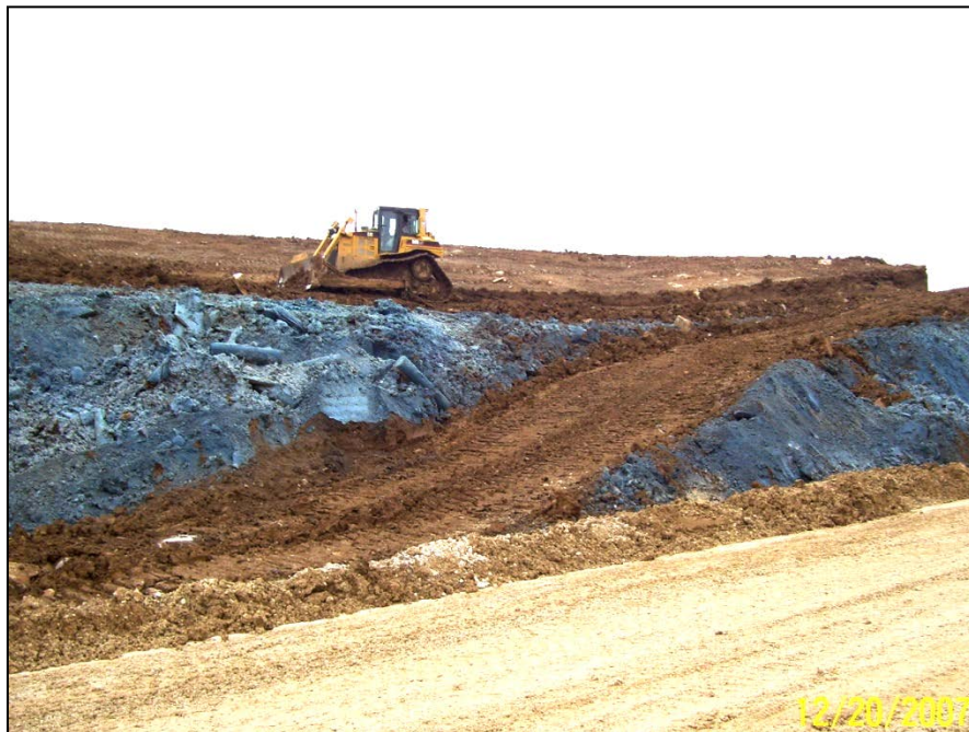
Photo No.10: AOI-4 - Grading Fill Placement (Facing North). December 2007
