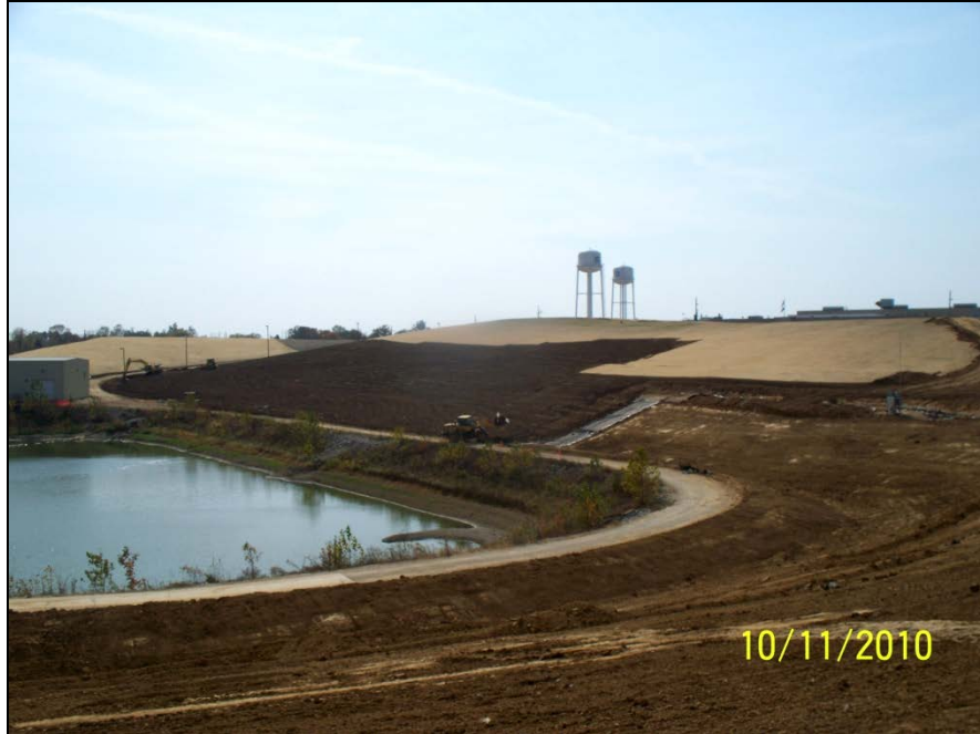
Photo No.57: AOI-5 - Topsoil placement (Facing Southwest). October 2010
