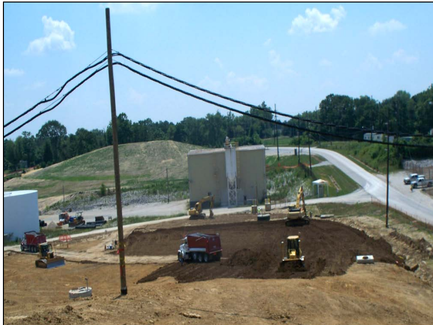
Photo No.54: AOI-8 - Topsoil placement (Facing South). July 2010
