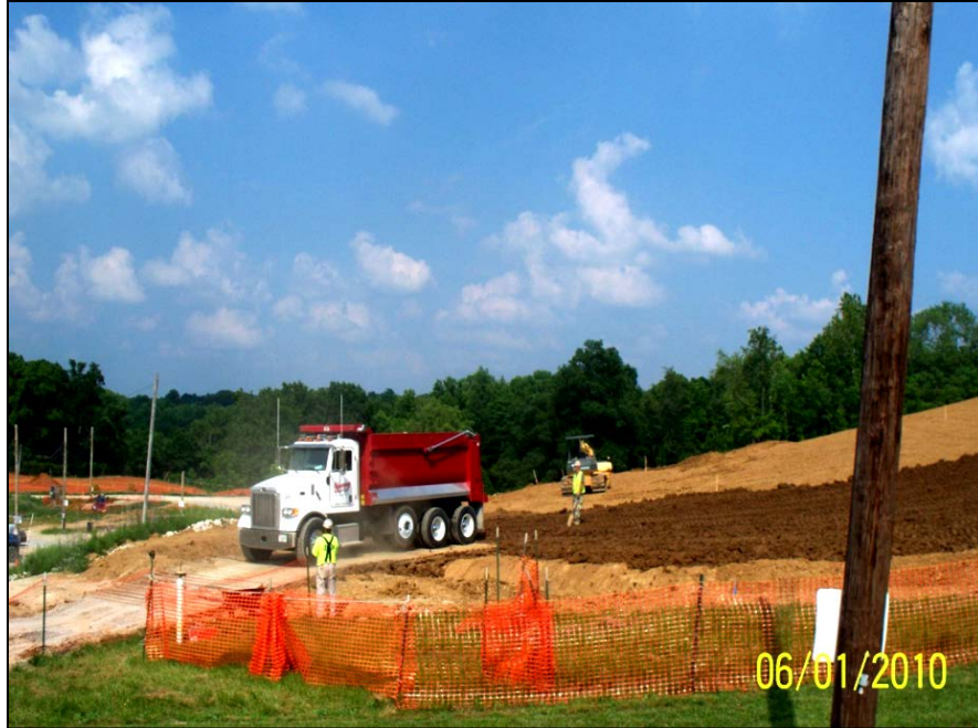
Photo No.51: Parcel 201 - Topsoil placement (Facing East). June 2010
