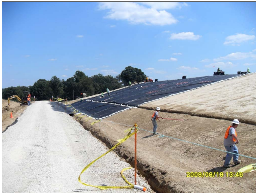
Photo No.24: AOI-6 - LLDPE liner installation (Facing East). August 2008
