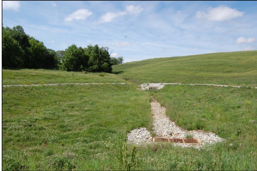
Photo No.73: East AOI-10 - Vegetative growth (Facing Southwest). June 2014
