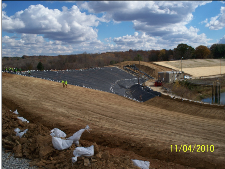
Photo No.29: AOI-4 - LLDPE liner installation (Facing East). November 2010
