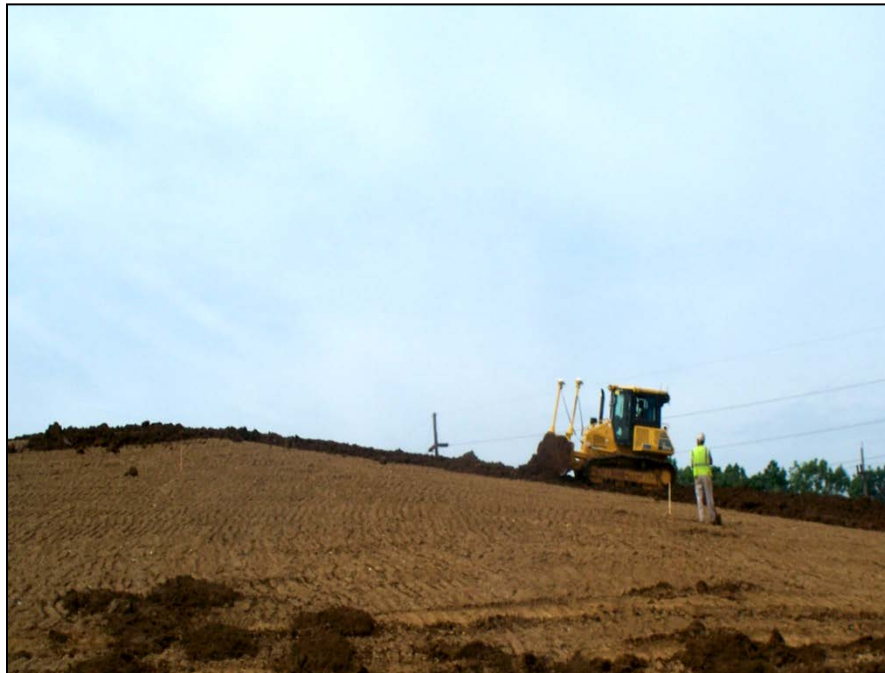
Photo No.52: Parcel 201 - Topsoil placement (Facing South). June 2010
