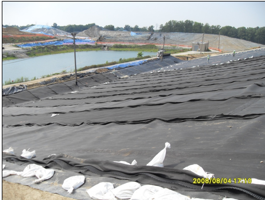
Photo No.36: East AOI-10 - Installed drainage geocomposite material (Facing Northwest). August 2008
