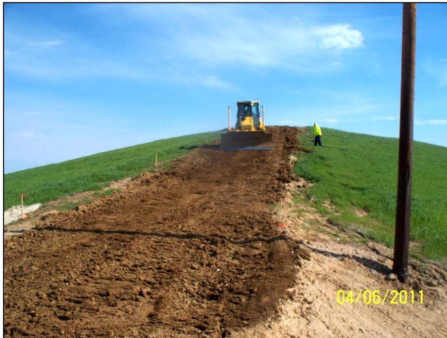
Photo No.74: AOI-5 - Access Road Construction (Facing Northeast). April 2011
