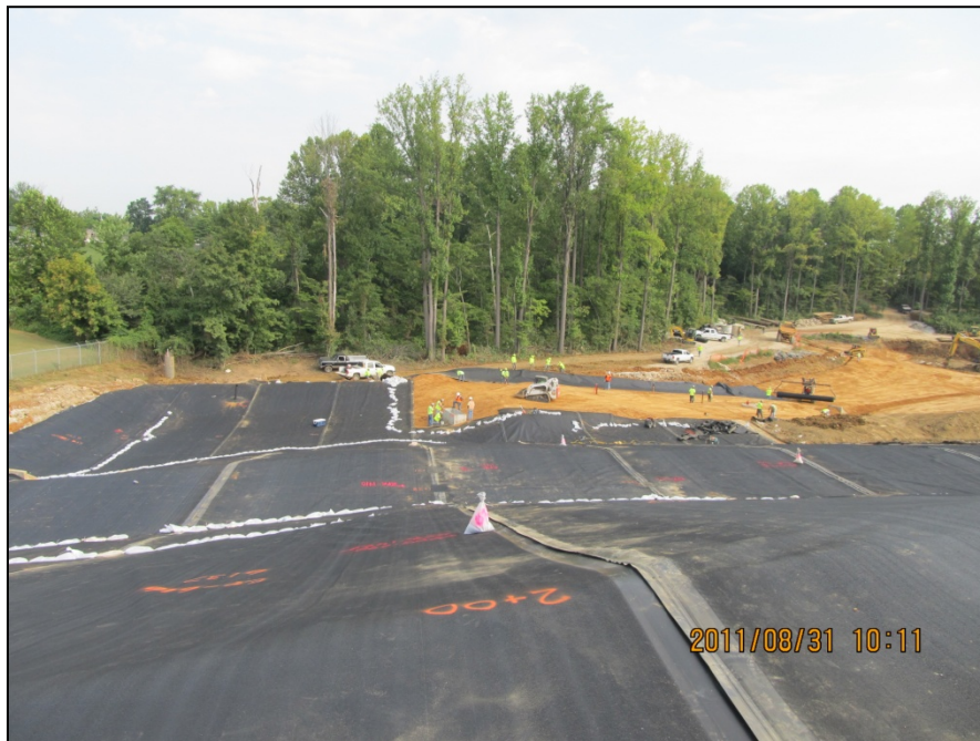
Photo No.30: AOI-4 - LLDPE liner installation (Facing North). August 2011
