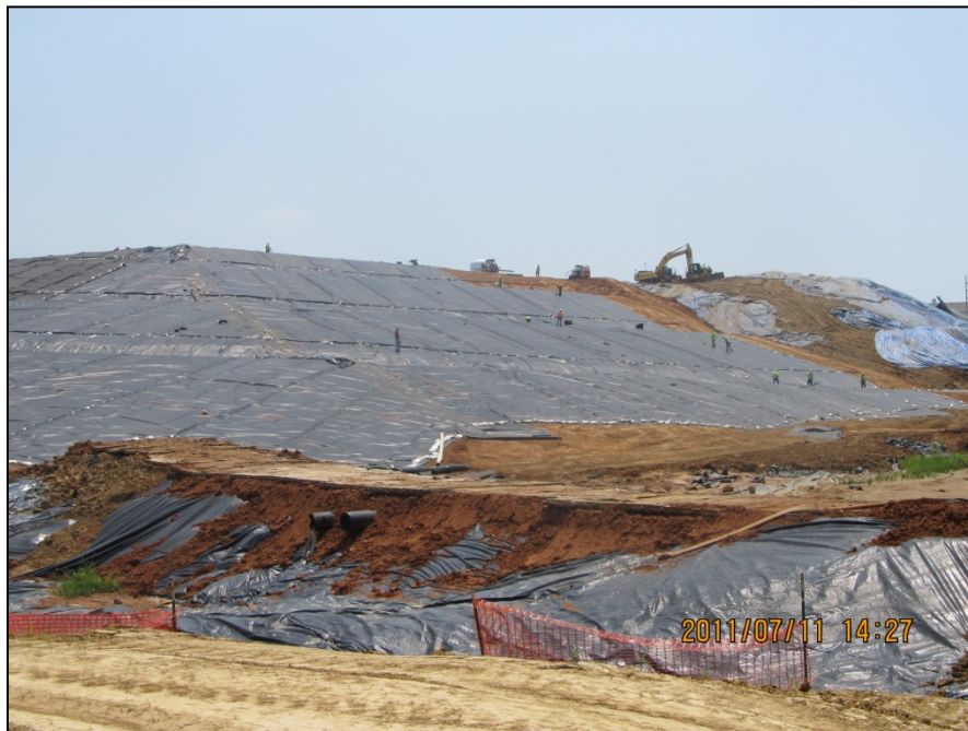
Photo No.28: AOI-4 - LLDPE liner installation (Facing South). July 2011
