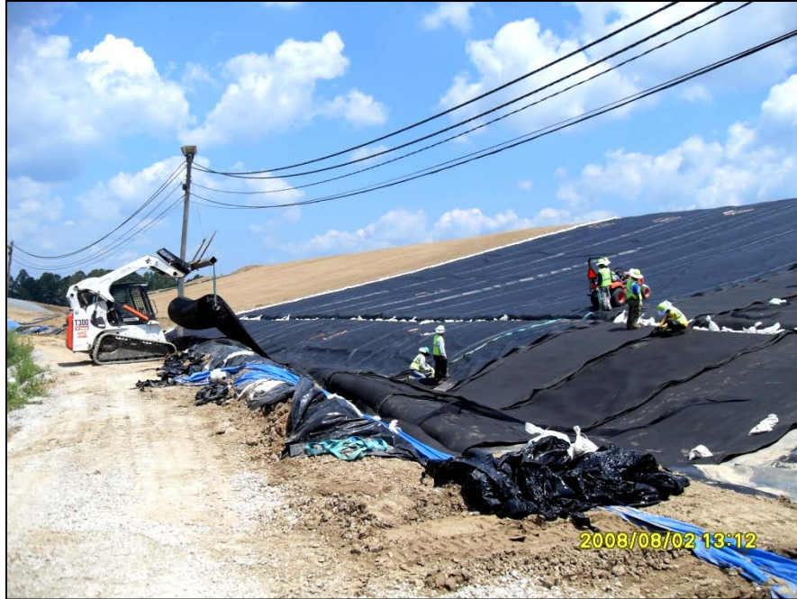
Photo No.35: East AOI-10 - Drainage geocomposite material installation (Facing North). August 2008
