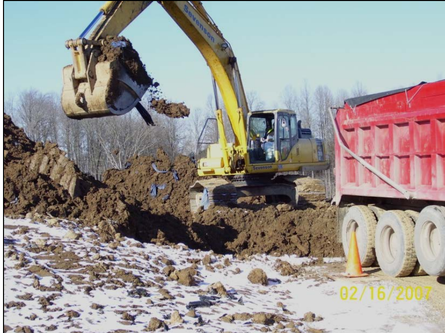
Photo No.1: East AOI-4 – Grading Fill Placement (Facing North). February 2007
