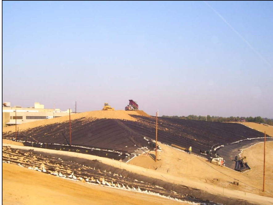
Photo No.43: AOI-5 – Common fill placement (Facing Northwest). October 2008
