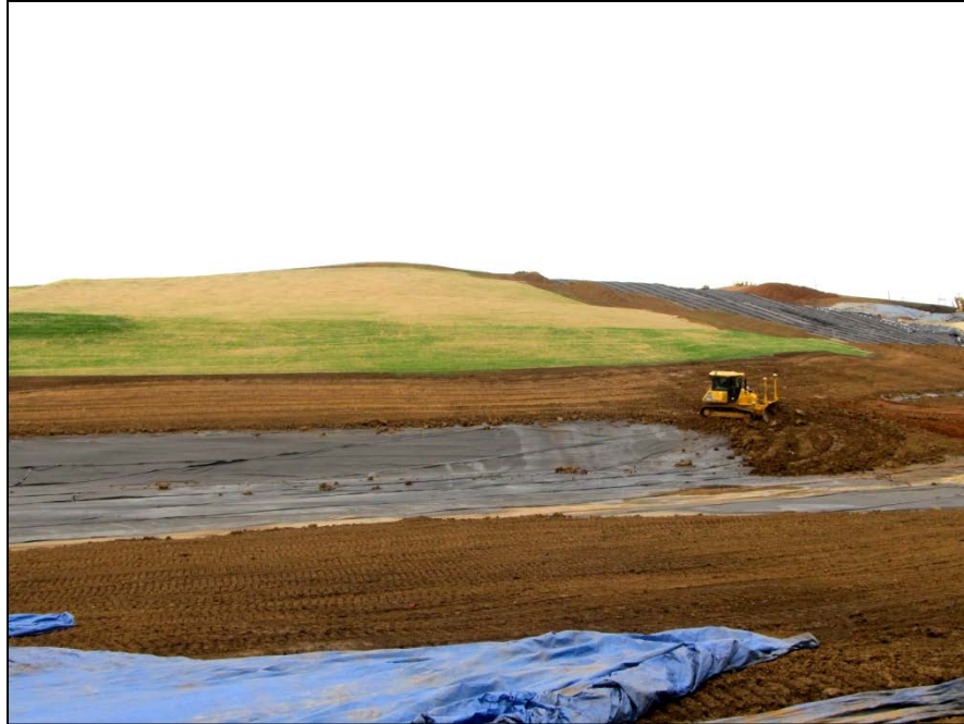
Photo No.49: AOI-4 – Common fill placement (Facing South). September 2011
