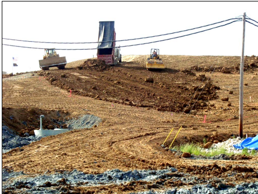
Photo No.14: AOI-6 - Clay Barrier Layer Placement (Facing North). May 2008
