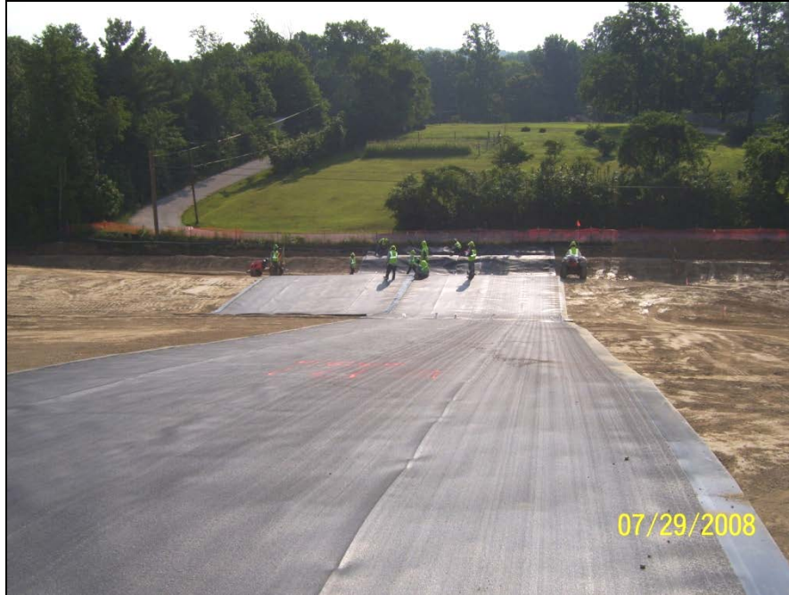
Photo No.25: East AOI-10 - LLDPE liner installation (Facing East). July 2008
