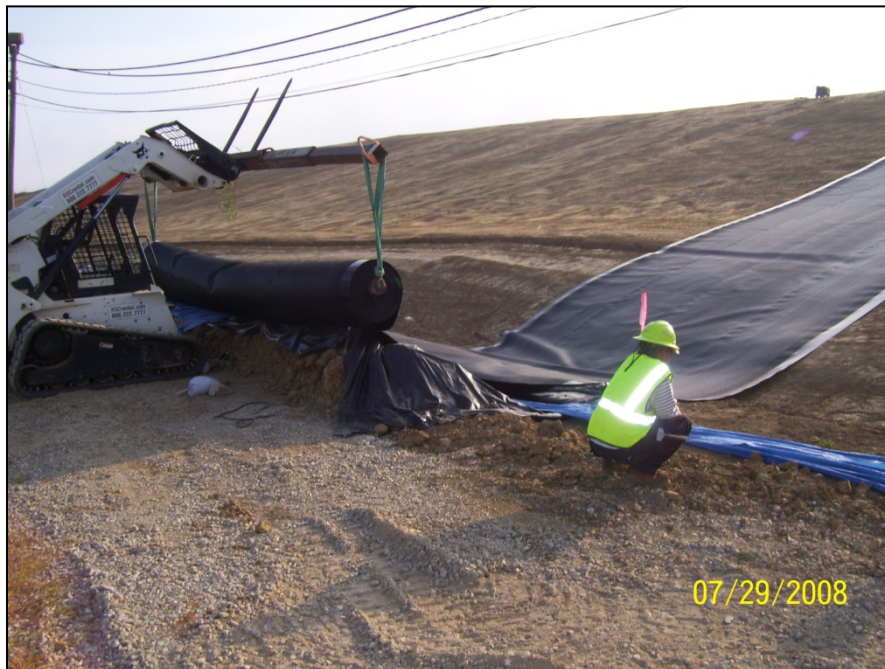
Photo No.26: East AOI-7 - LLDPE Liner Installation (Facing Southeast). July 2008
