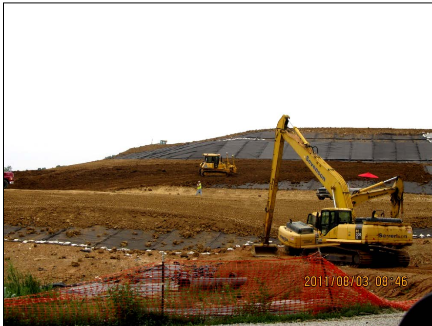
Photo No.50: AOI-4 - Common fill placement (Facing South). August 2011
