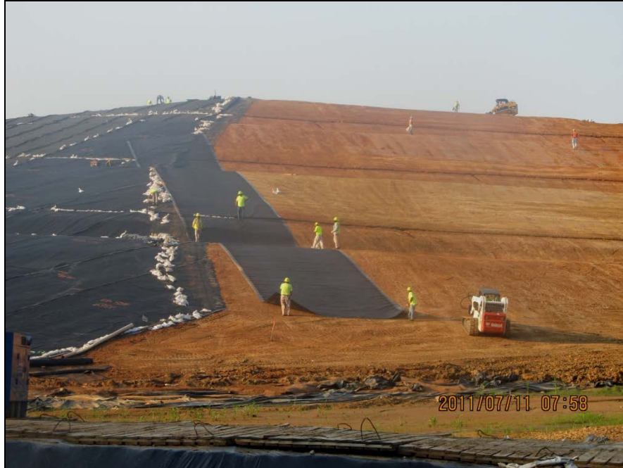
Photo No.27: AOI-4 - LLDPE liner installation (Facing South). July 2011
