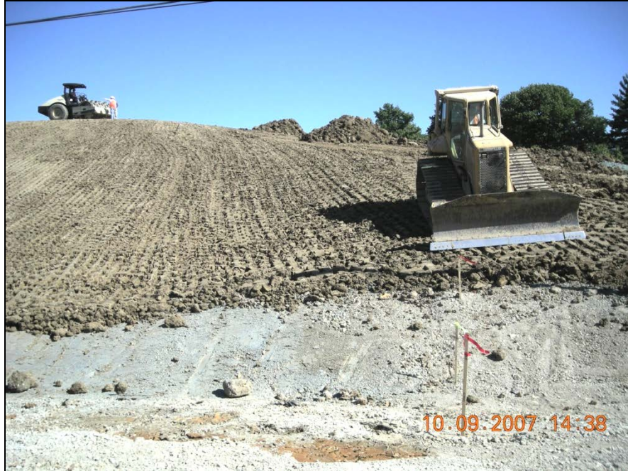
Photo No.15: East AOI-10 - Clay Barrier Layer Placement (Facing Northeast). October 2007
