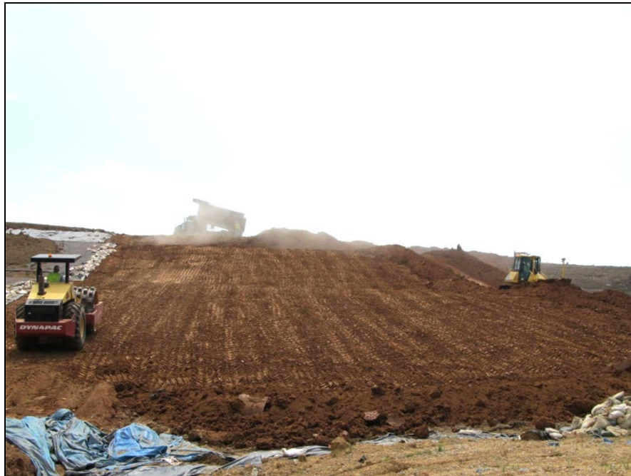
Photo No.20: AOI-15 - Clay Barrier Layer Placement (Facing South). August 2011
