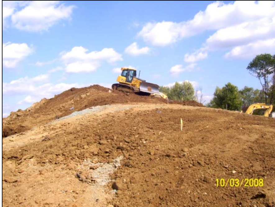
Photo No.5: Parcel 201 - Grading Fill Placement (Facing Northeast). October 2008
