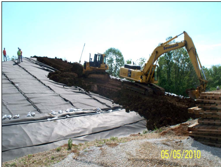
Photo No.42: Parcel 201 - Common fill placement (Facing Southeast). May 2010
