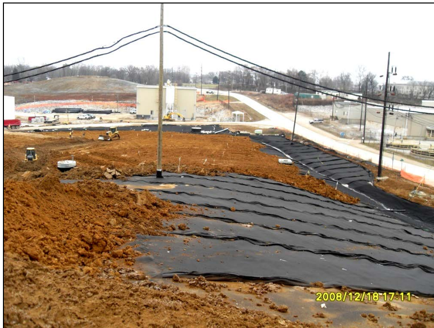
Photo No.44: AOI-6 - Common fill placement (Facing South). December 2008
