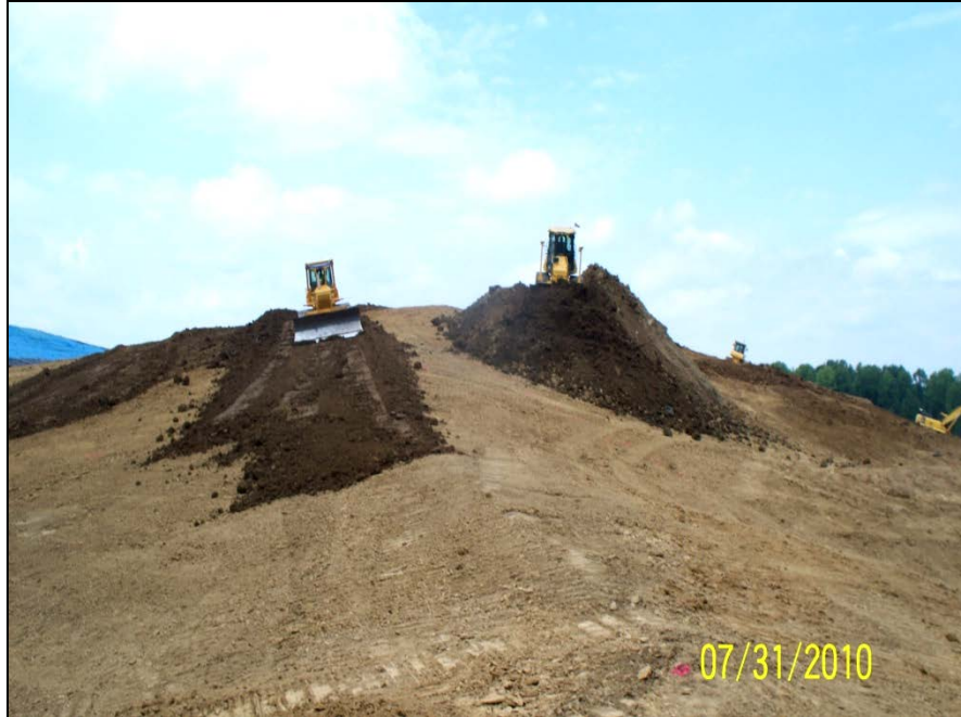
Photo No.55: East AOI-10 - Topsoil Placement (Facing Northeast). July 2010
