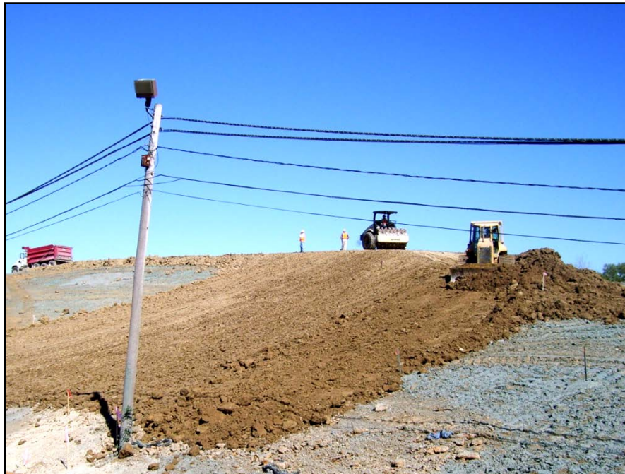
Photo No.16: East AOI-11 - Clay Barrier Layer Placement (Facing North). October 2007
