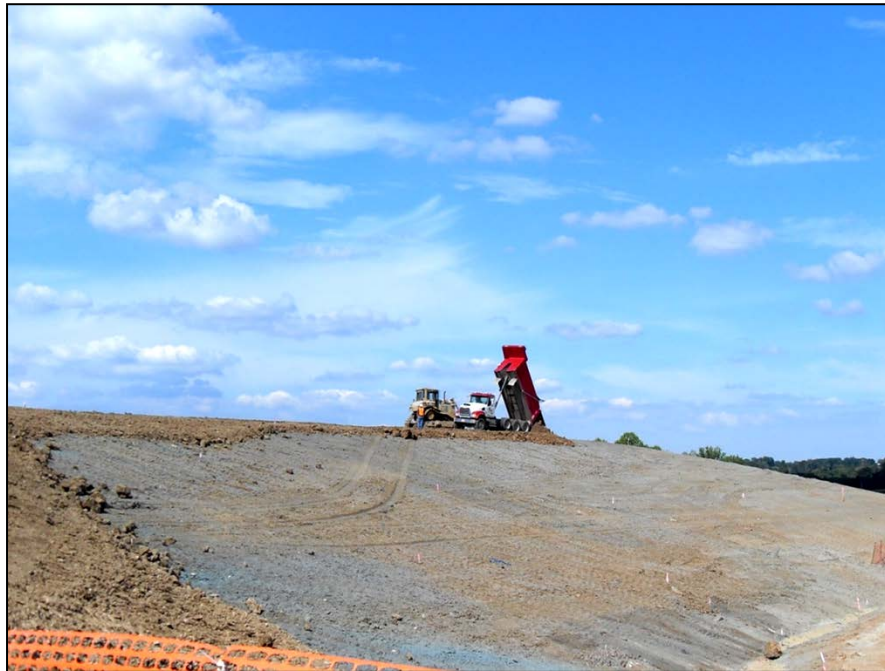
Photo No.18: AOI-5 - Clay Barrier Layer Placement (Facing Northwest). August 2008
