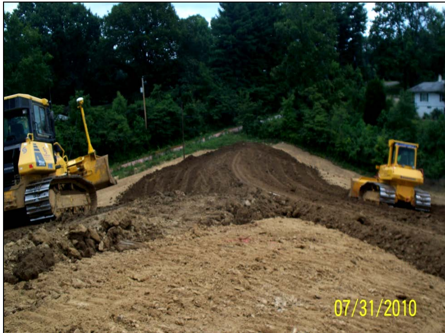
Photo No.56: East AOI-10 - Topsoil placement (Facing Southeast). July 2010
