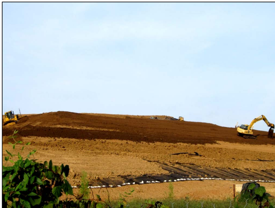
Photo No.60: AOI-4 - Topsoil placement (Facing West). August 2011
