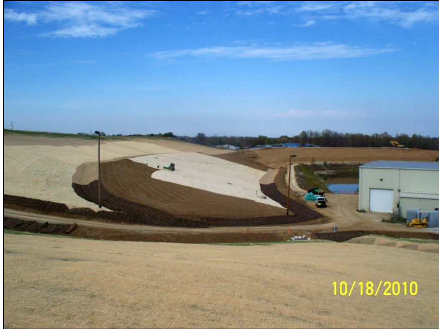
Photo No.65: AOI-5 - Erosion control matting placement (Facing North). October 2010
