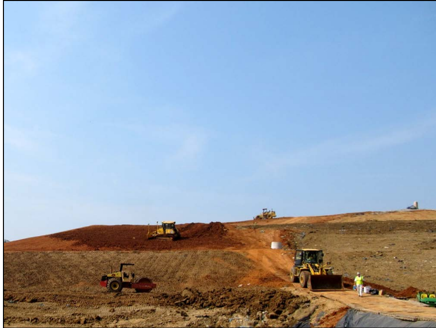
Photo No.19: AOI-4 - Clay Barrier Layer Placement (Facing South). June 2011
