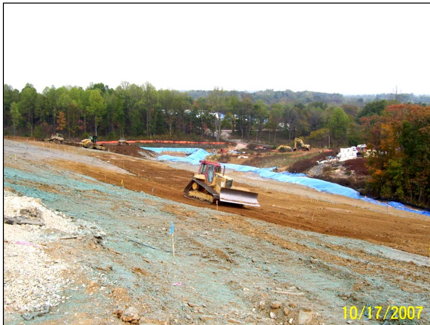
Photo No.8: East AOI-10 - Grading Fill Placement (Facing Northeast). October 2007
