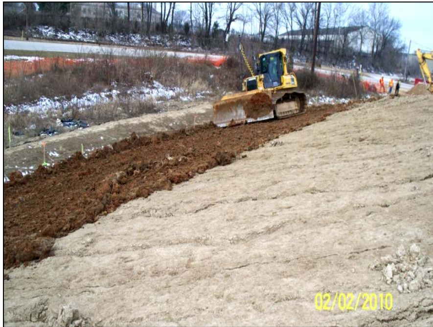
Photo No.12: Parcel 201 - Clay Barrier Layer Placement (Facing West). February 2010
