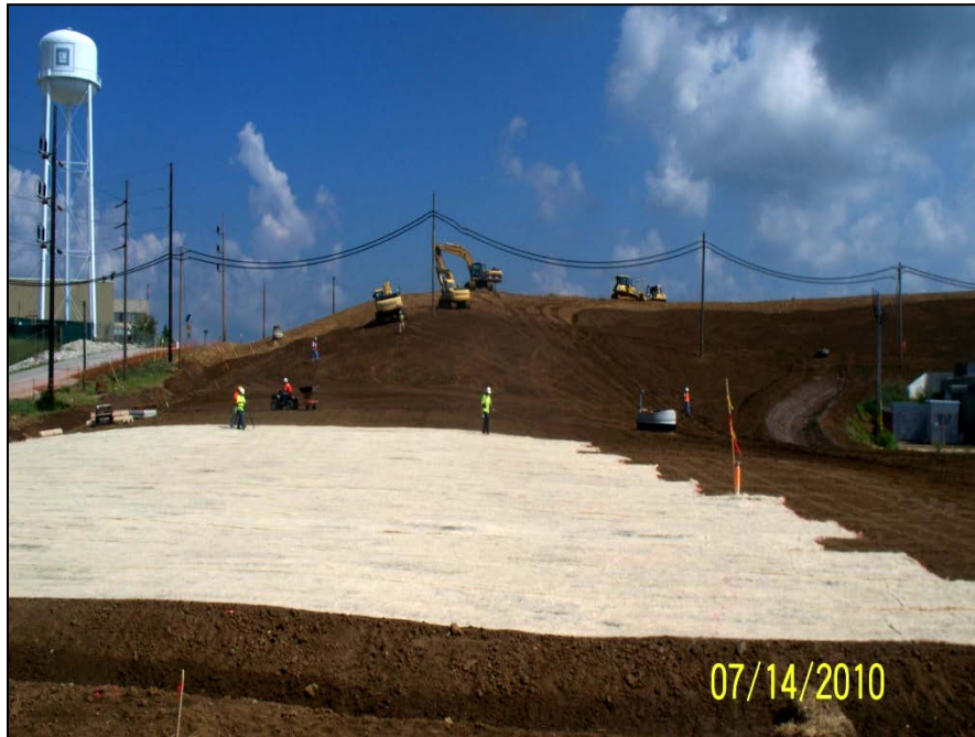
Photo No.62: AOI-8 - Erosion control matting placement (Facing North). July 2010
