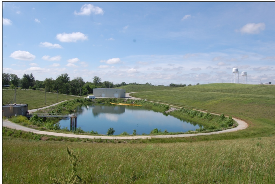
Photo No.70: AOI-10 - Vegetative growth (Facing South). June 2014
