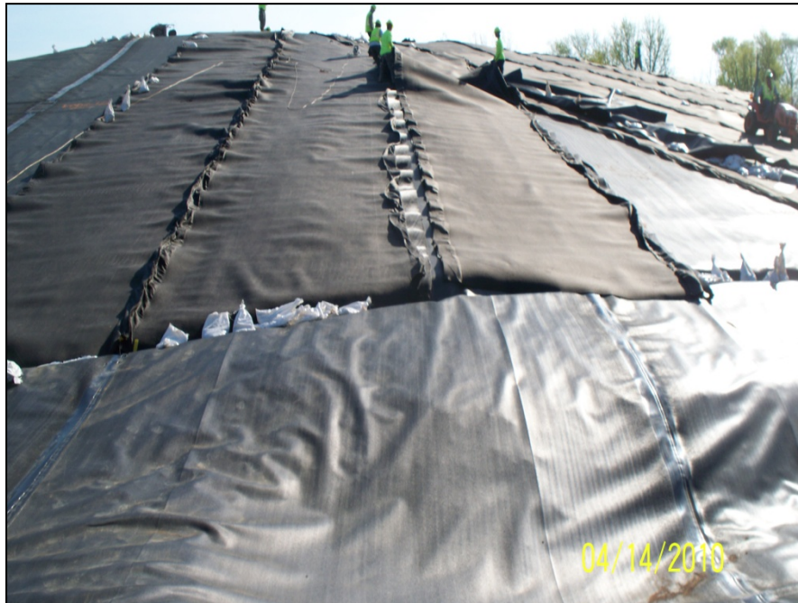
Photo No.32: Parcel 201 - Drainage geocomposite material installation (Facing South). April 2010
