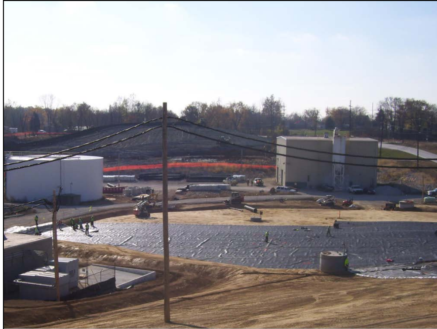
Photo No.23: AOI-8 - LLDPE liner installation (Facing South). November 2008
