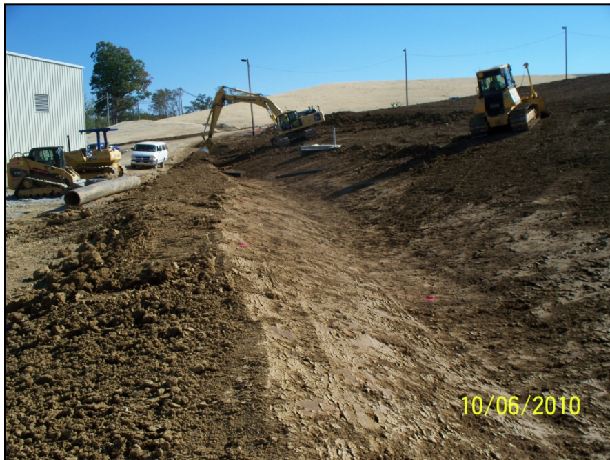
Photo No.58: AOI-5 - Topsoil placement (Facing Southeast). October 2010
