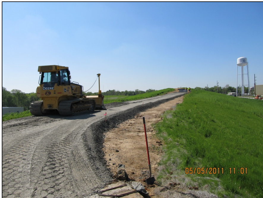
Photo No.76: AOI-5 - Access Road Construction (Facing South). May 2011
