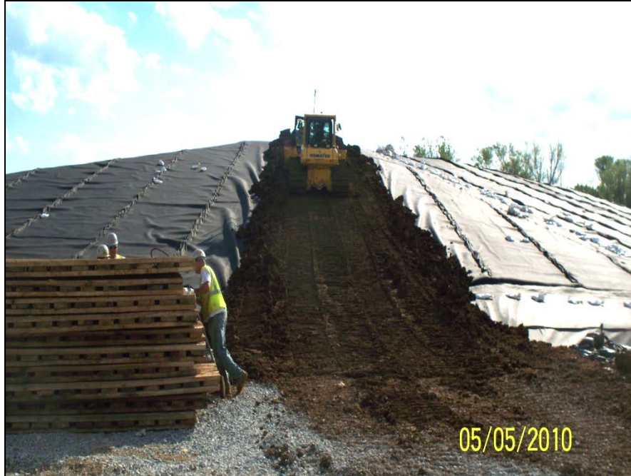
Photo No.41: Parcel 201 - Common fill placement (Facing Northeast). May 2010
