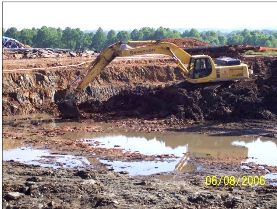
Photo No.2: AOI-5 – 750 ppm Excavation Activities (Facing East). June 2006
