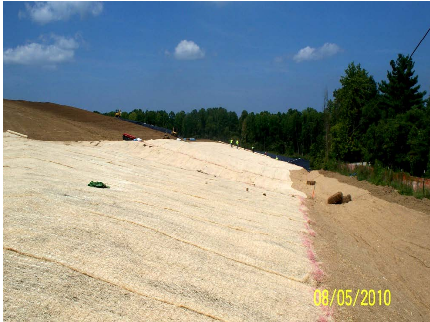
Photo No.64: East AOI-10 - Erosion control matting placement (Facing North). August 2010
