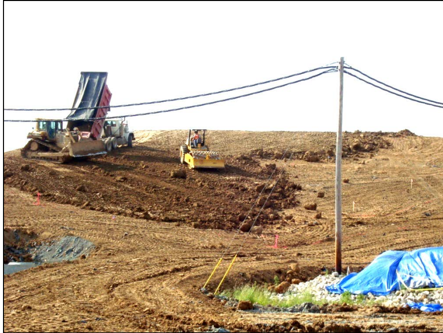
Photo No.13: AOI-6 - Clay Barrier Layer Placement (Facing North). May 2008
