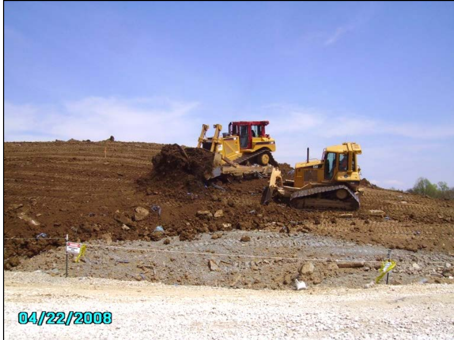
Photo No.9: AOI-5 - Grading Fill Placement (Facing Northeast). April 2008
