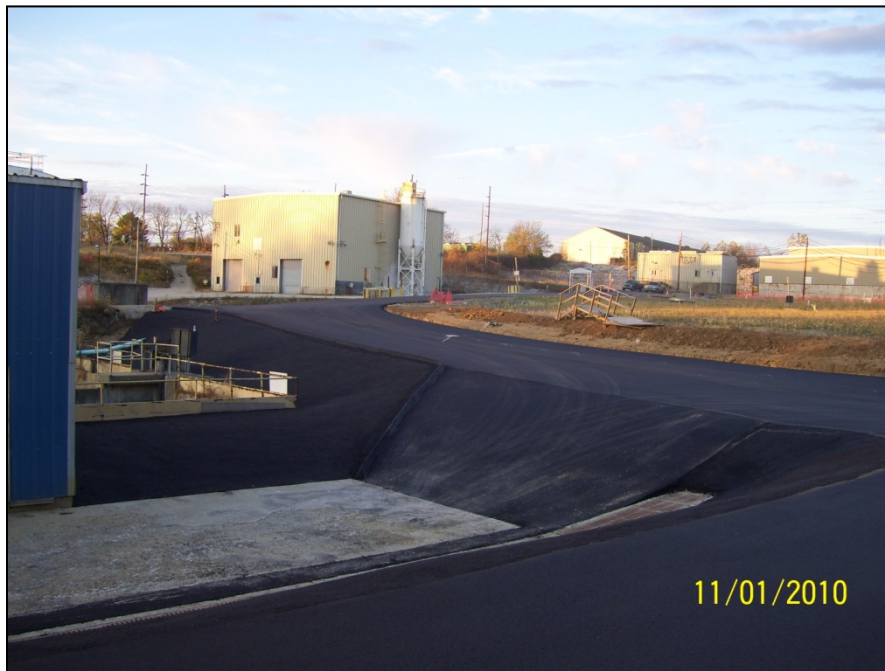
Photo No.80: AOI-8 - Asphalt Cover System (Facing Southwest). November 2010
