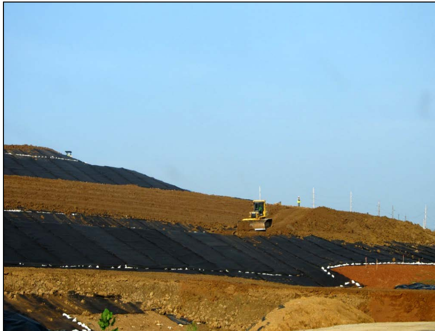
Photo No.48: AOI-4 - Common fill placement (Facing Southwest). July 2011
