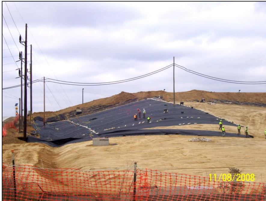
Photo No.22: AOI-8 - LLDPE liner installation (Facing North). November 2008
