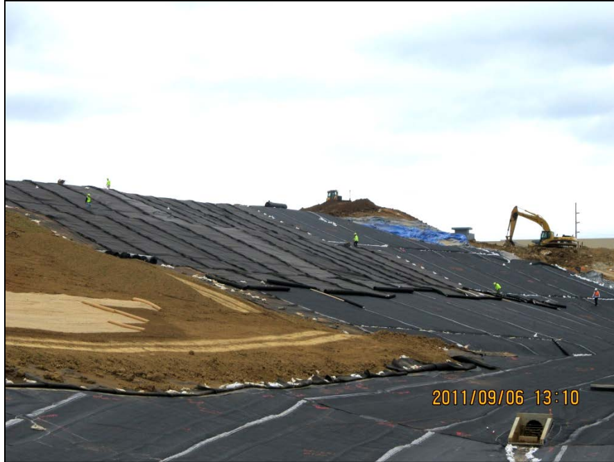
Photo No.39: AOI-4 - Drainage geocomposite material installation (Facing Southwest). September 2011
