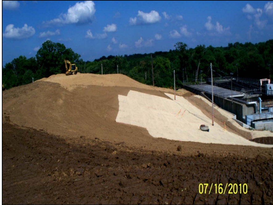
Photo No.63: AOI-11 - Erosion control matting placement (Facing East). July 2010
