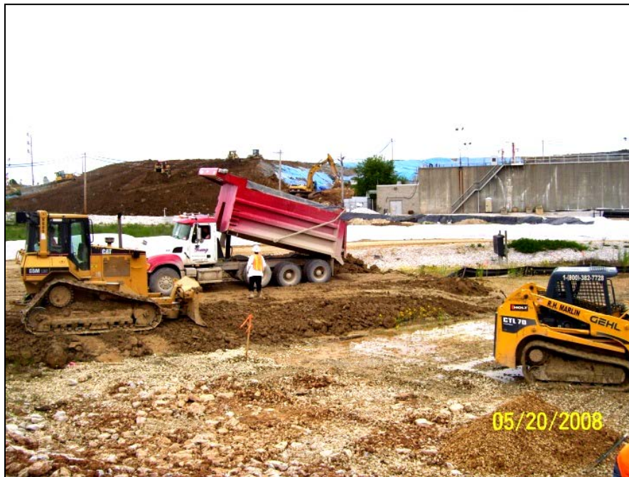
Photo No.4: AOI-8 - Access Road Construction (Facing North). May 2008
