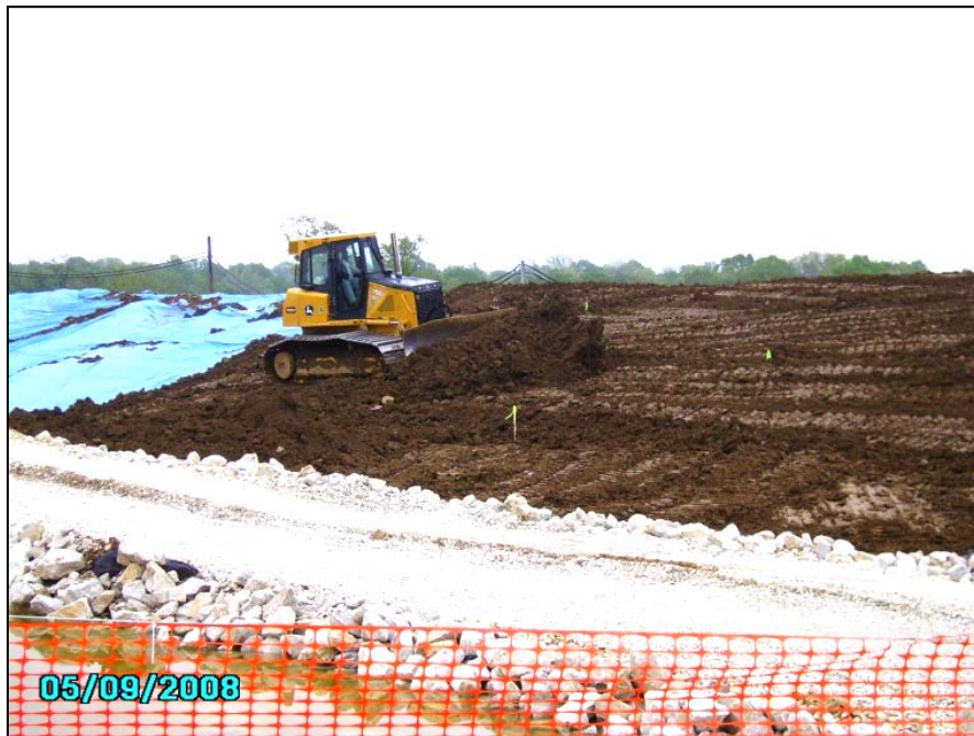
Photo No.6: AOI-6 - Grading Fill Placement (Facing Southeast). May 2008
