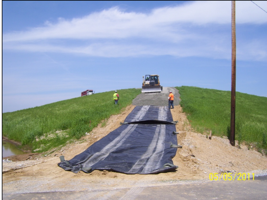
Photo No.75: AOI-5 - Access Road Construction (Facing East). May 2011
