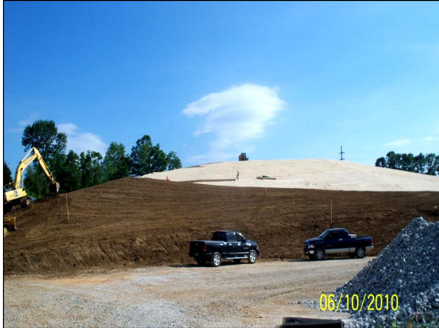
Photo No.61: Parcel 201 - Erosion control matting placement (Facing South). June 2010
