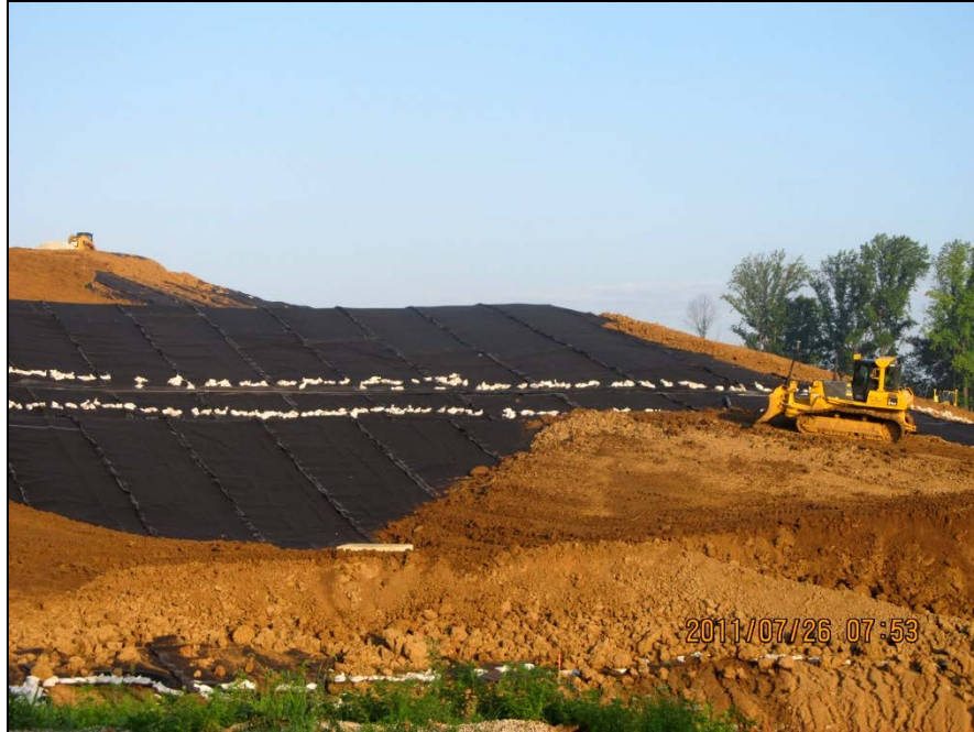
Photo No.45: East AOI-10 - Common fill placement (Facing West). July 2011
