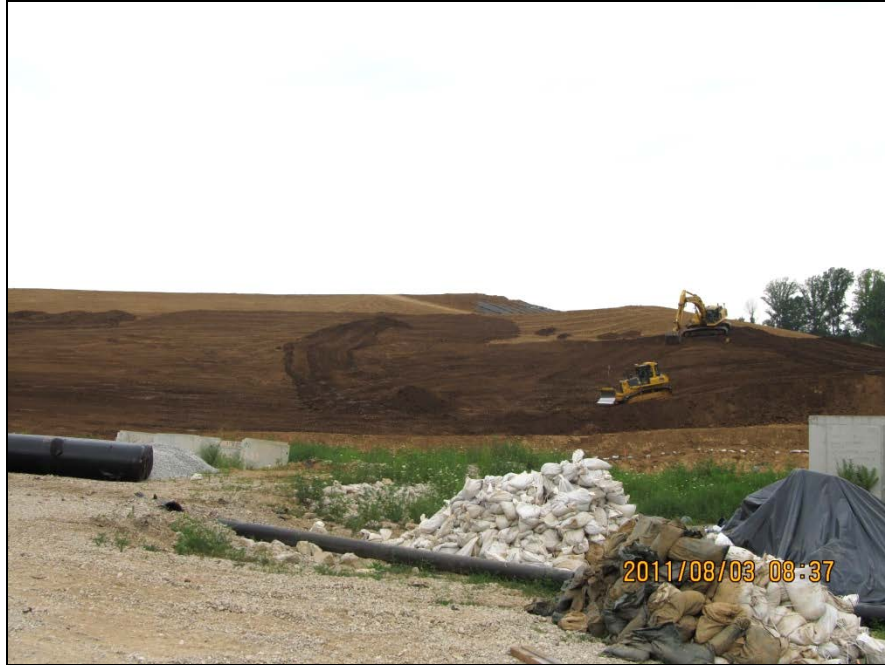
Photo No.59: AOI-4 - Topsoil placement (Facing West). August 2011
