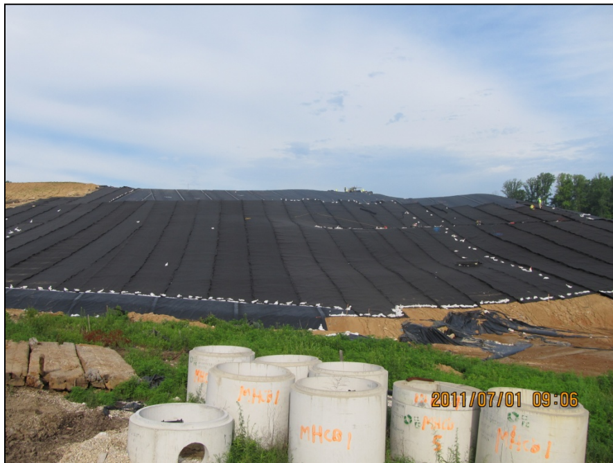
Photo No.38: AOI-10 – Drainage geocomposite material installation (Facing West). July 2011
