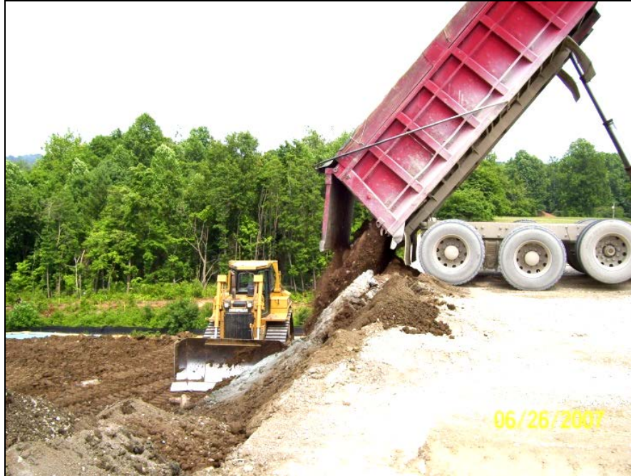
Photo No.7: East AOI-10 - Grading Fill Placement (Facing East). June 2007
