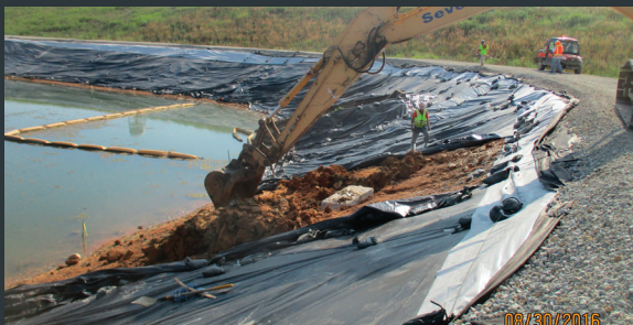
SETTING CONCRETE CABLE GUIDE FOR DREDGING
