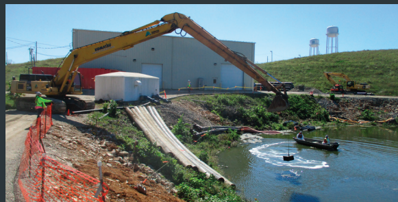
CLEARING CONCRETE BLOCKS FROM POND
