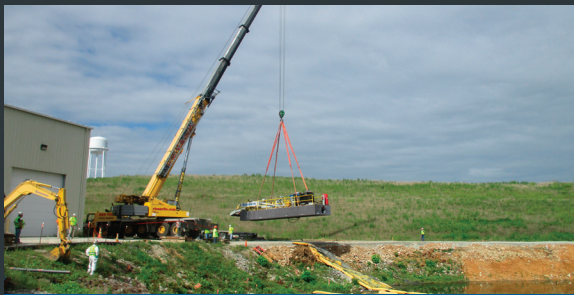
LIFTING DREDGE INTO STORMWATER POND
