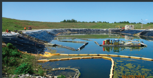
FLOAT LINES BEING CONNECTED TO DREDGE
