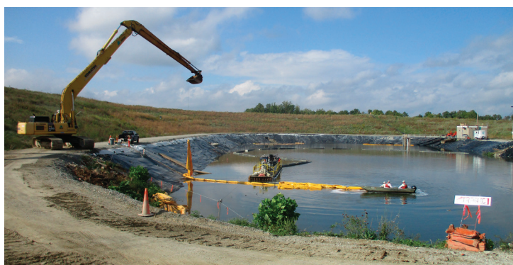
SLIT CURTAIN BEING DEPLOYED IN POND
