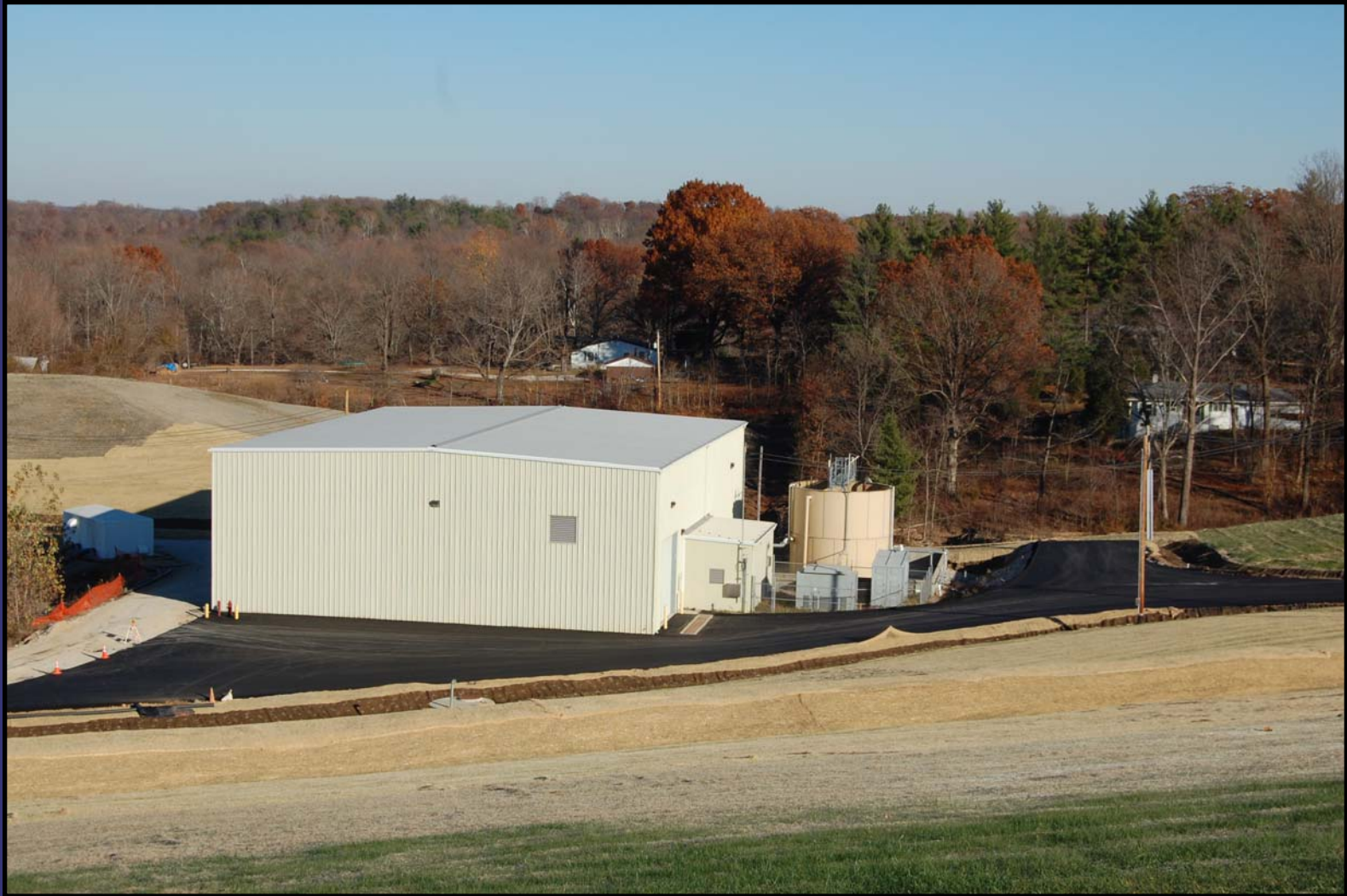
Completed asphalt cover work around the water treatment facility.
