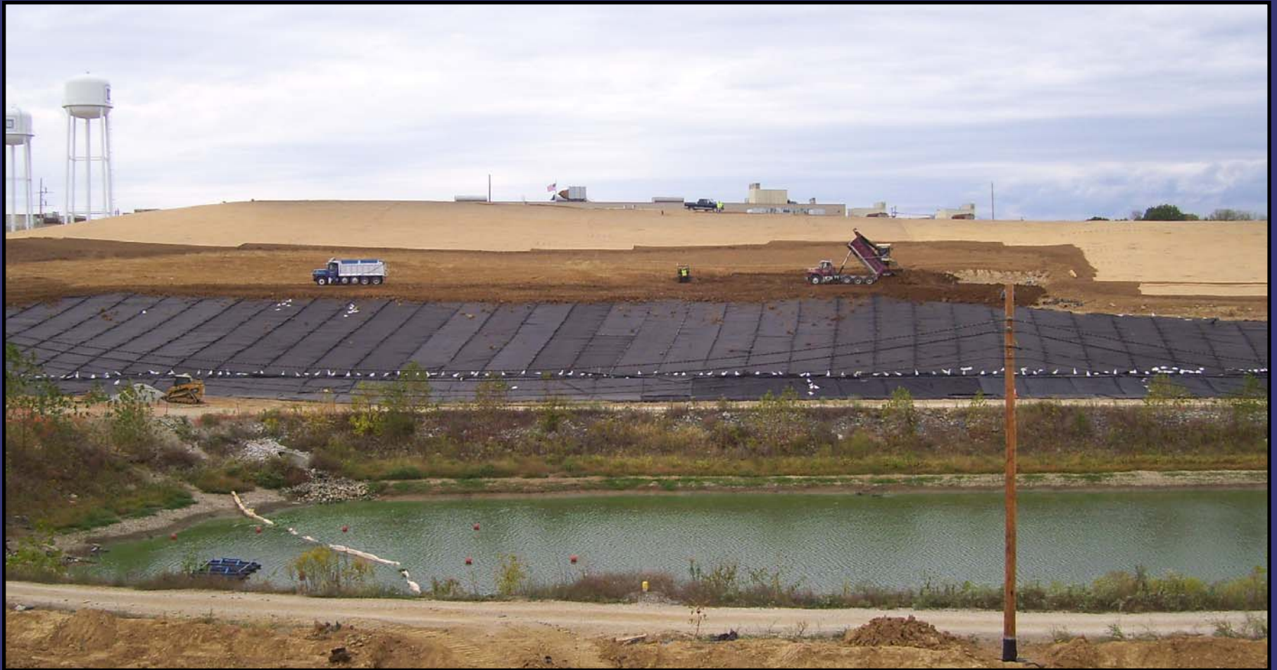
Placing clean soil over liner.
