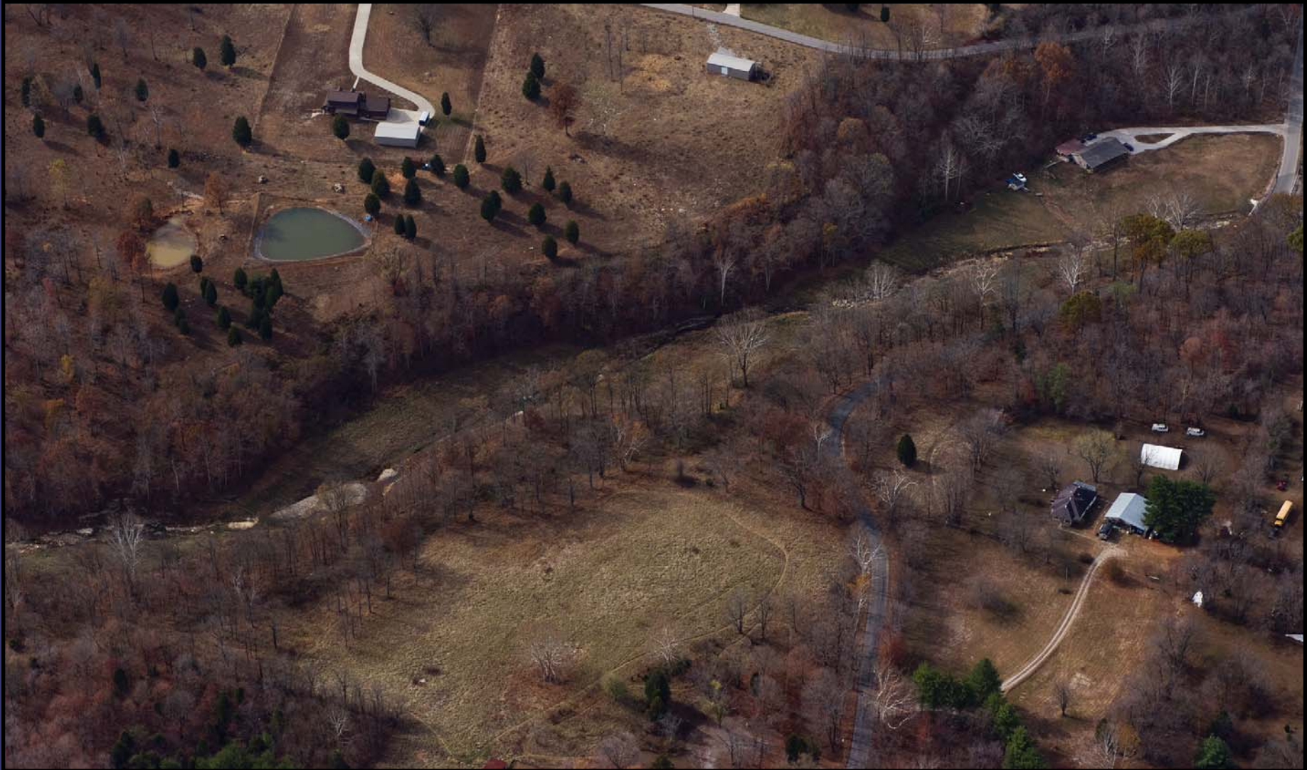
South of Broomsage Road Restoration
