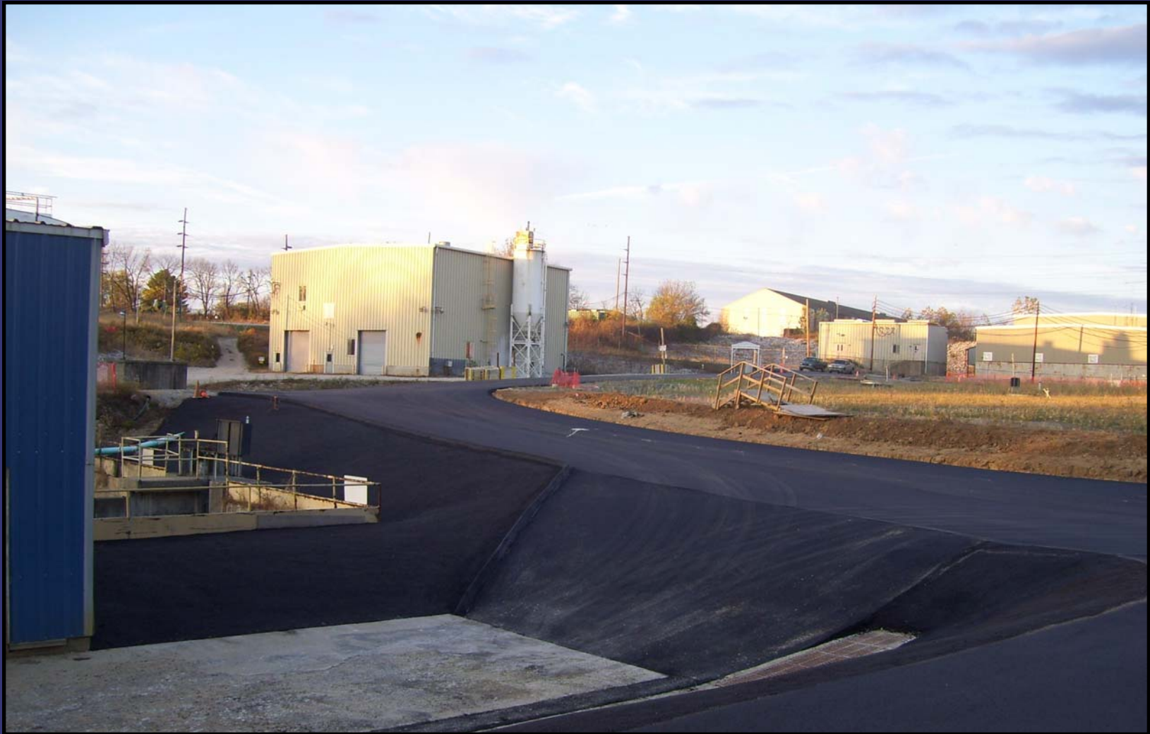
Close-up of the asphalt cover installed at the water treatment facility.
