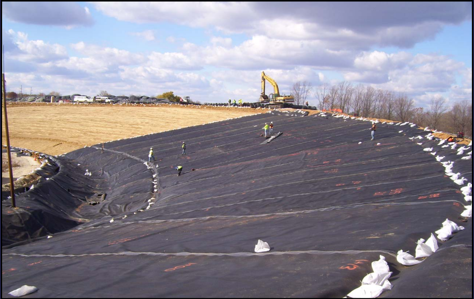
Workers checking liner seams north of the stormwater pond.
