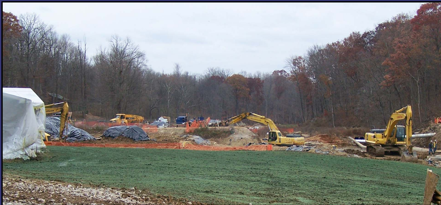
Property south of Broomsage Road restoration
