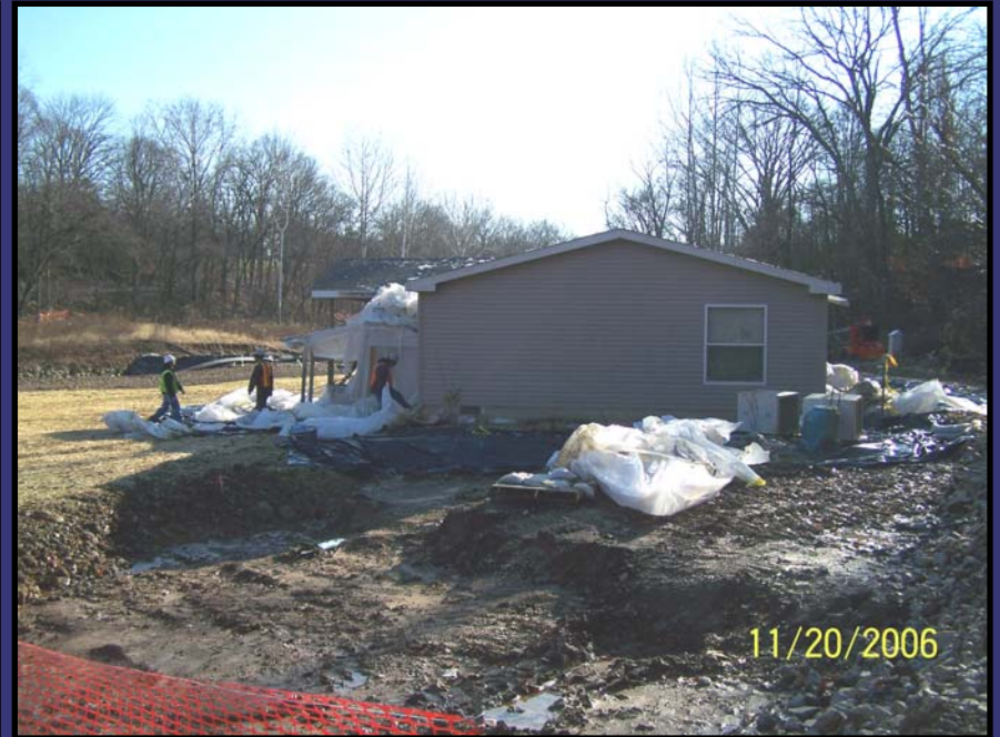
Property south of Broomsage Road
