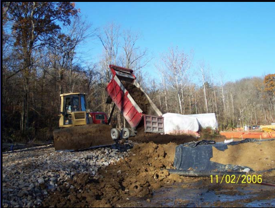
Property south of Broomsage Road restoration
