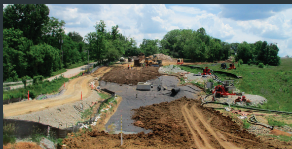
LINER WORK RESTORATION
