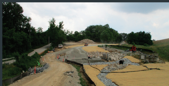
ACCESS ROAD TO WET WELL #4 AND AROUND DB-4
