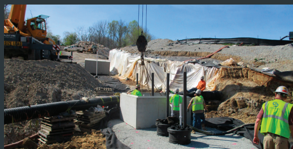
INSTALLING WET WELL #4 CHAMBER BASE
