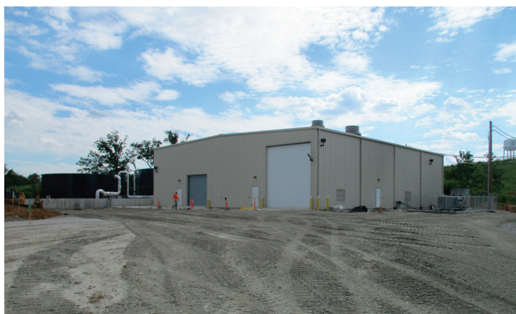
NEW GROUNDWATER TREATMENT PLANT
