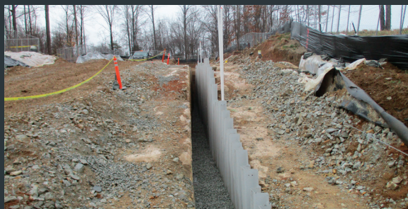
SHEET PILE AND GRAVEL BASE PLACED IN TRENCH
