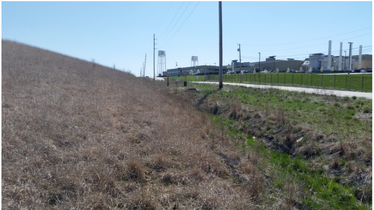
Photo 9: EV1 Vault Cover System, looking South along ES3
