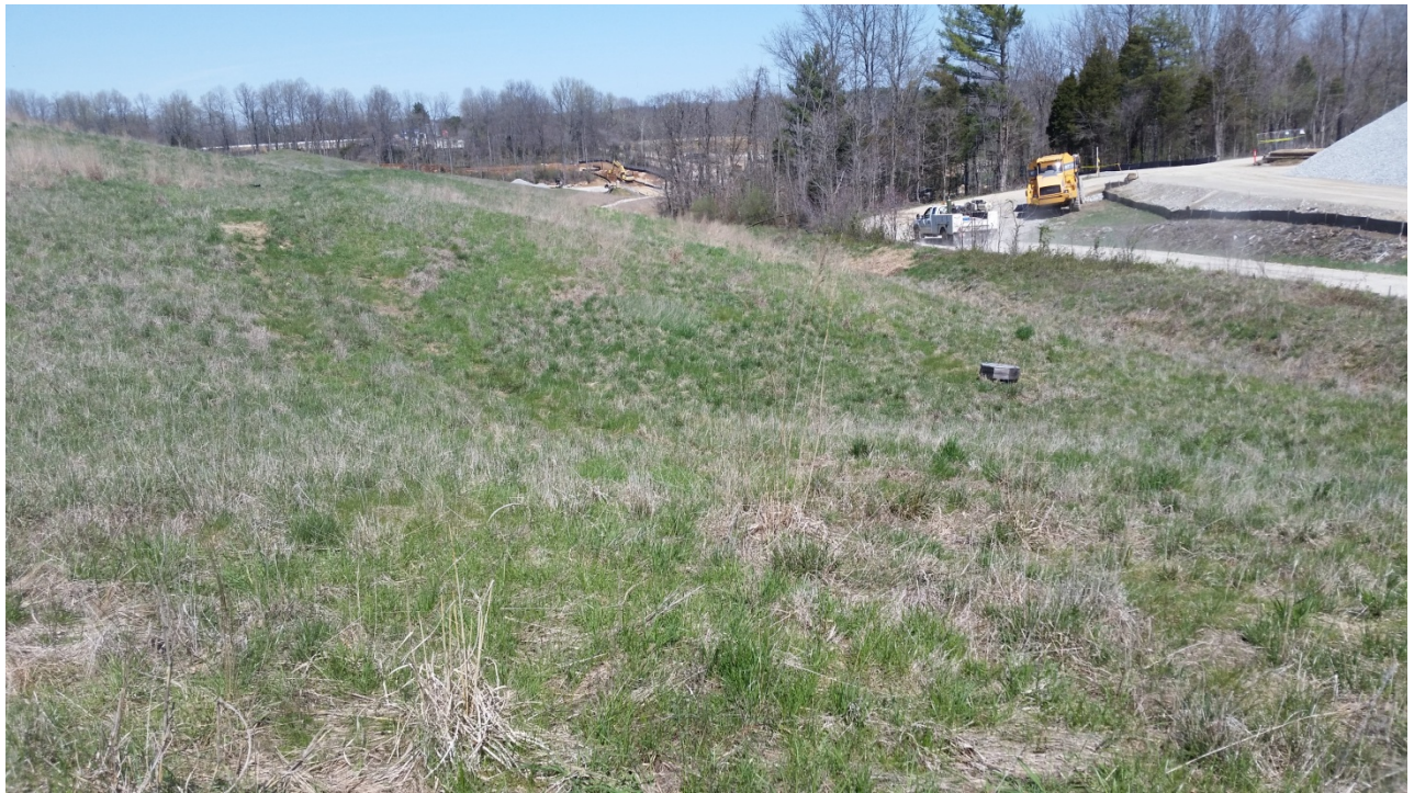
Photo 1: ES6 south of EV5 East Plant Area Cover facing North
