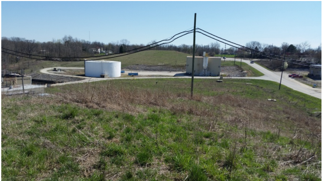
Photo 16: Looking South toward EA2 East Plant Area Cover at EV7
