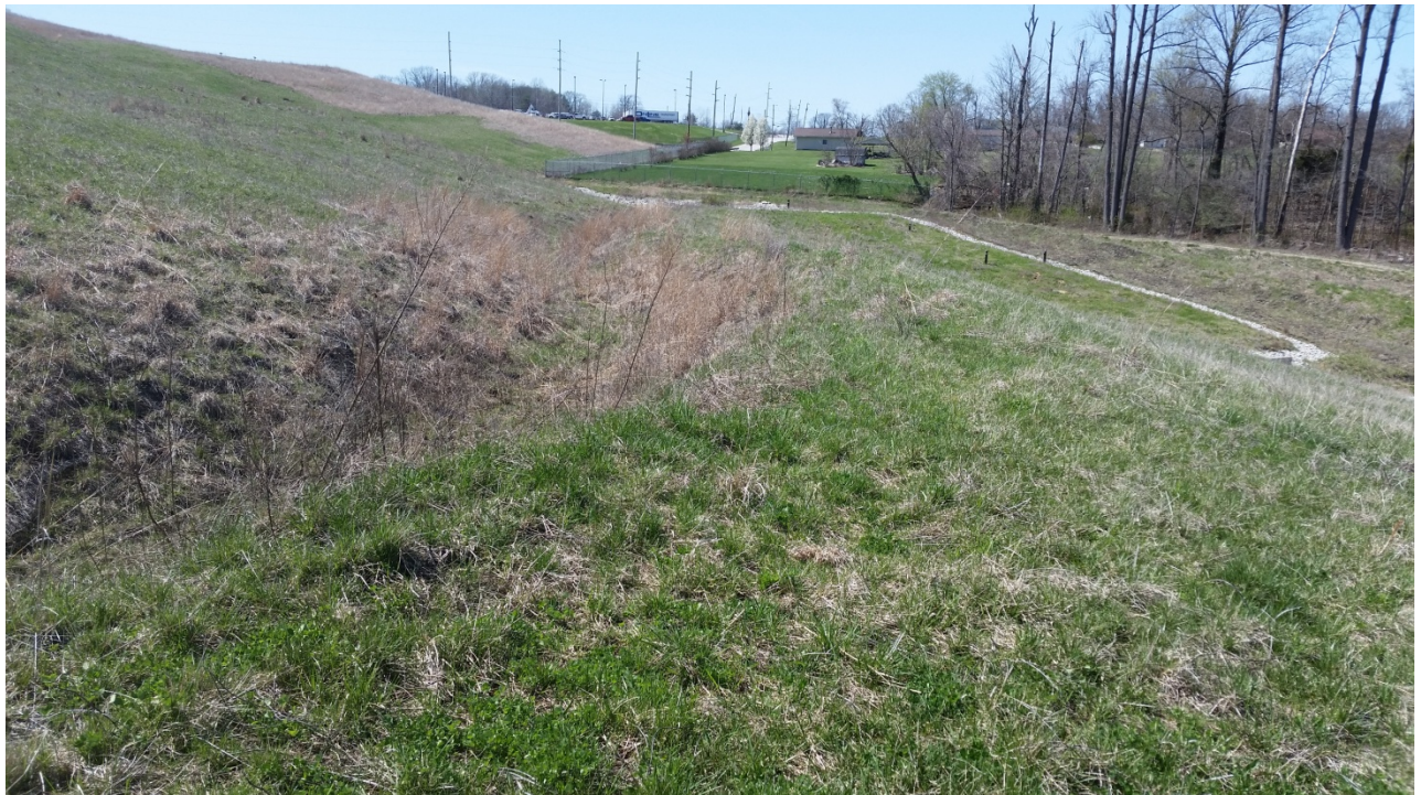
Photo 6: Looking along ES5 East Plant Area Cover facing West
