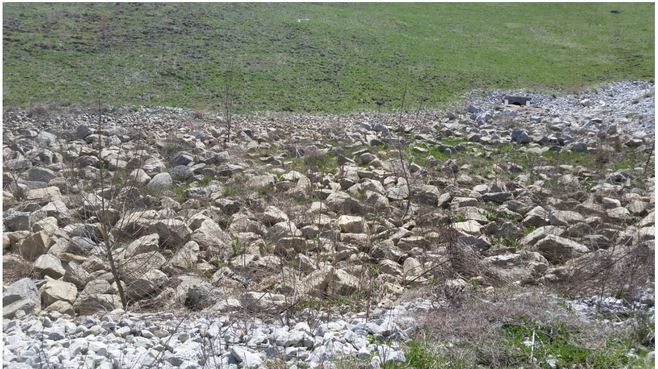
Photo 7: ES6 East Plant Area Cover facing South
