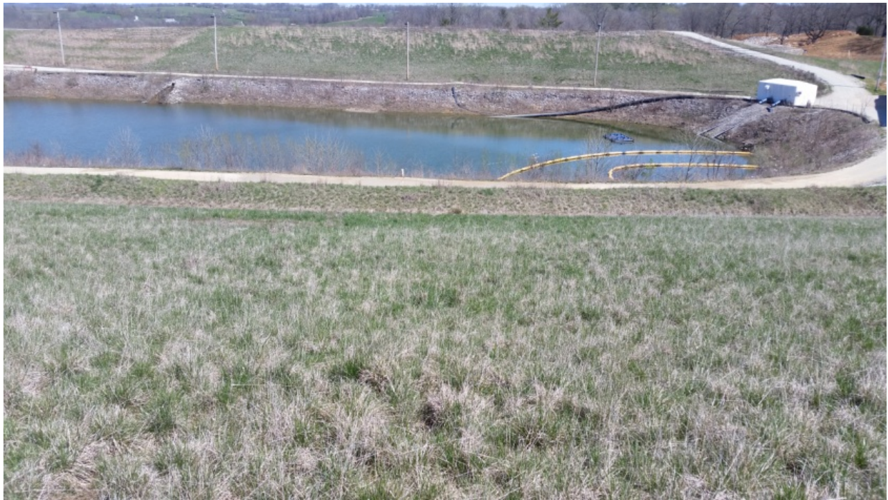
Photo 11: Facing East toward ES1 East Plant Area Cover
