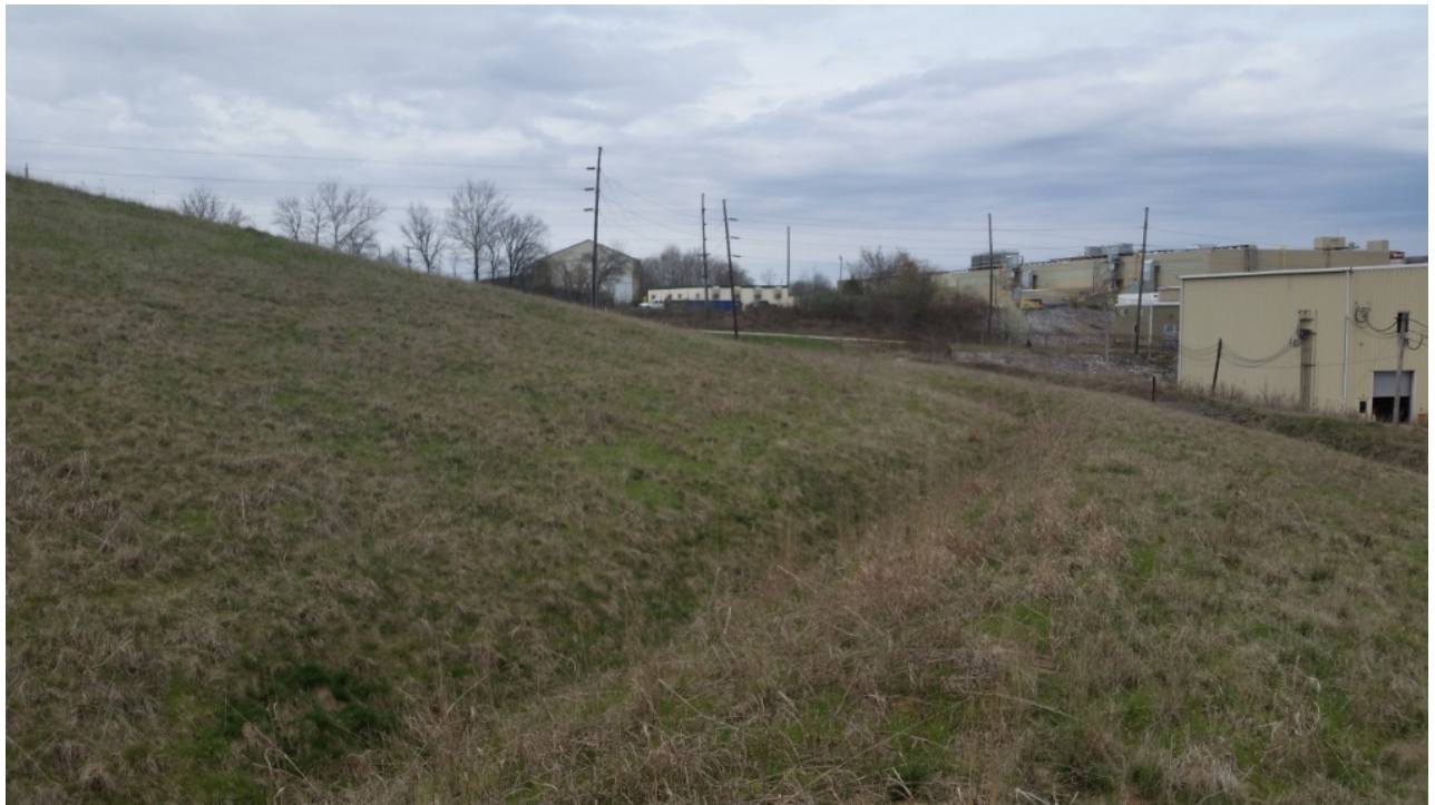
Photo 18: EV9 East Plant Area Cover System at ES14
