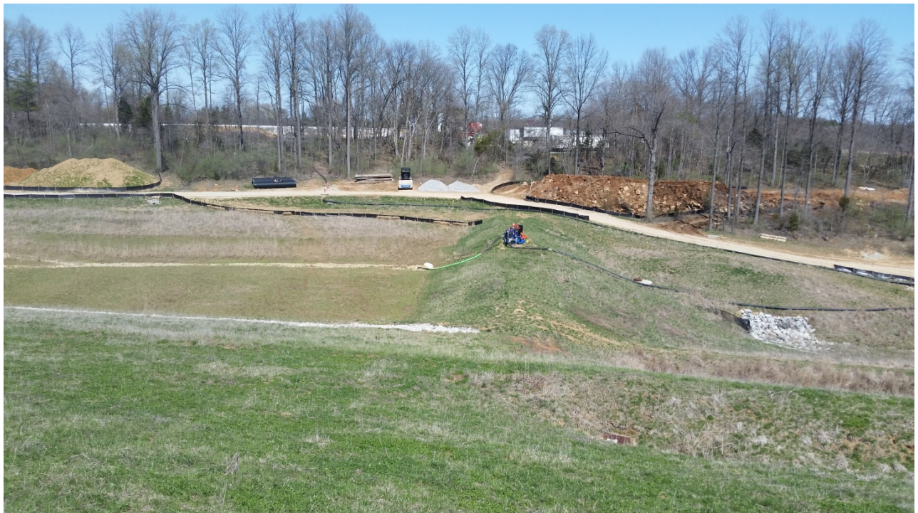
Photo 4: Looking Northeast along EV4 East Plant Area Cover
