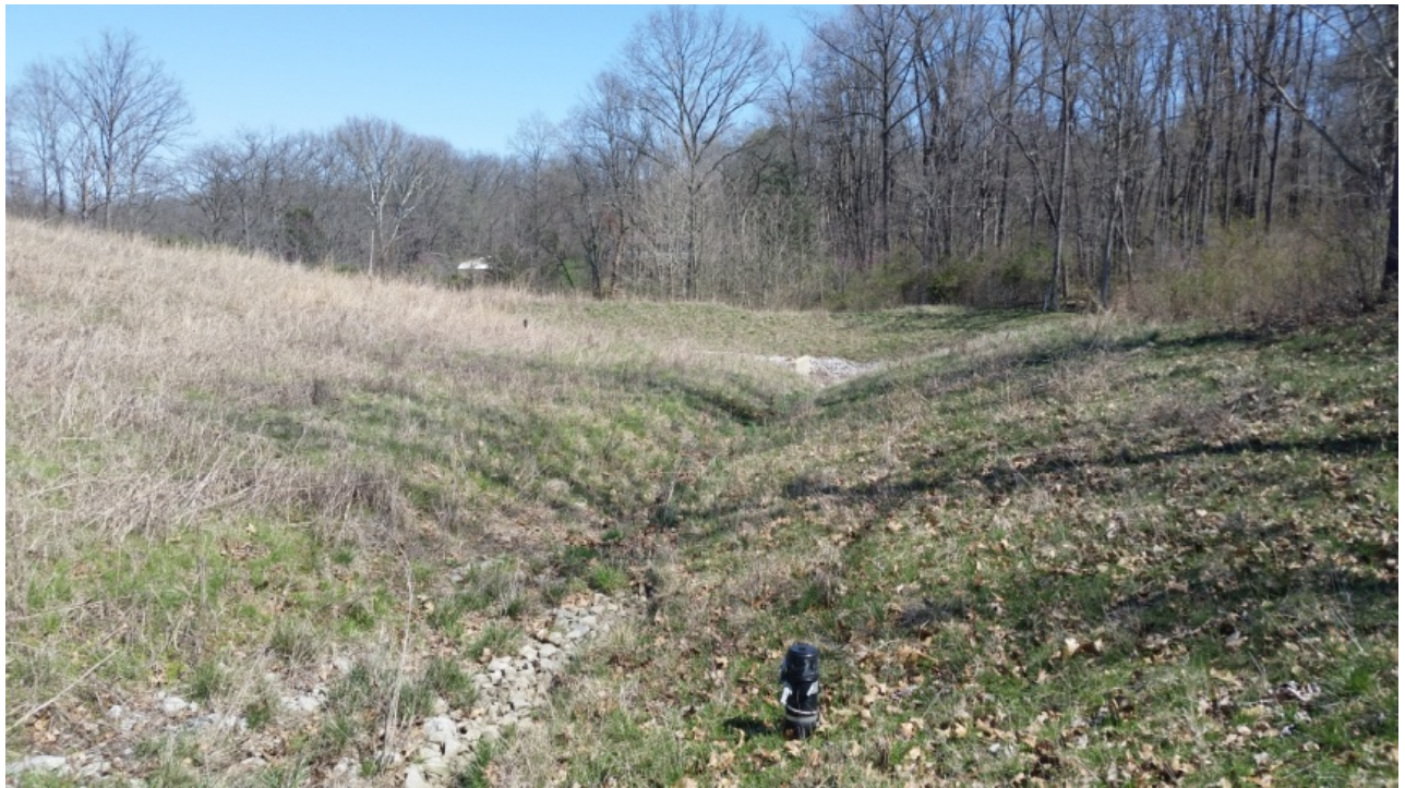
Photo 14: EV8 East Plant Area cover (Parcel 205) facing East
