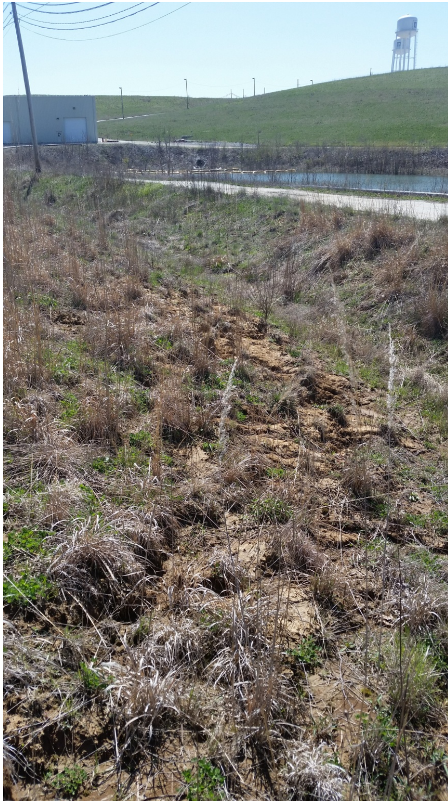
Photo 13: Weed growth and bare spots along ES1 East Plant Area Cover System facing South
