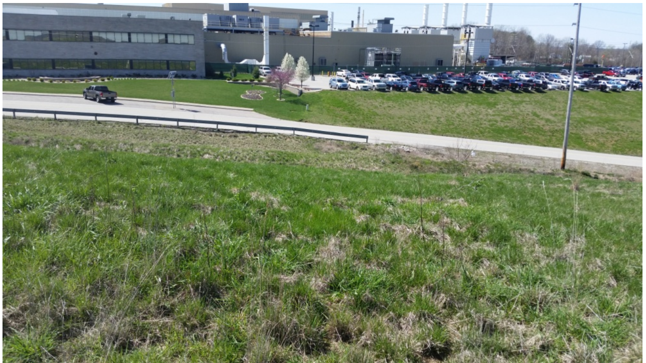
Photo 10: Looking West at WV1 West Plant Area Cover System
