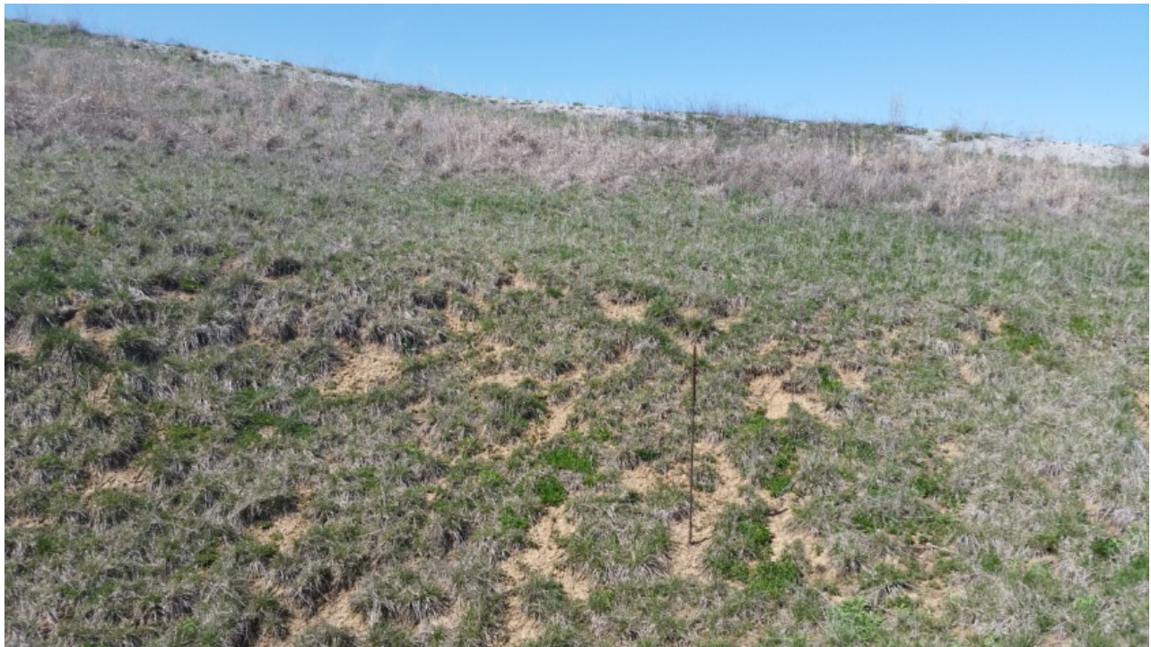
Photo 12: Bare spots near ES2 East Plant Area Cover System facing West
