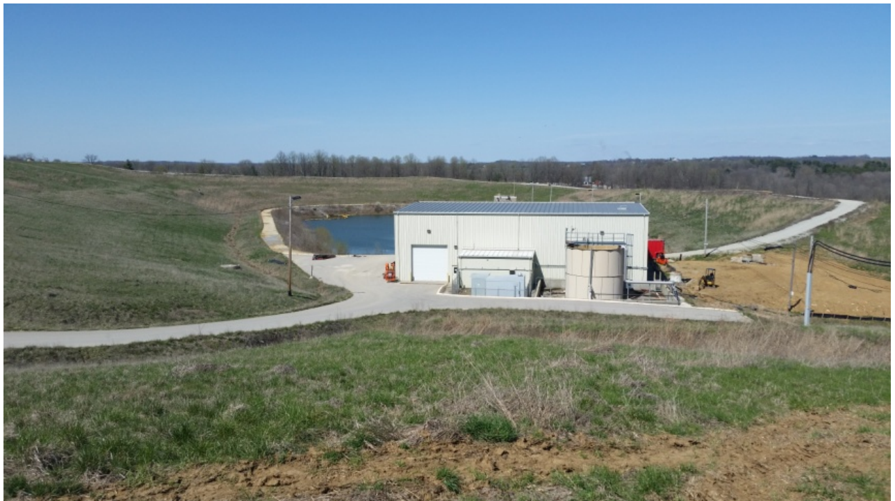
Photo 15: ES12 East Plant Area Cover System looking North
