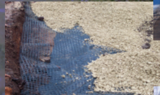
Repairs Performed by Specialized Contractors
