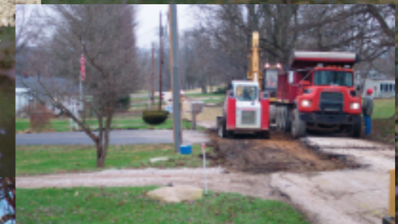
Repairs in Progress
