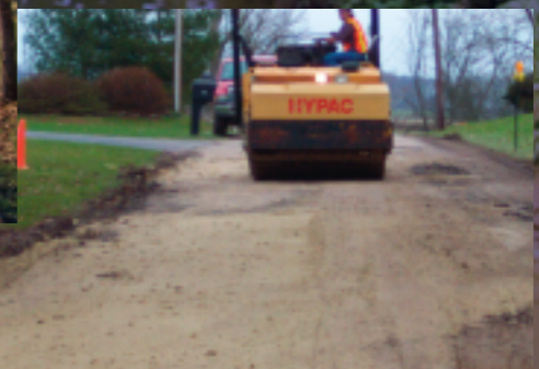
Repairs in Progress
