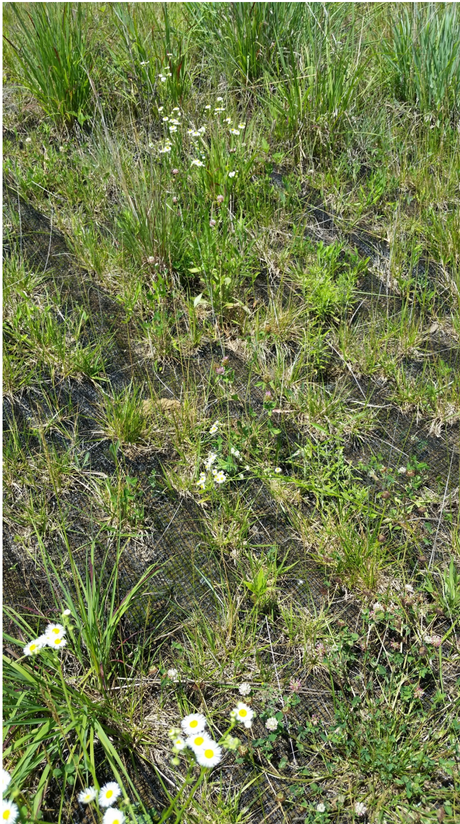
Photo 12: Weed growth and patchy spots along ES1 East Plant Area Cover System facing South.
