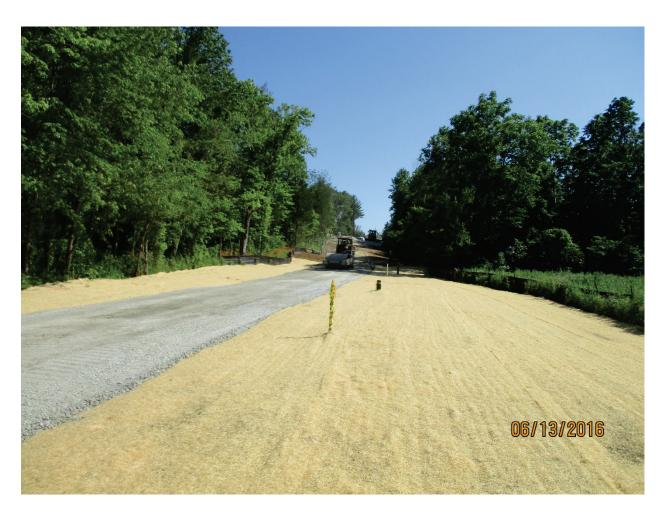
Photo 180: Compaction of #53 stone for WW4 access road. Jun. 2016
