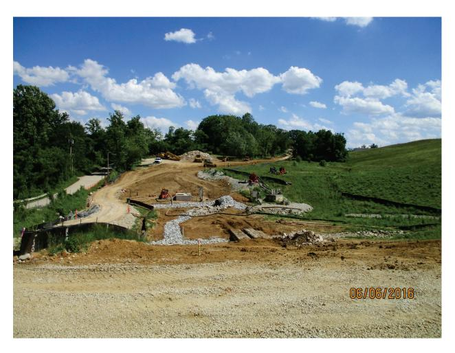
Photo 168: Riprap in low flow channel for DB-4. Jun. 2016
