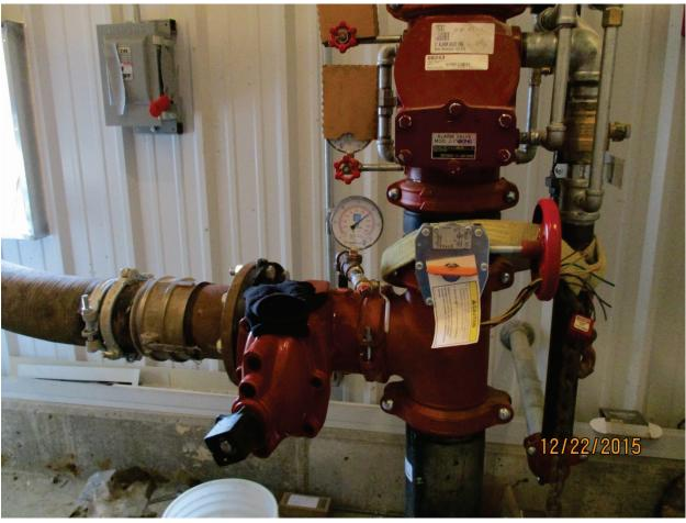
Photo 34: Pressure testing of firemain. Dec. 2015
