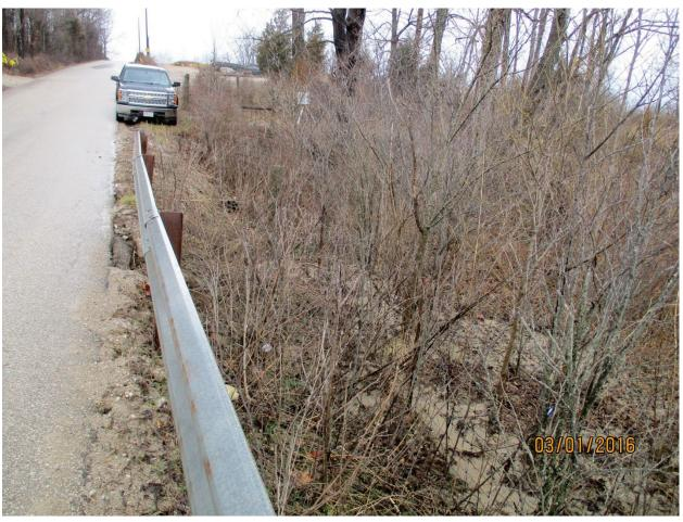
Photo 67: Road erosion at guard rail on east side of Bailey Scales Road. Mar. 2016
