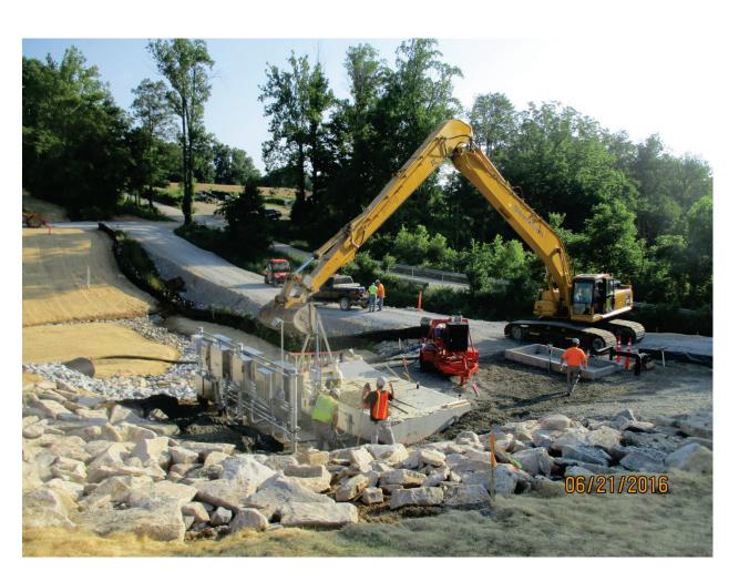
Photo 186: Placing stone for pad around WW4. Jun. 2016
