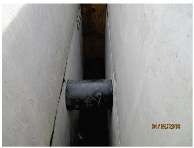
Photo 117: HDPE sleeve between WW chambers. Apr. 2016
