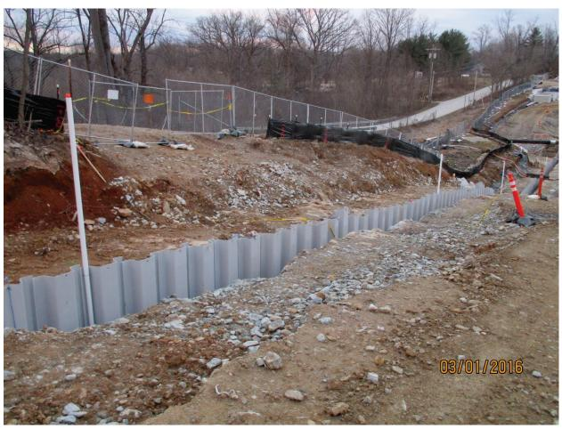
Photo 66: Monitoring wells inside the trench. Mar. 2016
