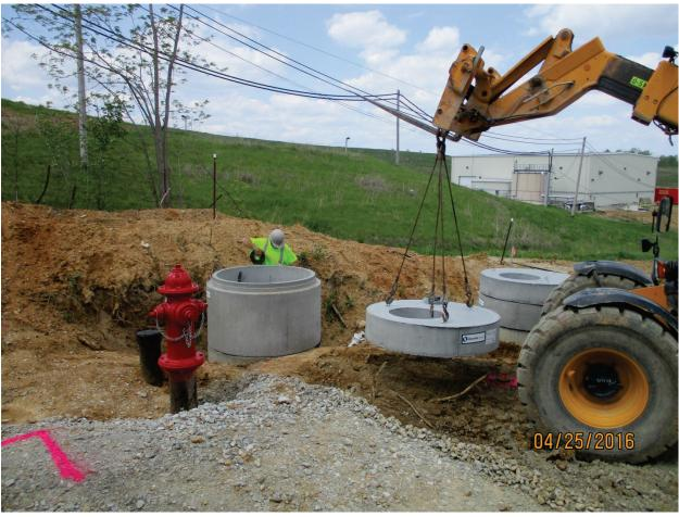
Photo 122: Risers installed on firemain and forcemain MHs. Apr. 2016
