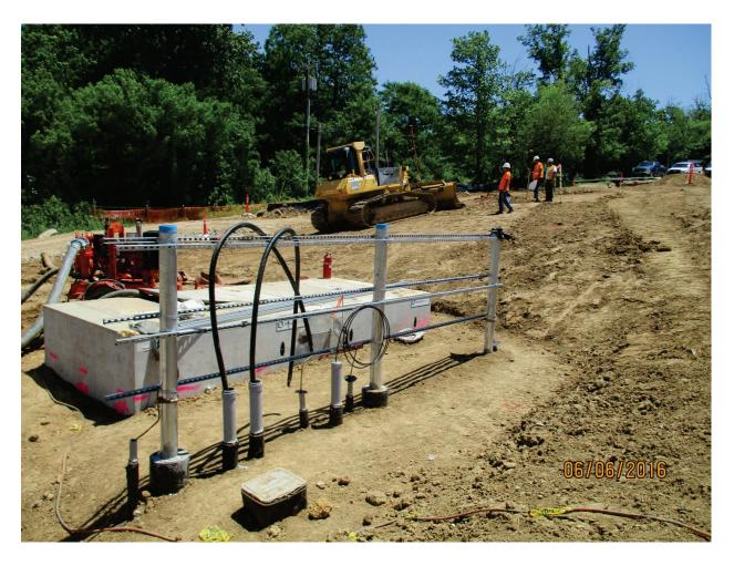
Photo 166: Power cables and fiber optic pulled to WW4 control panel. Jun. 2016
