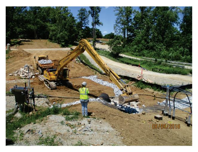
Photo 167: Riprap around DB-5 outfall pipe. Jun. 2016
