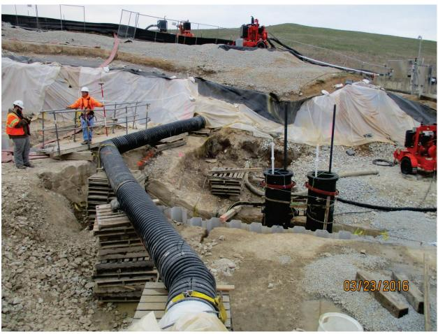
Photo 88: WTP discharge around WW4 chamber. Mar. 2016
