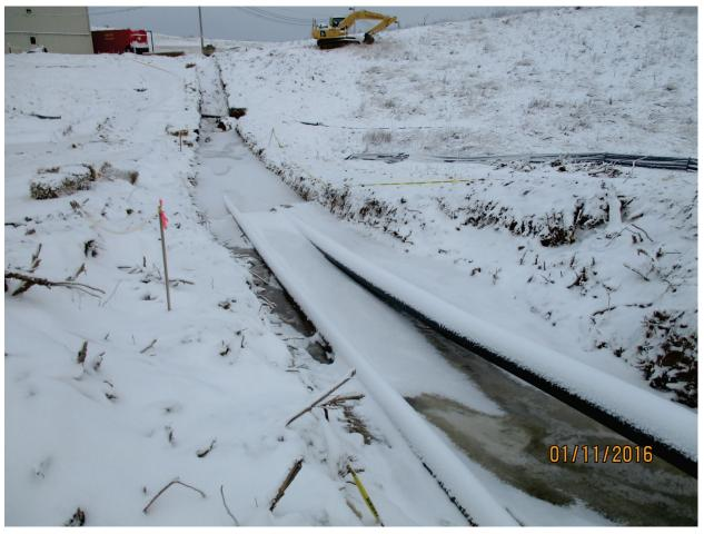
Photo 39: Water in pipe trench. Jan. 2016
