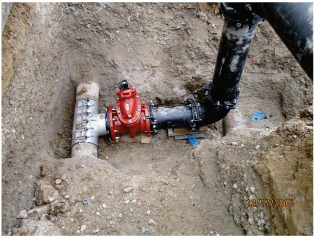
Photo 27: Joint restraints on firemain (deep). Dec. 2015
