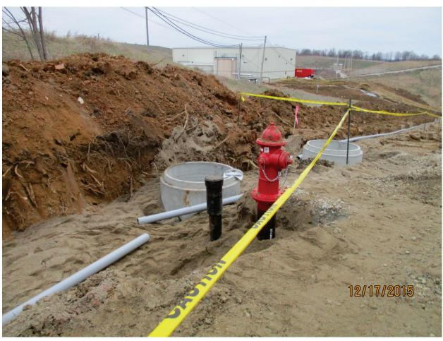
Photo 32: Fire hydrant at new WTP. Dec. 2015
