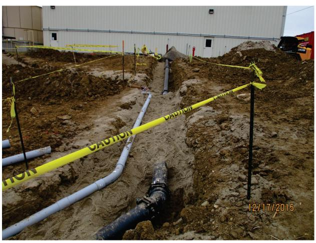
Photo 28: Joint restraints on firemain (shallow). Dec. 2015
