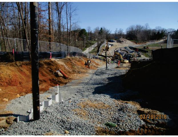
Photo 87: Stone backfill in north trench section. Mar. 2016
