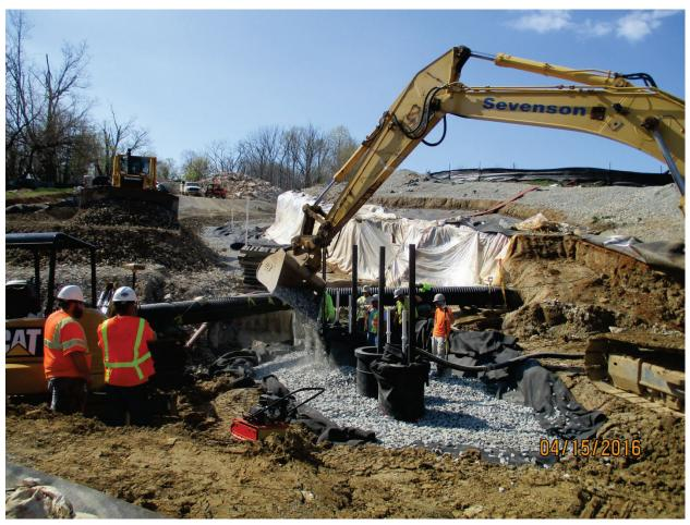
Photo 111: Backfilling around sumps with 2-inch stone. Apr. 2016
