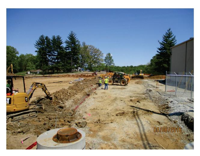
Photo 136: Backfilling conduit trench to pull box. May. 2016
