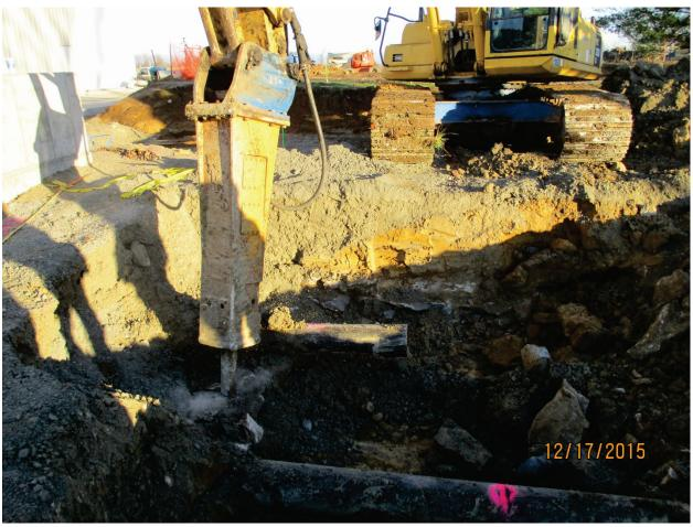
Photo 30: Concrete breaking at MH-10 and MH-14. Dec. 2015
