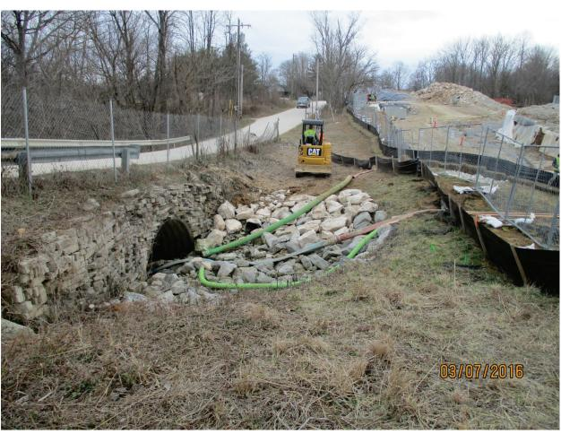
Photo 74: Riprap at discharge under Bailey Scales Road. Mar. 2016
