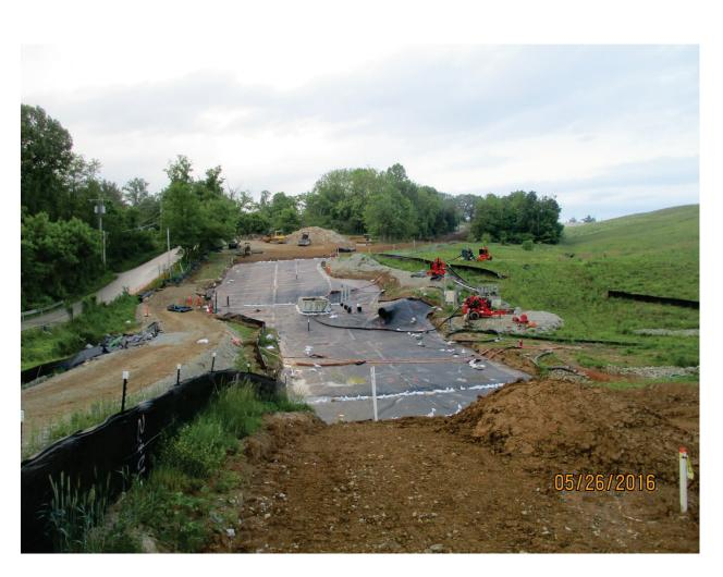
Photo 155: Liner placement over trench area. May. 2016
