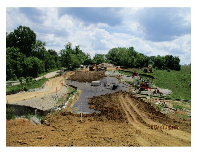
Photo 160: Placing common fill over liner. May. 2016
