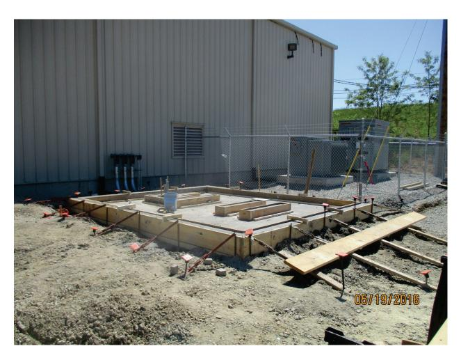
Photo 153: Concrete pour for containment around generator pad at GWTP. May. 2016
