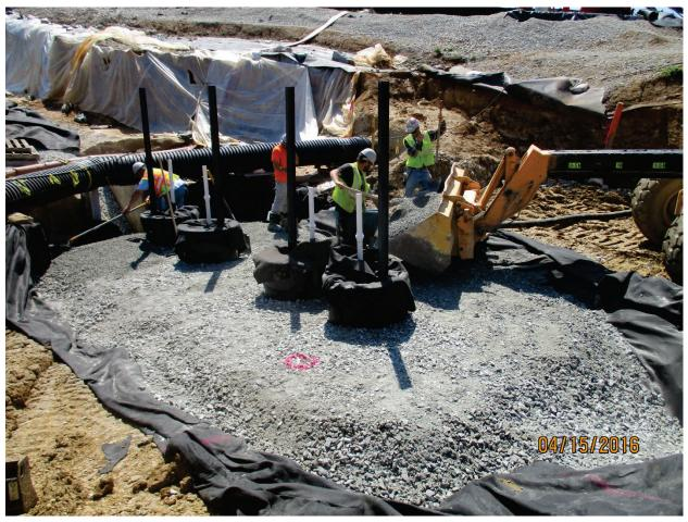
Photo 112: Levelling subgrade with #11 stone and filter fabric at WW sumps. Apr. 2016
