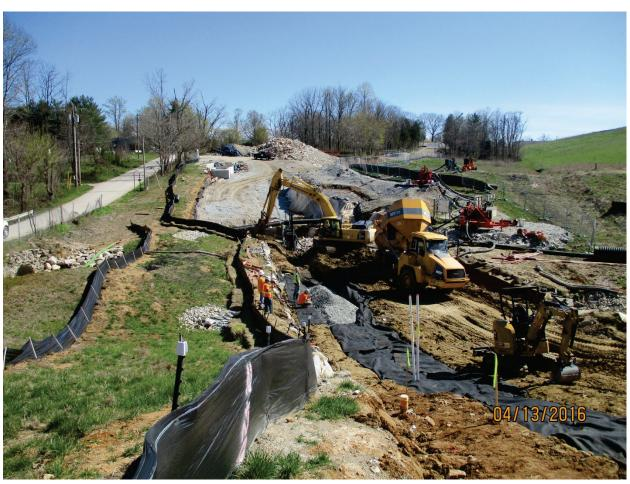
Photo 110: Covering of filtration media at working platform. Apr. 2016
