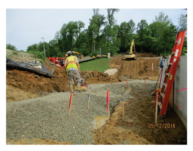
Photo 143: Compacting stone over outfall pipe. May. 2016
