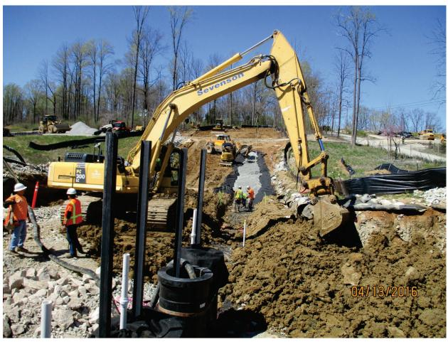
Photo 109: Placement of filtration media at working platform. Apr. 2016
