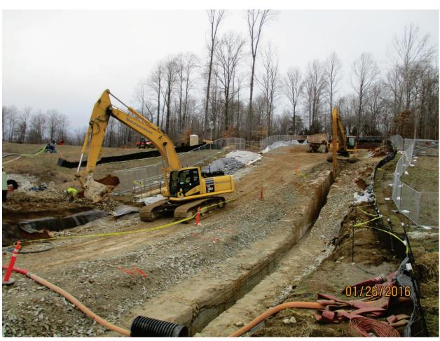
Photo 47: Trench cleanout for vinyl sheet installation. Jan. 2016
