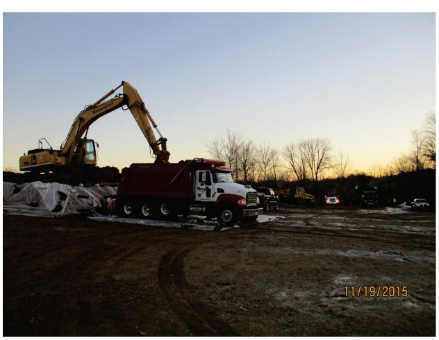
Photo 9: Loading contaminated soil. Nov. 2015
