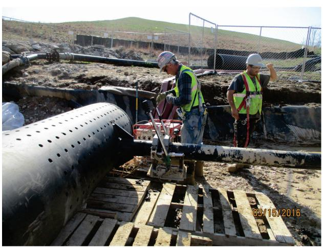
Photo 83: Welding perforated pipe to WW sump. Mar. 2016
