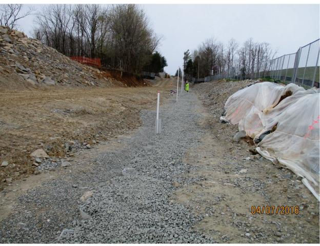
Photo 105: Stone placed in south trench. Apr. 2016
