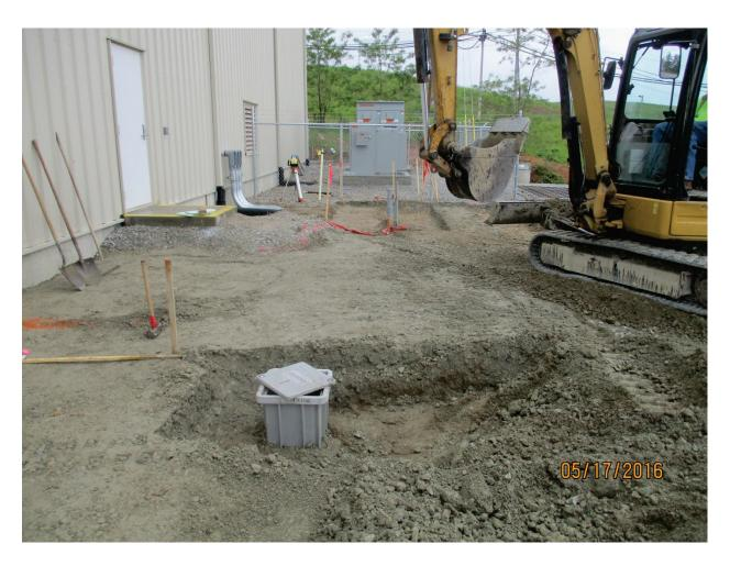
Photo 149: Grounding inspection well by generator. May. 2016
