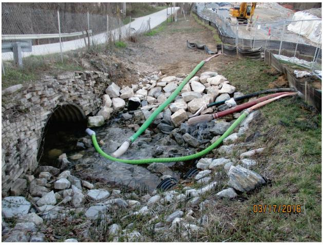
Photo 86: Stormwater discharge from DBs (filter socks on discharge). Mar. 2016
