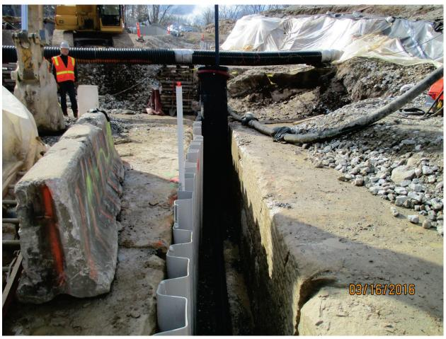
Photo 84: Sump and perforated pipe in north trench. Mar. 2016
