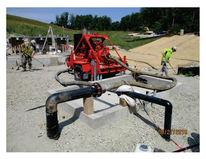
Photo 187: Hooking up backup pump near WW4. Jun. 2016
