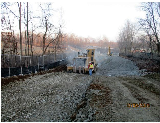
Photo 22: Extended working platform. Dec. 2015
