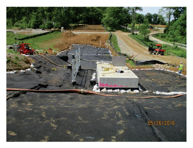
Photo 157: Geocomposite and filter fabric over liner. May. 2016
