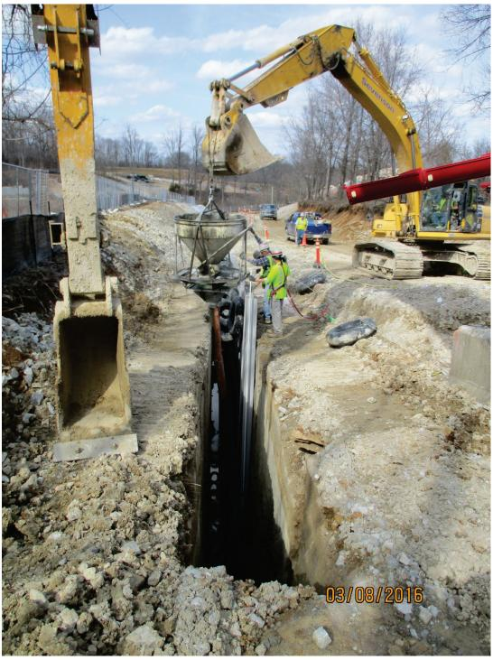
Photo 77: Completion of grout placement. Mar. 2016
