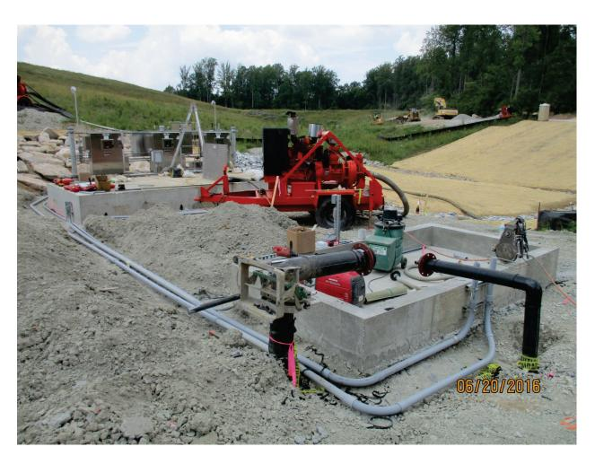
Photo 185: Conduits between WW4 and diesel pump pad. Jun. 2016
