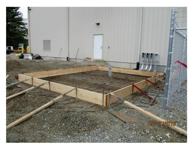
Photo 150: Forming rebar mat for generator pad. May. 2016
