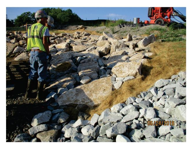
Photo 189: Re-enforcing rock barrier with riprap. Jun. 2016.
