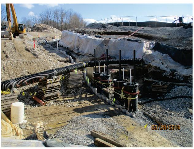
Photo 92: Sump pipes set into trench, surrounded by 2-inch stone. Mar. 2016
