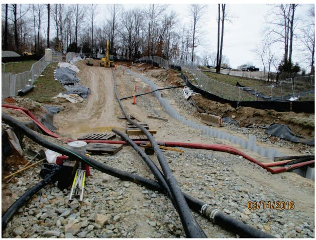
Photo 81: Welded perforated pipe. Mar. 2016
