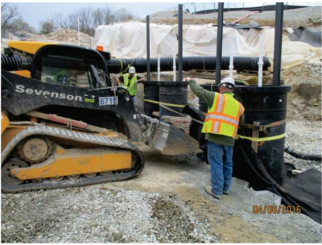
Photo 104: Backfill behind sheets at sump area. Apr. 2016
