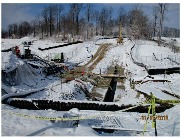
Photo 40: Trench cleared for sheet piling. Jan. 2016
