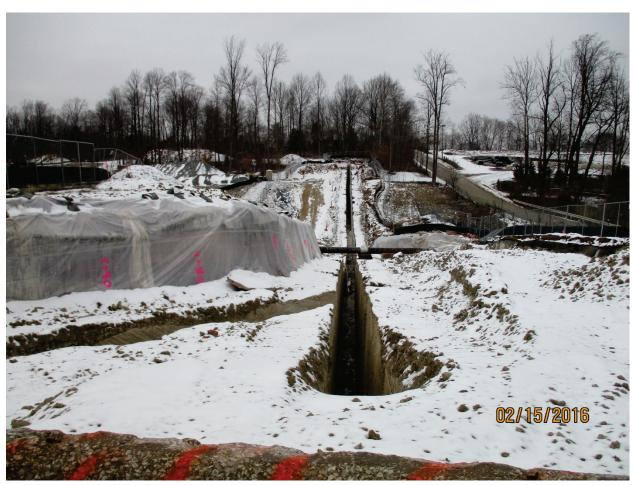
Photo 51: Buildup of fines at trench bottom. Feb. 2016
