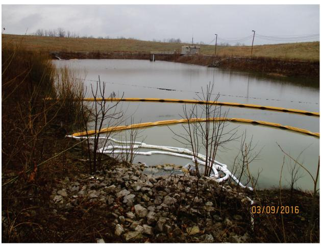
Photo 80: Absorbent boom at SW outfall to SW pond. Mar. 2016
