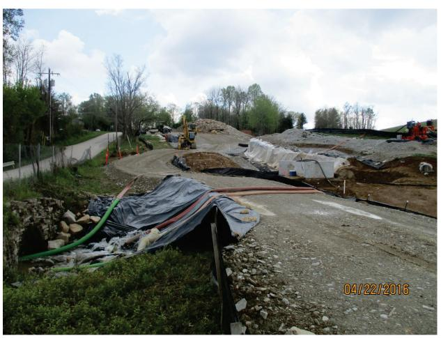
Photo 121: Pumping DB-2 water through bag filters. Apr. 2016
