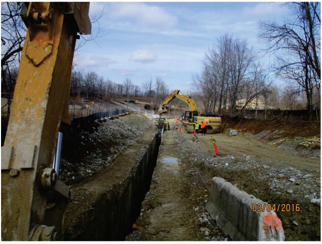
Photo 72: Grout placement using concrete bucket. Mar. 2016
