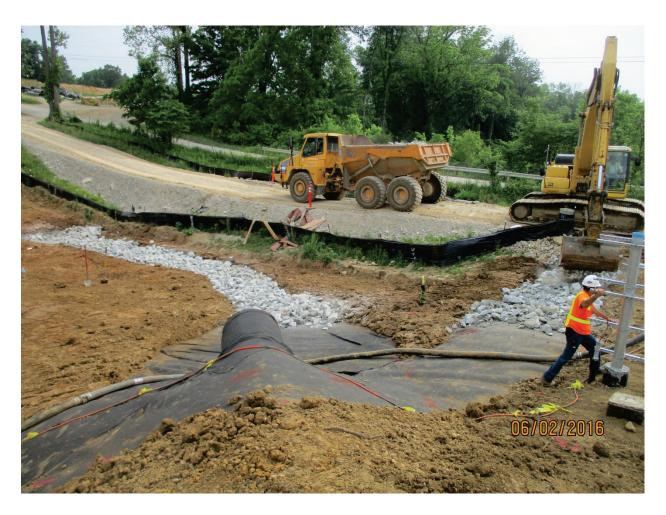
Photo 164: Placing stone in DB-4 low flow channels. Jun. 2016
