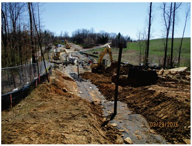
Photo 94: Clay backfill over north trench. Mar. 2016
