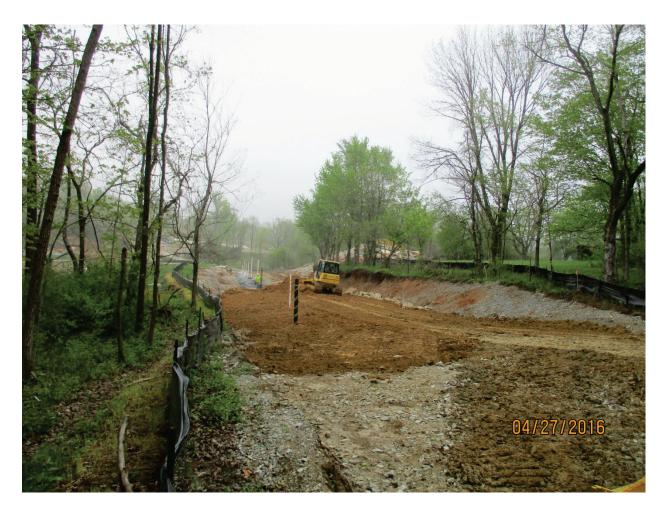
Photo 127: Clay from GWTP placed over south trench. Apr. 2016
