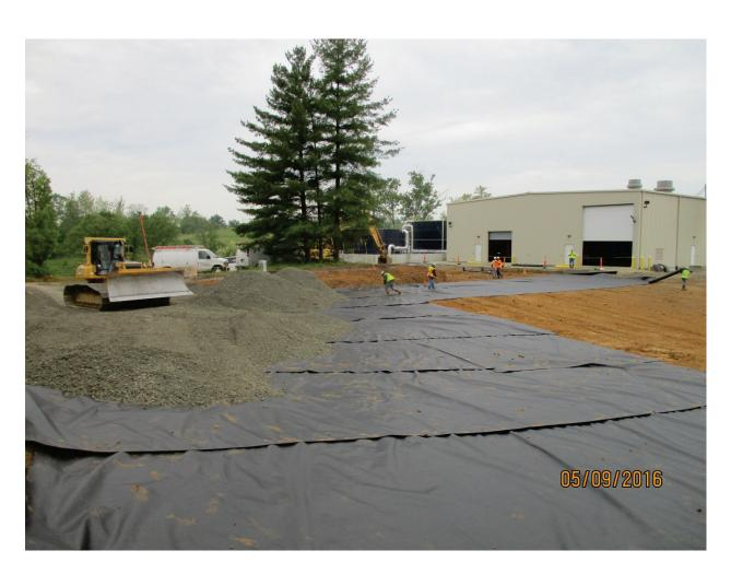
Photo 139: First lift of stone on drive area. May. 2016
