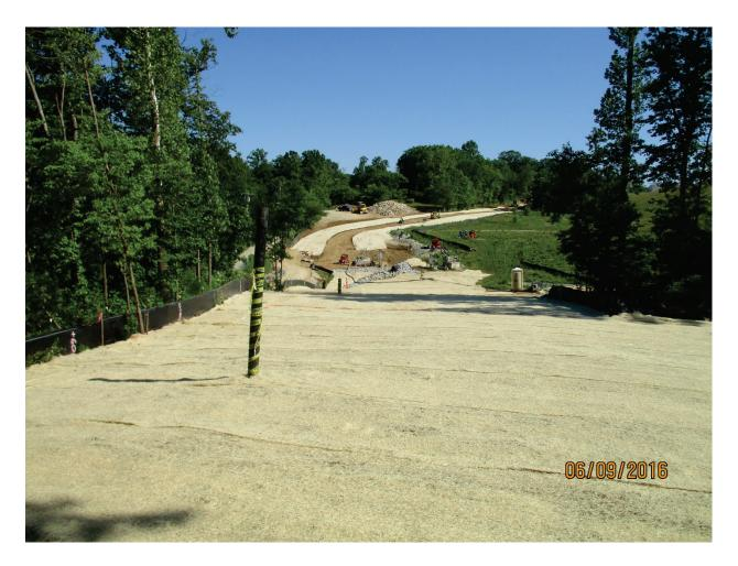
Photo 176: Seeding and erosion control mat over trench. Jun. 2016
