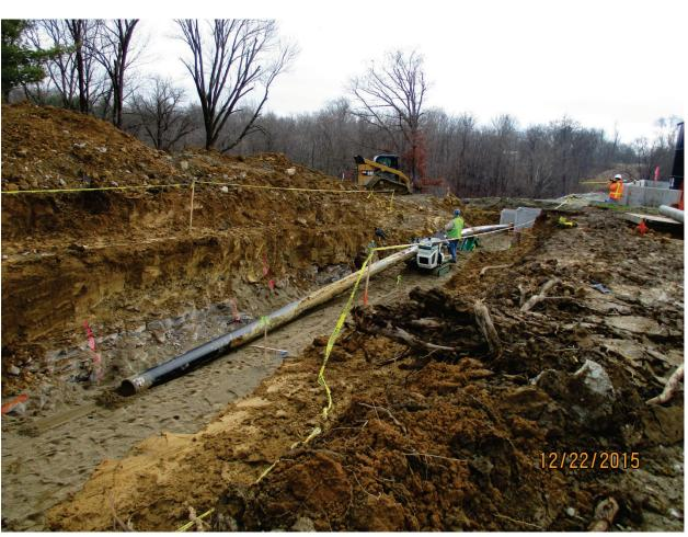
Photo 35: Laying pipe in trench. Dec. 2015
