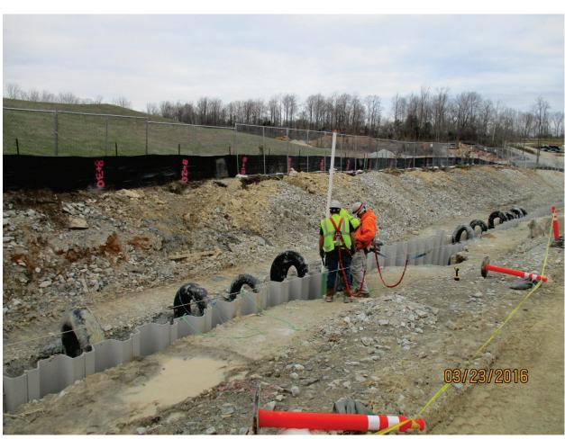
Photo 89: Piezometers in south trench. Mar. 2016
