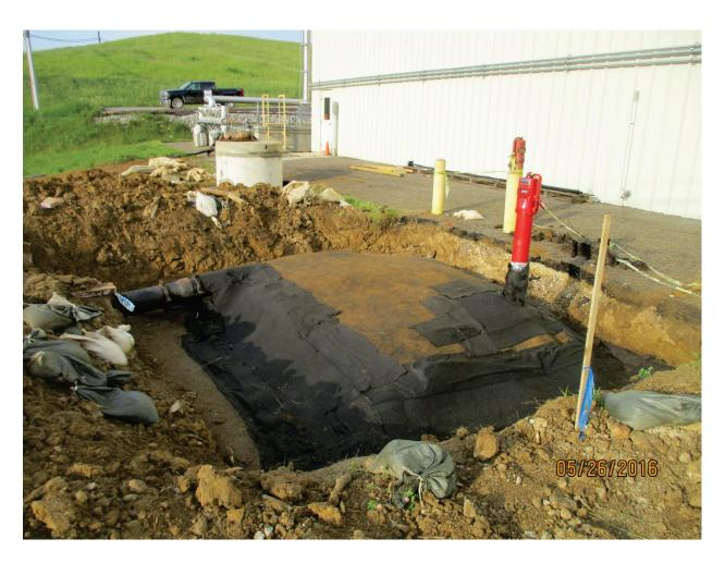
Photo 156: Liner repair at firemain and PIV. May. 2016
