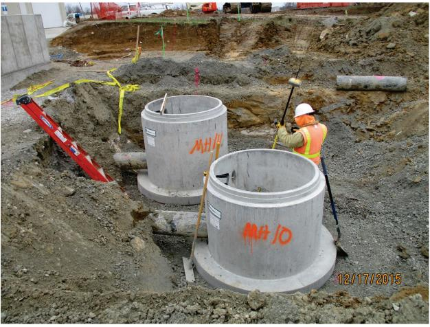
Photo 31: Manhole placement at MH-10 and MH-14. Dec. 2015
