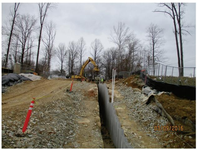
Photo 78: Stone placement in base of trench. Mar. 2016
