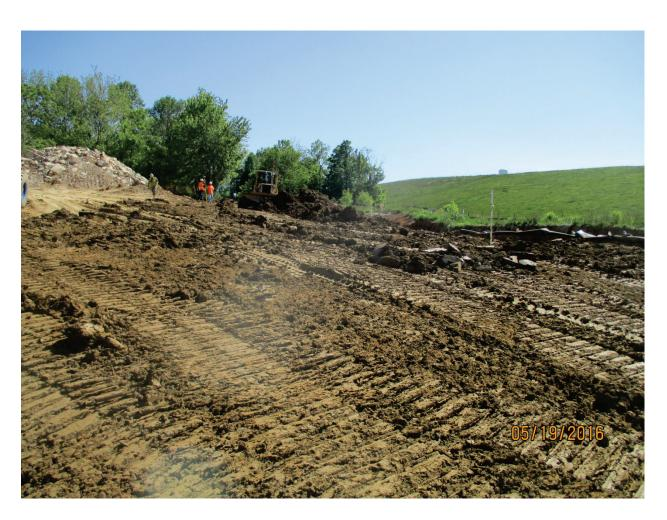
Photo 154: Grading clay over south trench area. May. 2016
