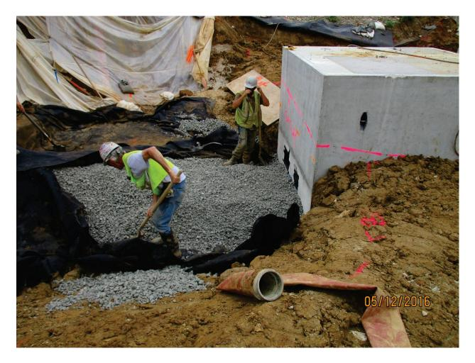
Photo 144: Infiltration media south of WW4 chamber. May. 2016
