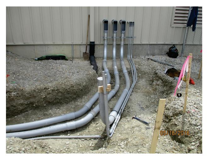
Photo 146: Conduits run for WW4 cables and generator. May. 2016
