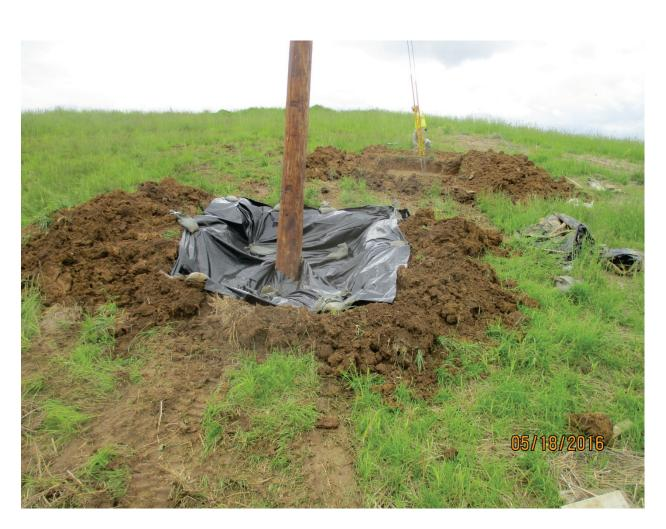
Photo 151: Preparing for liner repair around power poles. May. 2016
