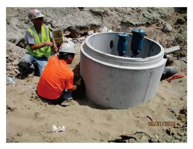
Photo 161: Grout sealing of MH-16. May. 2016
