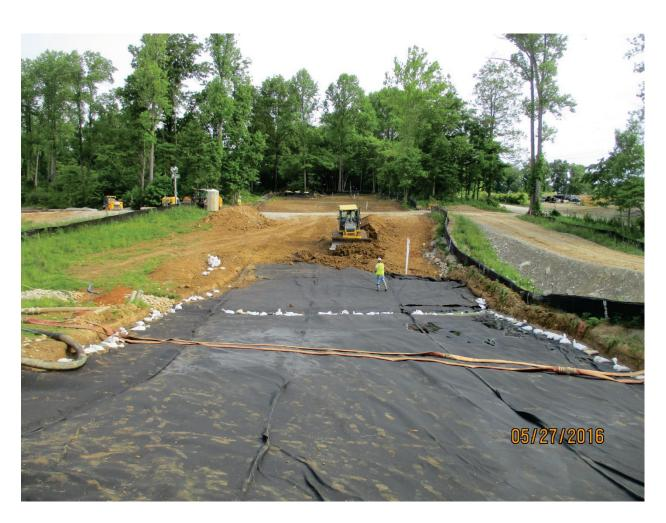
Photo 159: Backfilling anchor trench at north end. May. 2016
