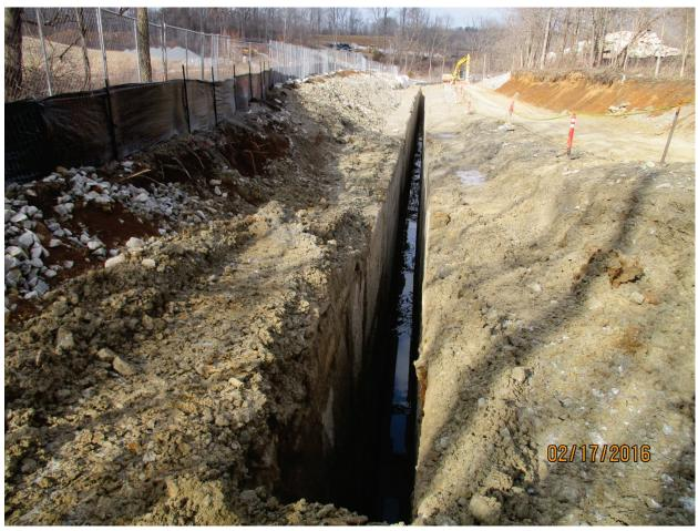
Photo 55: South trench with cuttings removed. Feb. 2016
