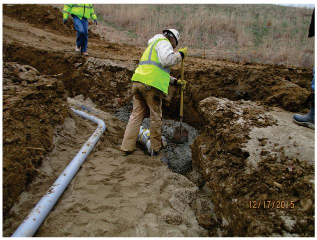
Photo 29: Thrust block for firemain. Dec. 2015
