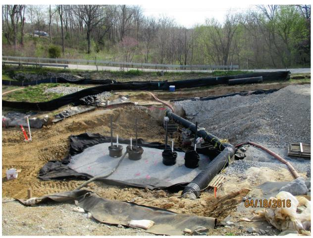
Photo 113: Compacting subgrade around WW4 sumps. Apr. 2016
