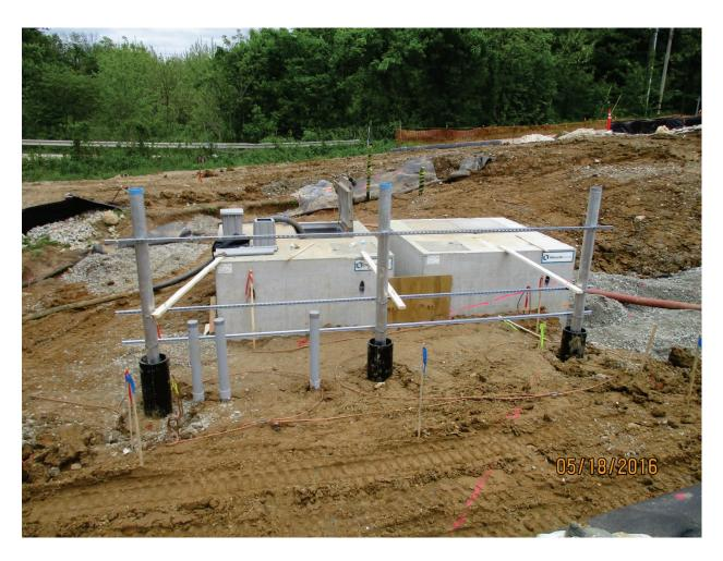
Photo 152: Posts for electrical panel at WW4. May. 2016
