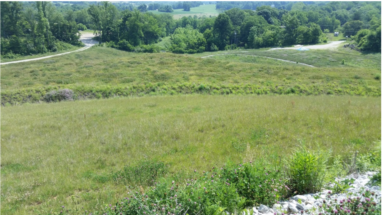
Photo 6: EV4 East Plant Area cover facing northeast
