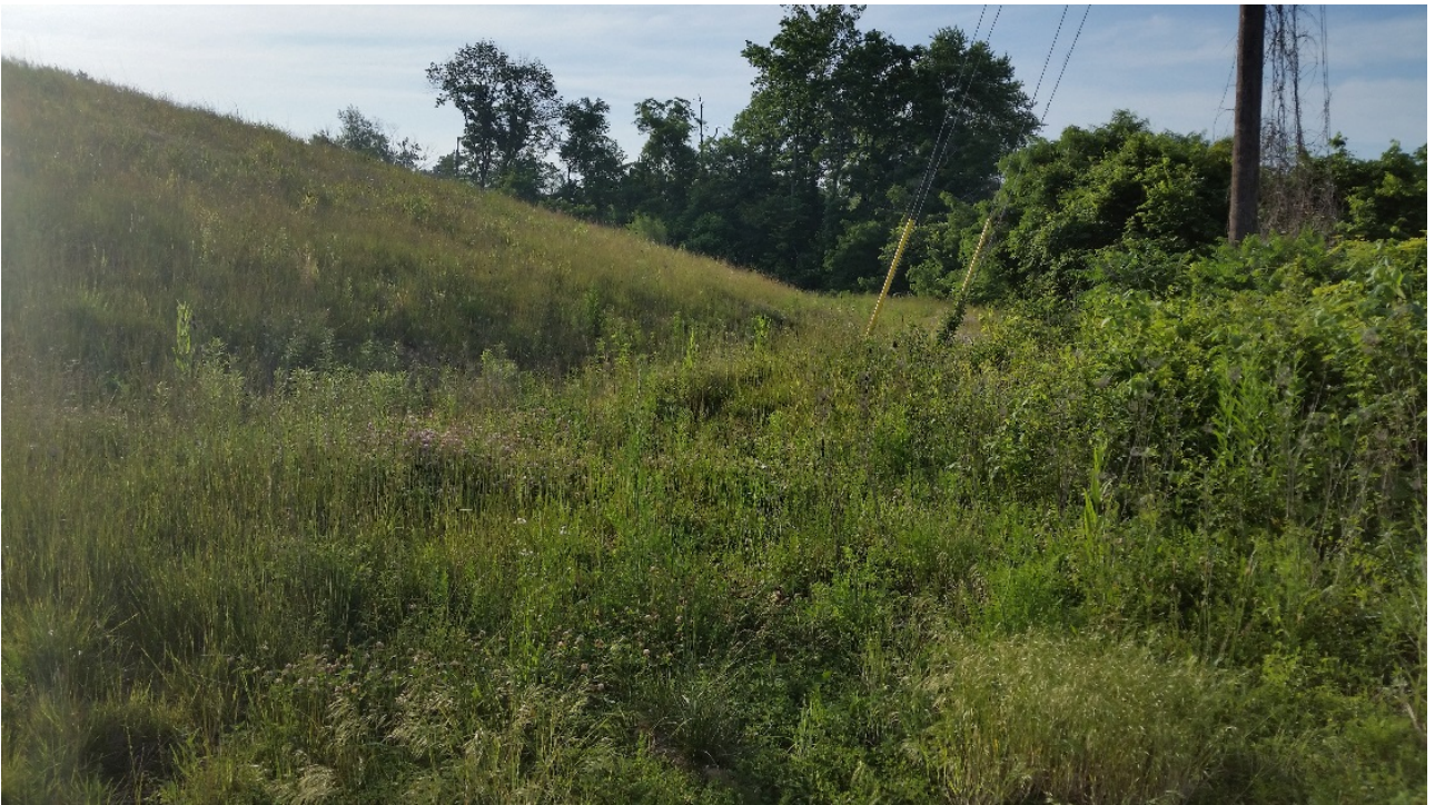
Photo 13: EV9 East Plant Area cover facing east (at base of slope)
