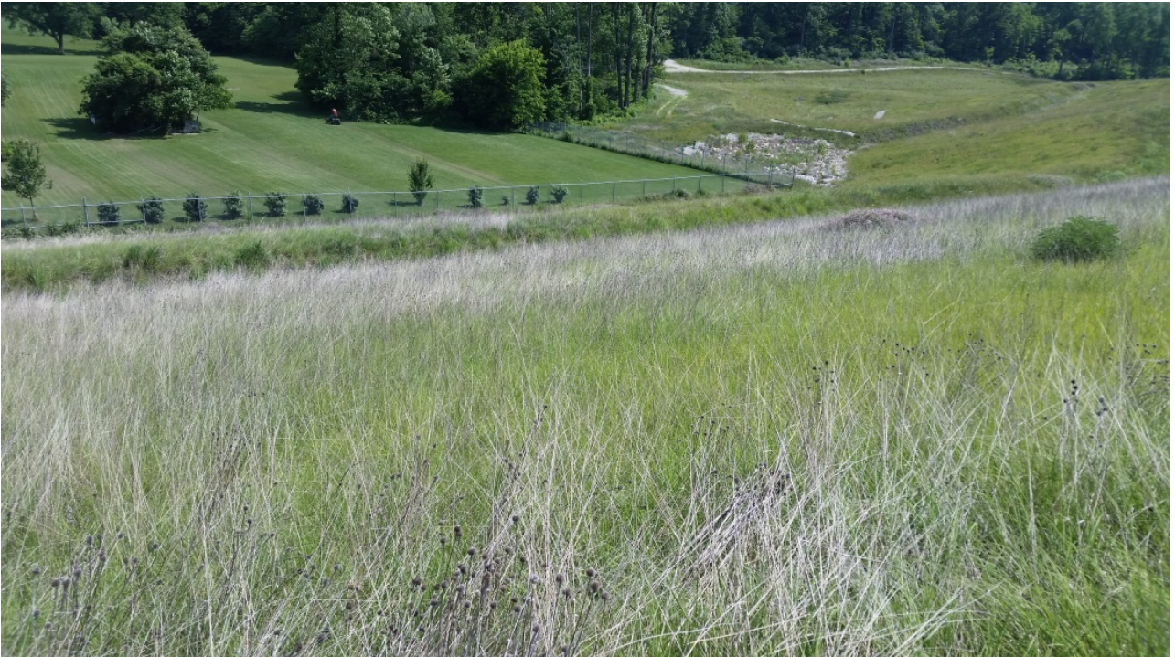
Photo 19: ES5 drainage swale facing northeast
