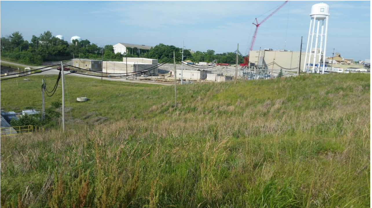
Photo 10: EV6 East Plant Area cover facing southwest
