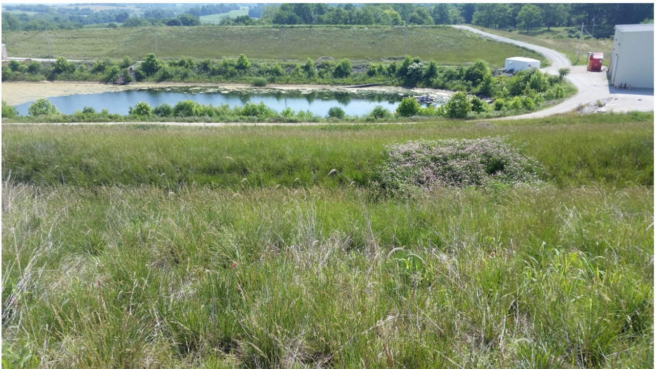
Photo 2: EV1 Vault cover (and East Plant Area cover beyond) facing east
