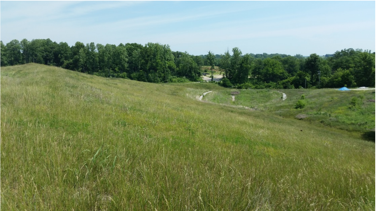
Photo 23: ES11 detention basin #5 facing north
