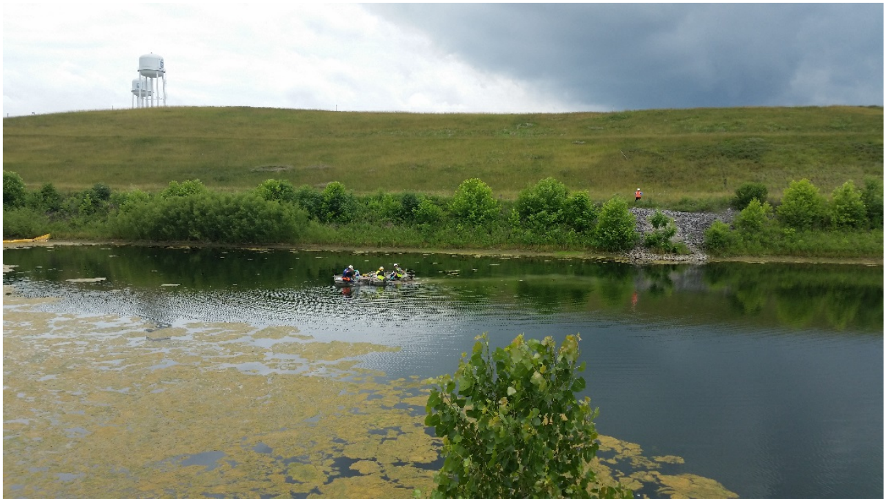
Photo 27: Phoslock Application in the stormwater pond facing southwest
