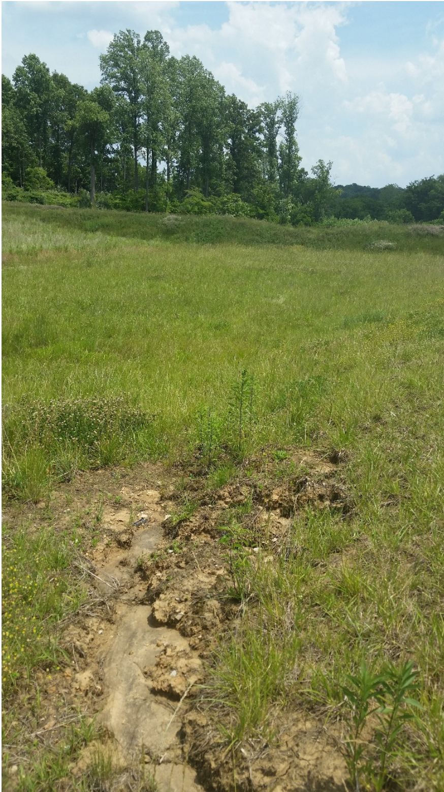
Photo 22: ES10 channel through detention basin #3 facing east
