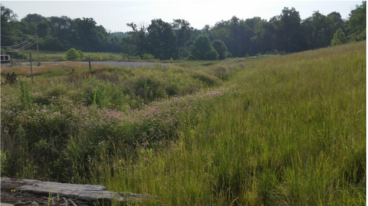
Photo 14: ES14 East Plant Area cover facing northwest
