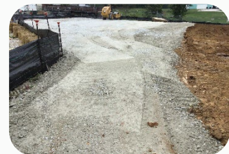
Parking Area Repair
